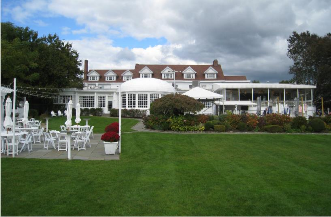
Fig. 4. Rear view of The Inn at Longshore, Existing Conditions
