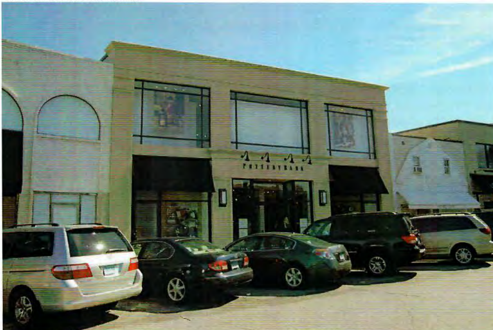
View of the west elevation.
