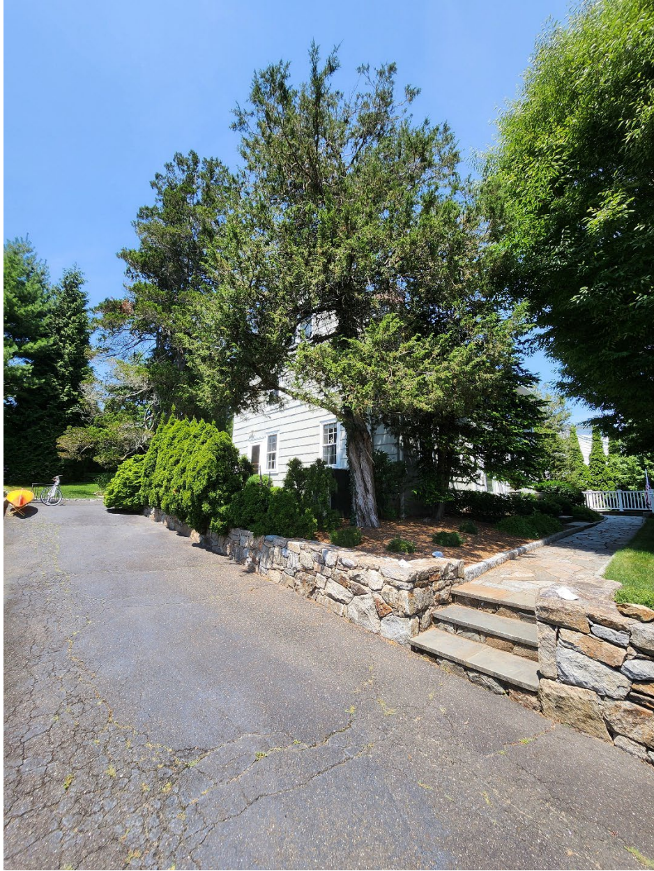
Southern elevation, view northwest
