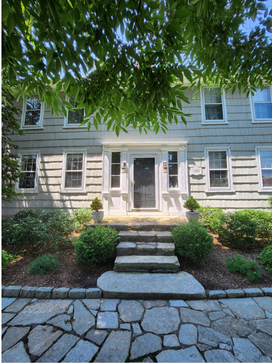
Detail of front door and eastern facade, view west
