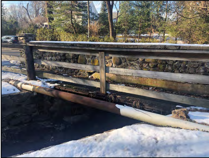
Figure 9 - Long Lots Road - View of South Parapet Wall Looking NW
