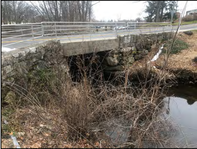
Figure 3: Jesup Road Bridge North Side Looking SW
