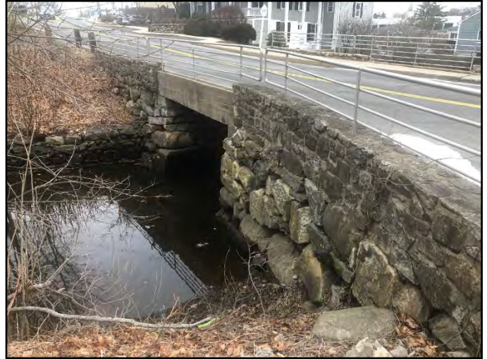
Figure 4: Jesup Road Bridge South Side Looking NW
