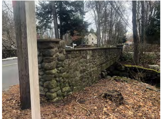
Figure 2: Evergreen Avenue Bridge - North Parapet Wall Looking SW
