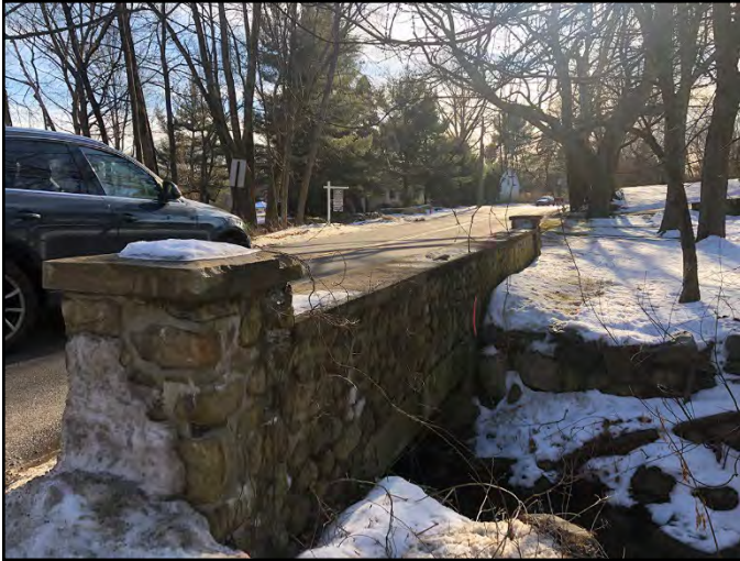
Figure 7: Cross Highway Bridge - View of North Parapet Wall Looking SW
