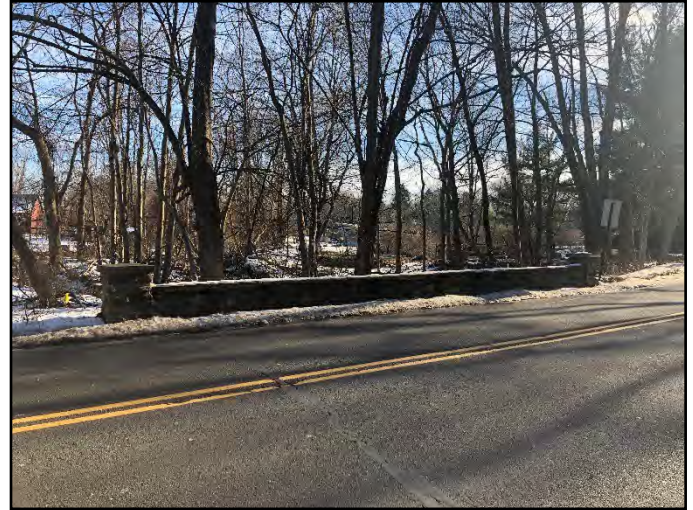
Figure 8: Cross Highway Bridge - View of South Parapet Wall Looking SW
