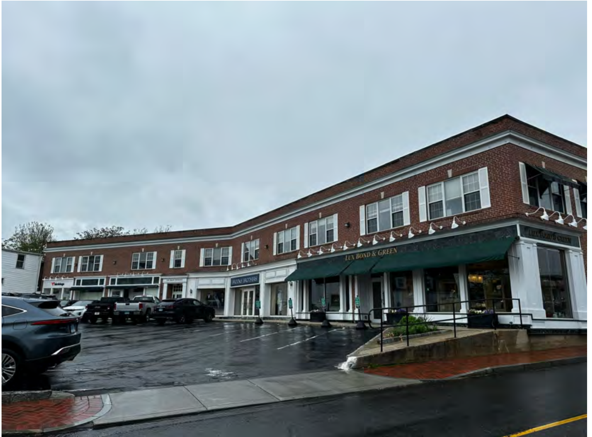
Existing full-front elevation, from across Elm Street (better view than Main)
