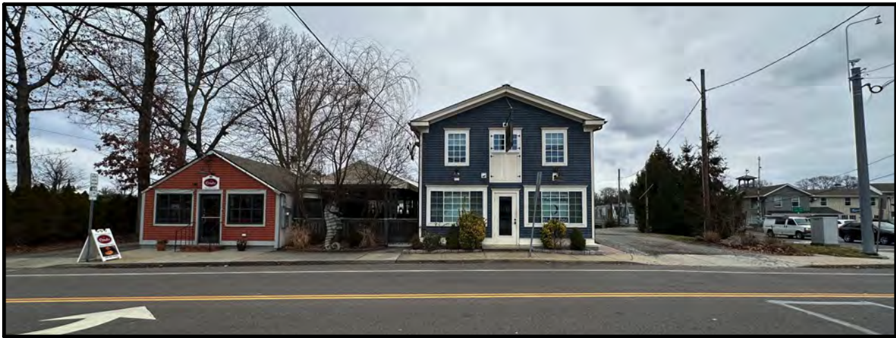
2 RIVERSIDE AVE FACADE AND ADJACENT BUILDING
