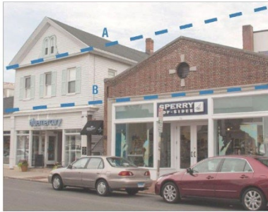
A: Similar Cornice Line and Roof Peak B: Similar Cornice Lines
