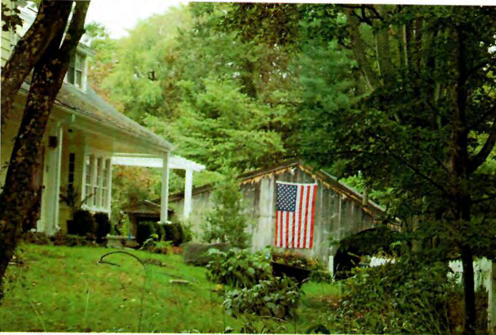
View of the south elevation of the barn.
