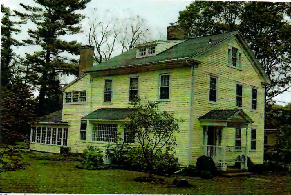
View of the west and south elevations.
