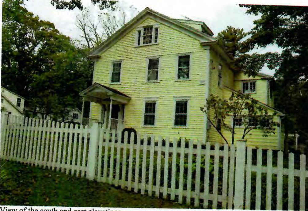
View of the south and east elevations.
