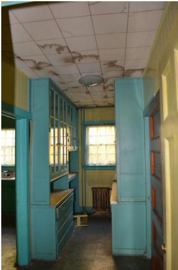
Photograph 23. Butler's Pantry, looking north from dining room
