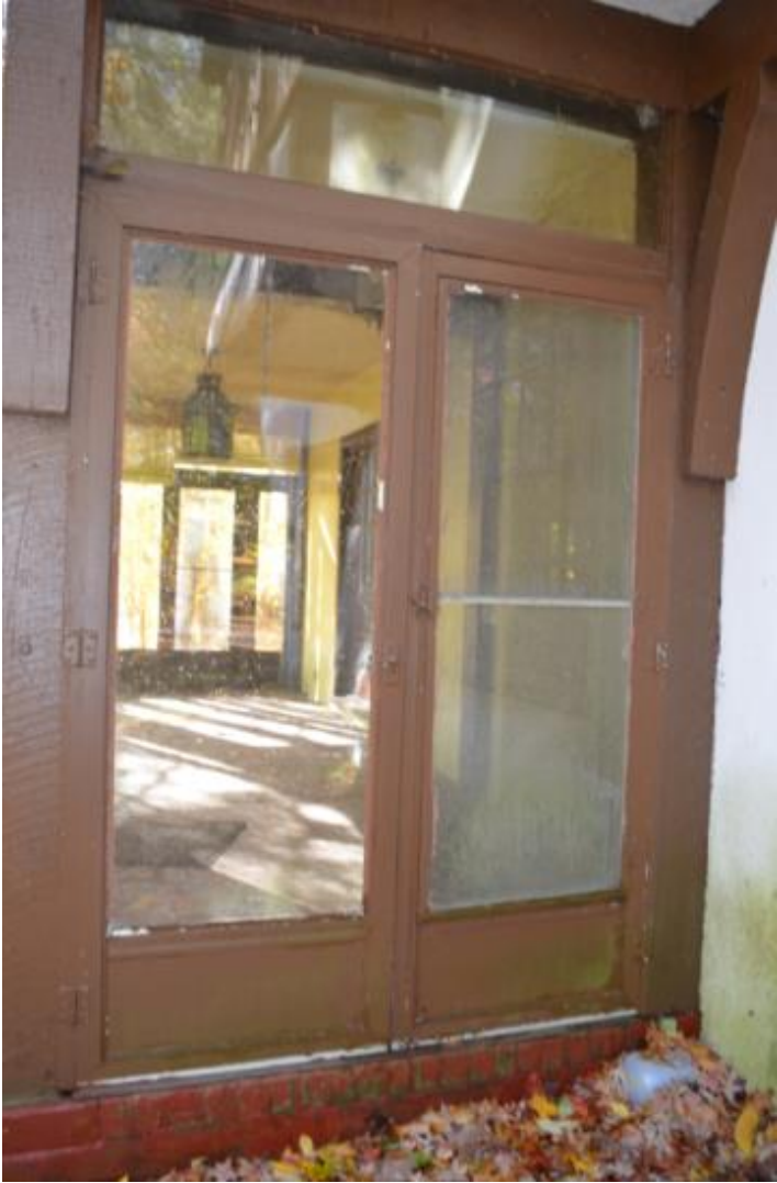
Photograph 4. Façade, east elevation, looking south at entry porch
