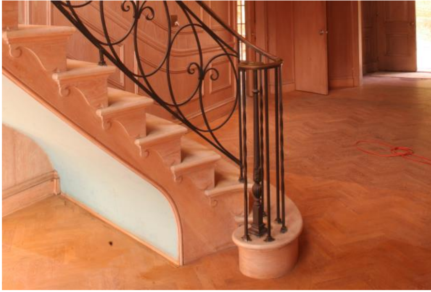
Photograph 14. Main Staircase in Foyer, stair detail, looking northeast
