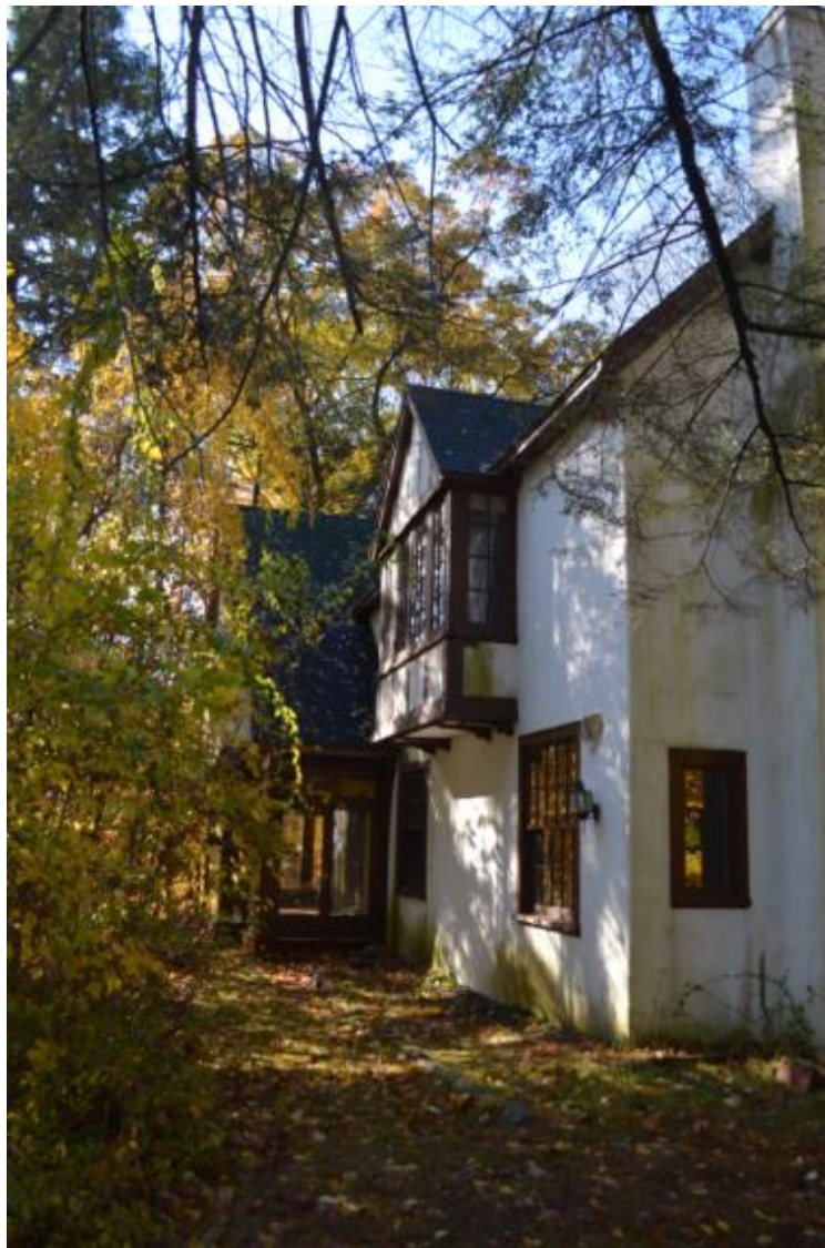
Photograph 1. Façade, east elevation looking south
