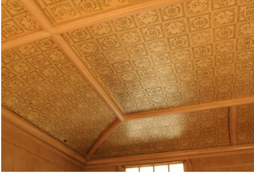
Photograph 24. Living room ceiling detail, looking southwest
