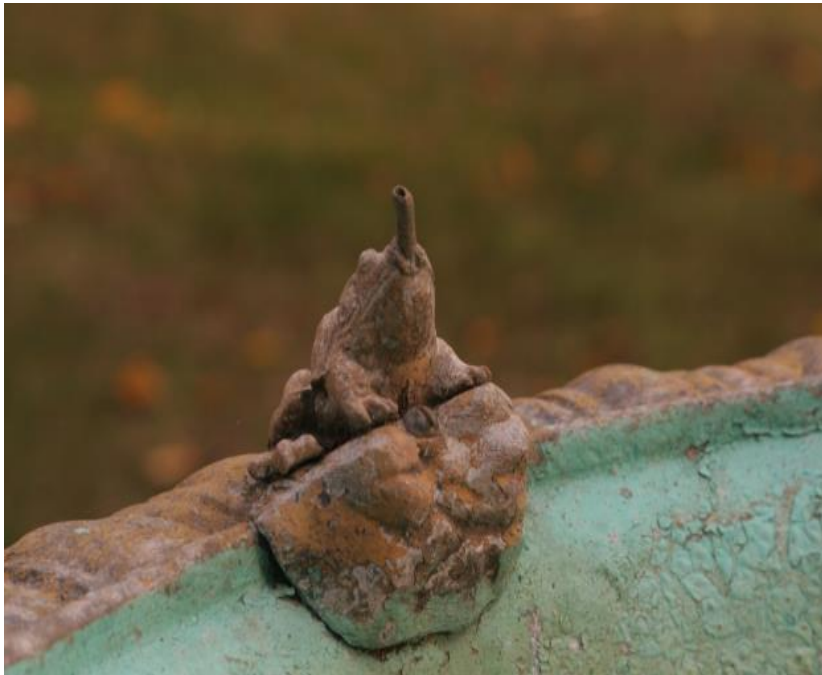
Photograph 57. Fountain, rear yard, detail
