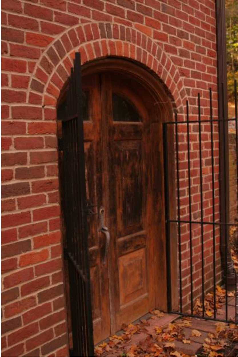
Photograph 6. South elevation, east corner entrance to basement level, looking northeast
