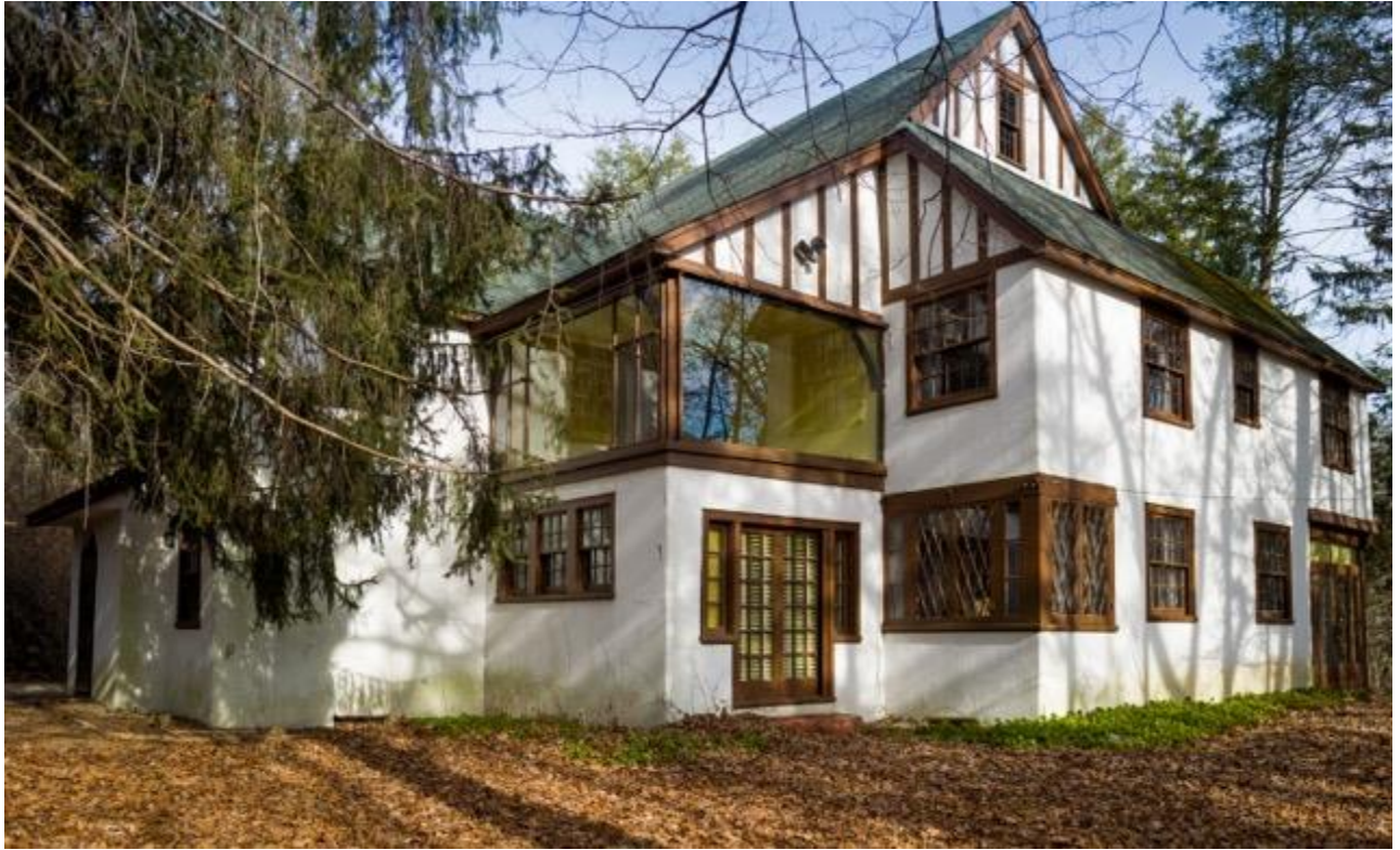
Photograph 8. West (rear) and south (side) elevations, looking northeast
