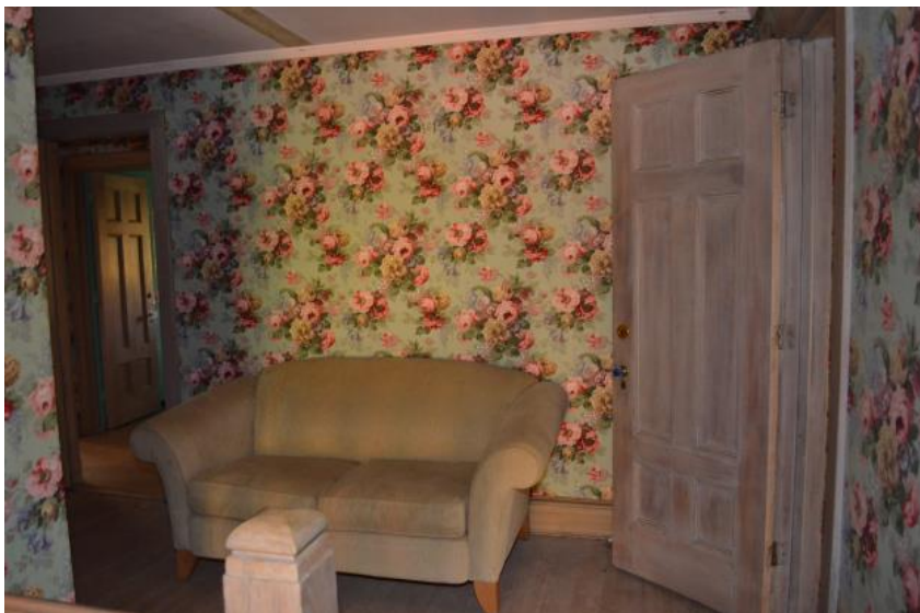
Photograph 31. Second Floor Main Hallway, looking south
