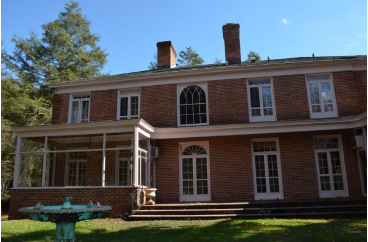
Photograph 9. West, rear, elevation, looking northeast
