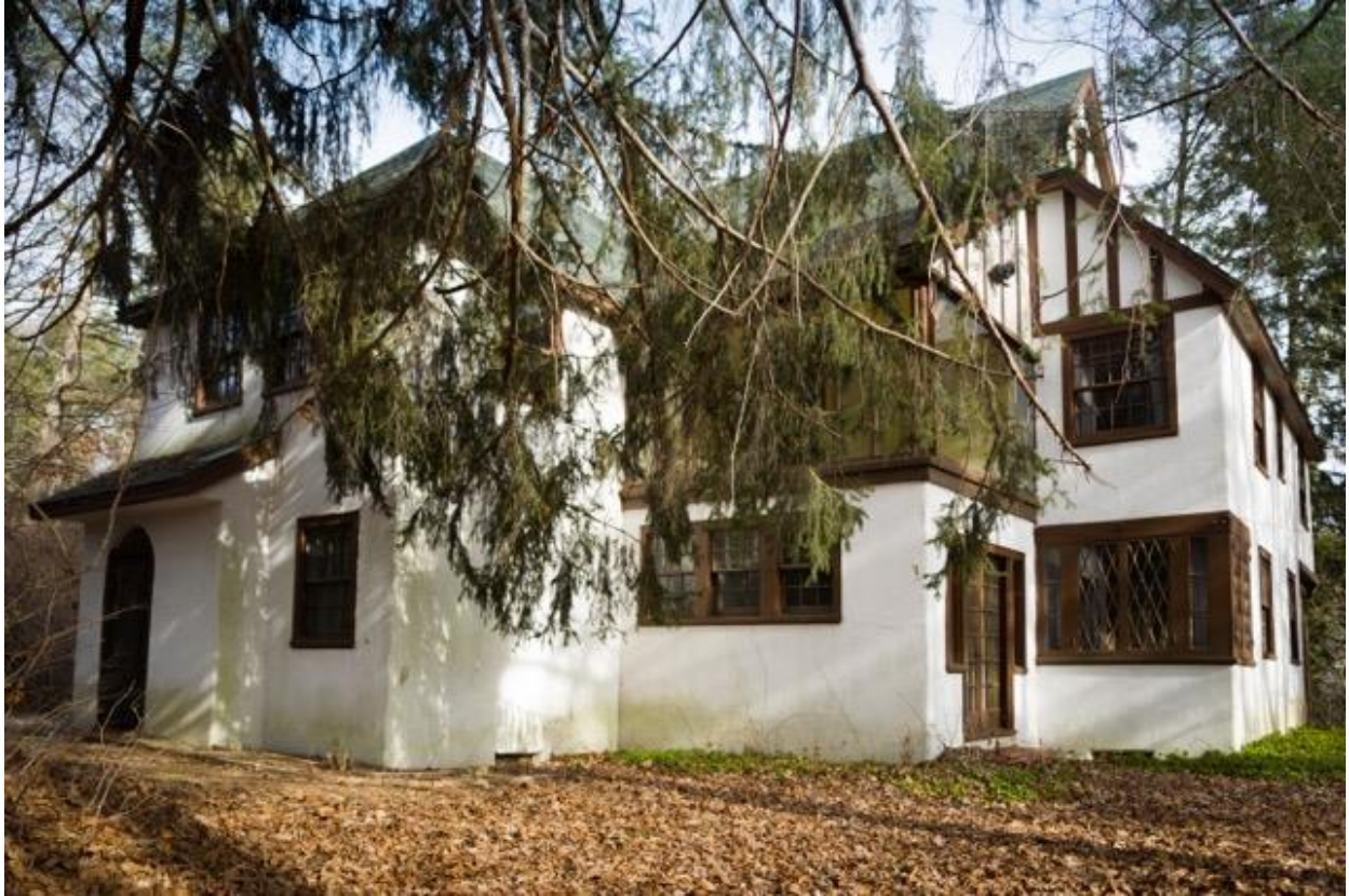
Photograph 9. West (rear) and south (side) elevations, looking northeast
