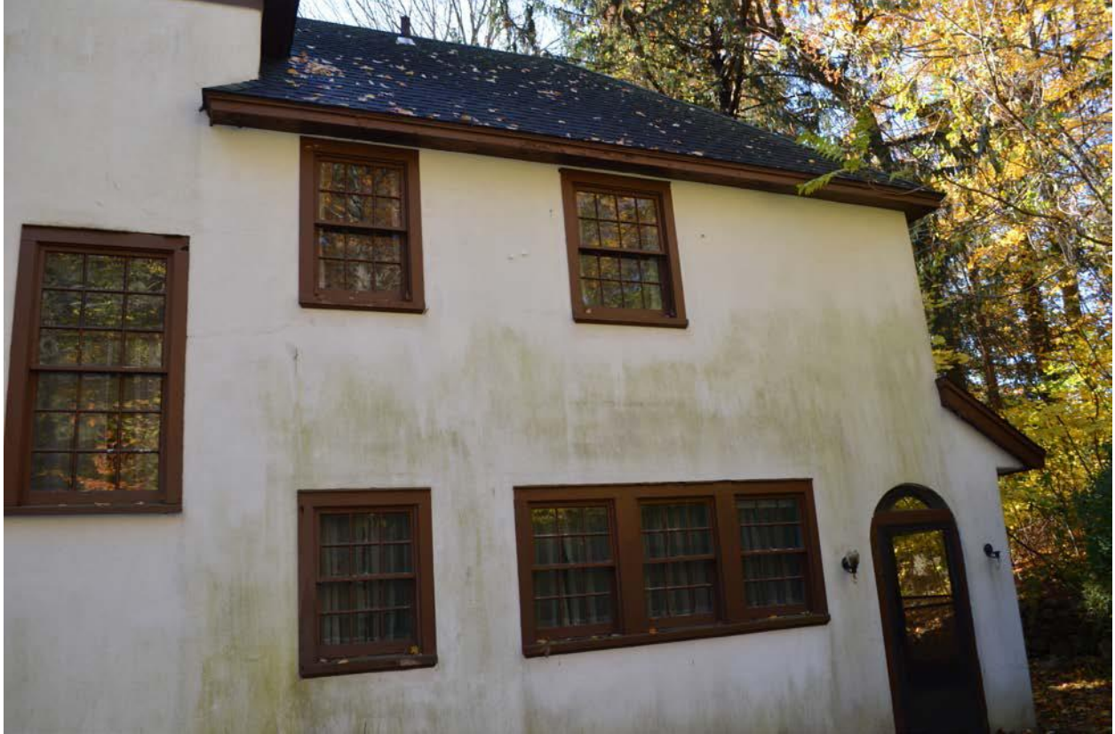
Photograph 11. North elevation, kitchen entrance, looking southwest
