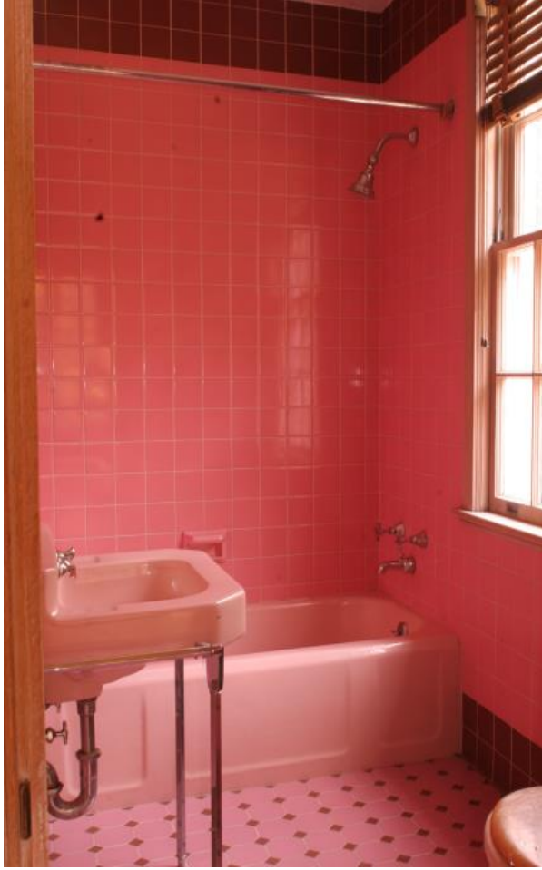
Photograph 55. Second floor front bathroom, looking north
