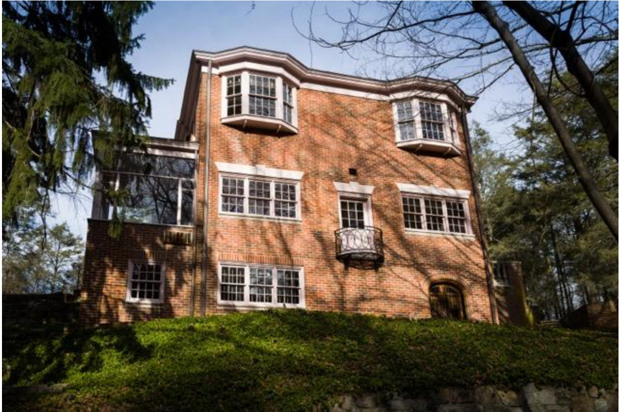
Photograph 5. South elevation, looking northeast from depressed lawn area
