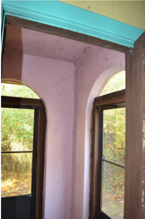
Photograph 27. Rear entry at kitchen, looking northwest
