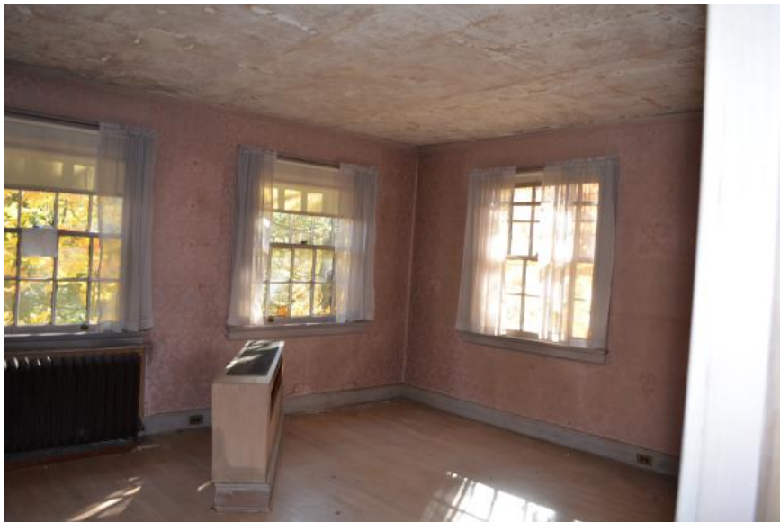
Photograph 37. Front Guest Bedroom, looking southeast
