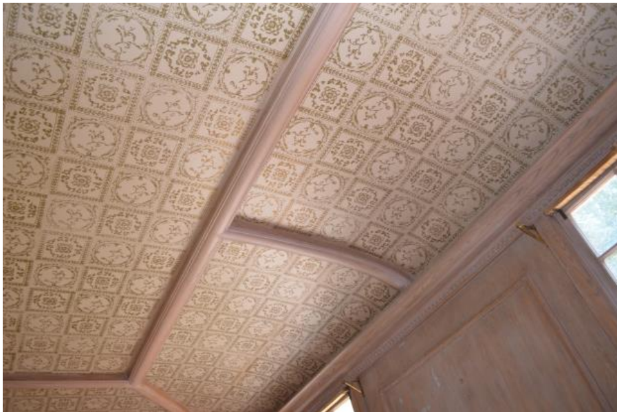
Photograph 23. Living room ceiling detail, looking northeast
