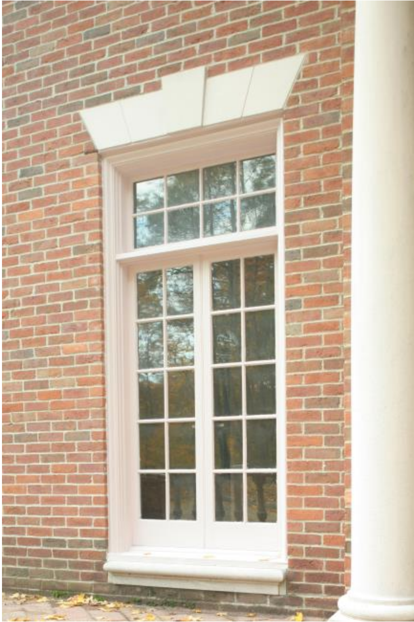
Photograph 3. Façade, east elevation, French door detail, looking southwest
