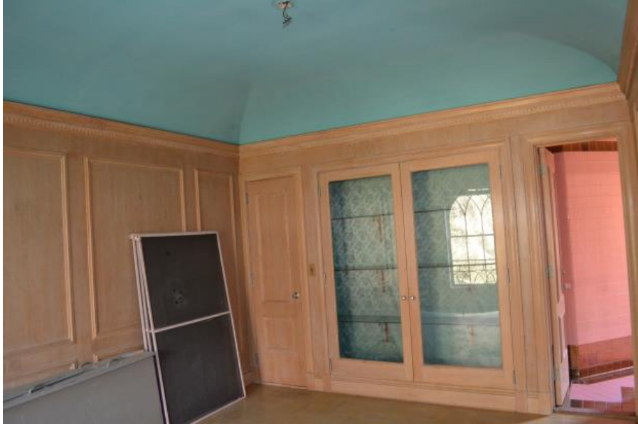
Photograph 39. Second Floor hallway, closet wall, looking northeast
