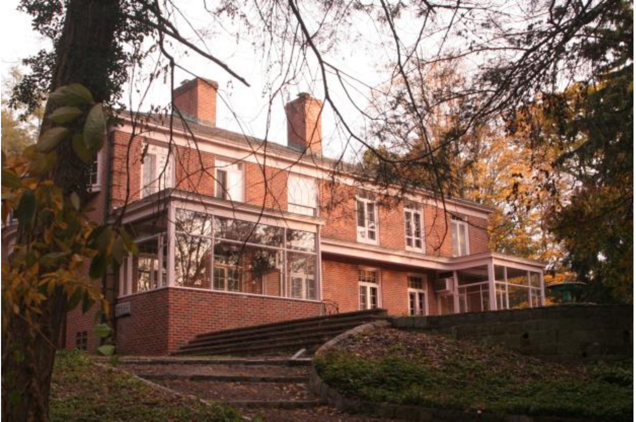
Photograph 8. West, rear, elevation, looking southeast
