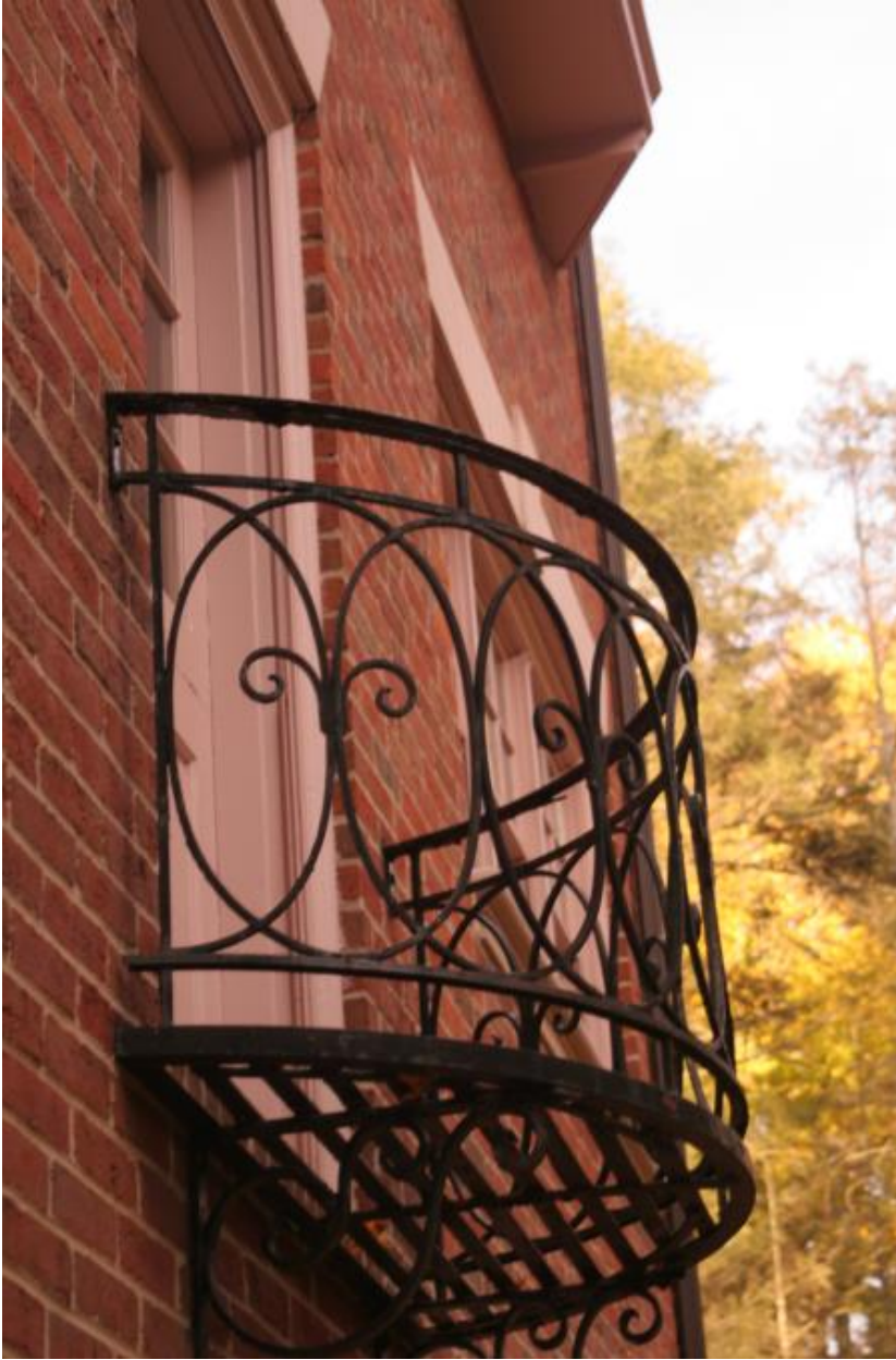
Photograph 7. South elevation, Juliette balcony, looking northeast
