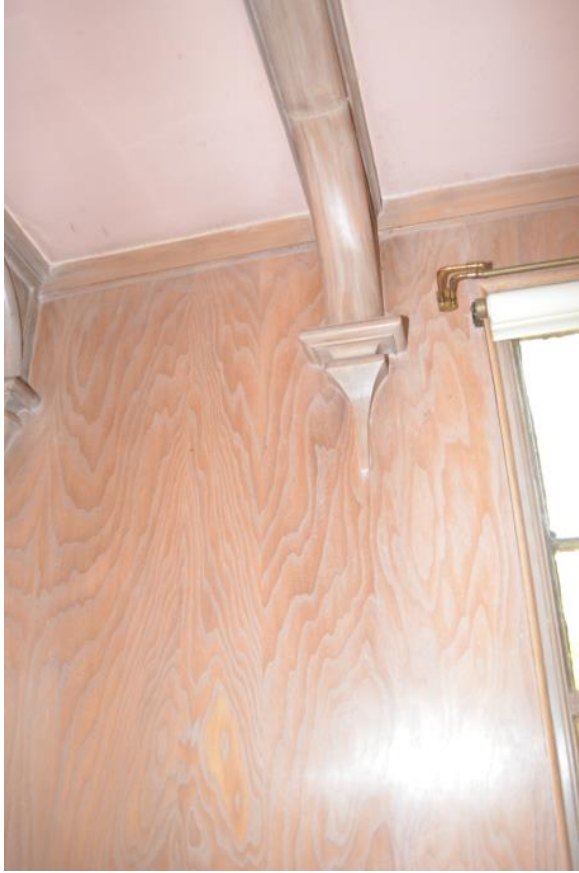
Photograph 14. Living Room, looking up at ceiling at northeast corner
