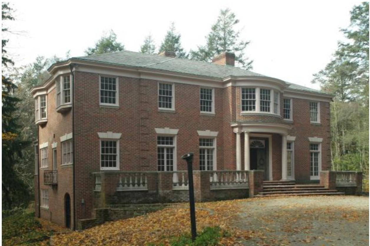
Photograph 1. Façade, east elevation, looking northwest
