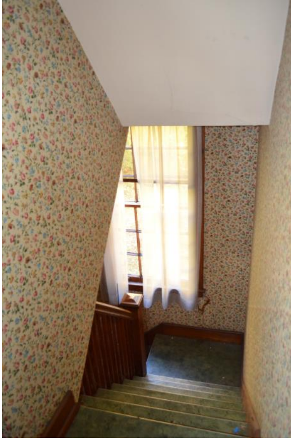
Photograph 42. Service stairwell, looking down and north from second floor landing
