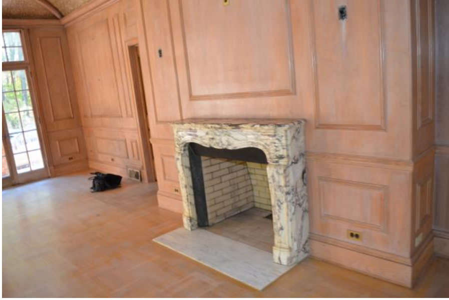
Photograph 22. Living Room, mantle, looking southeast
