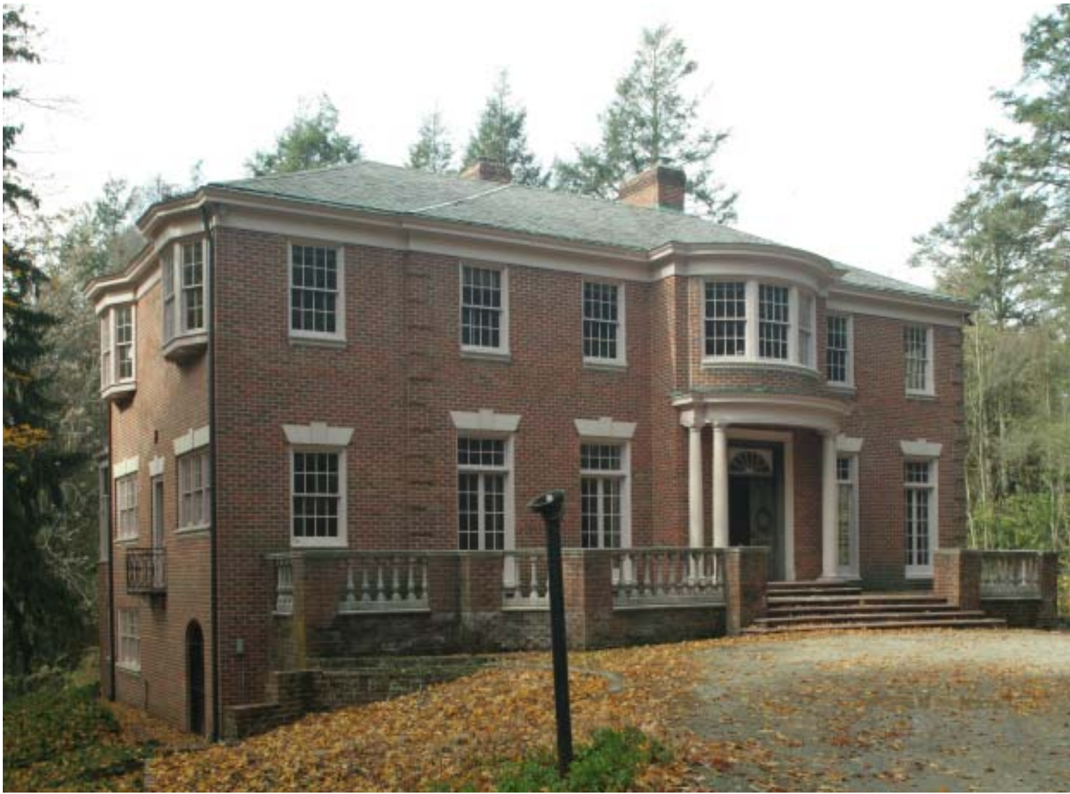
Golden Shadows, East and South elevations, view: southeast to northwest.
