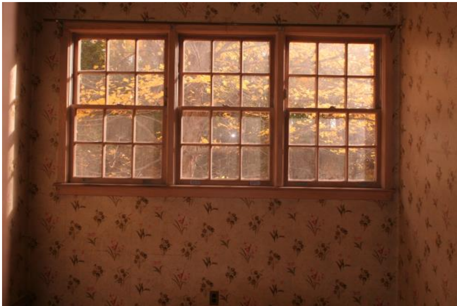
Photograph 35. Study off butler's pantry, looking south
