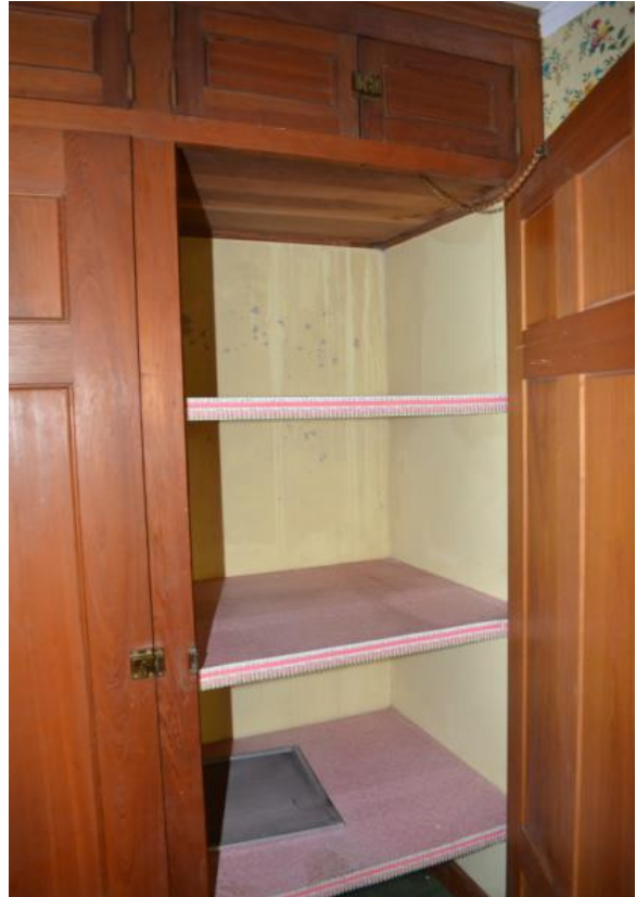
Photograph 43. Service wing closet, looking south
