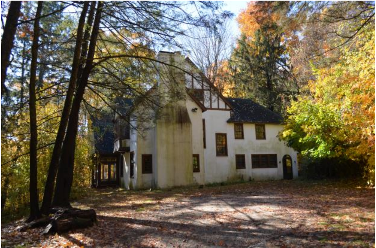
Photograph 10. North elevation, looking south
