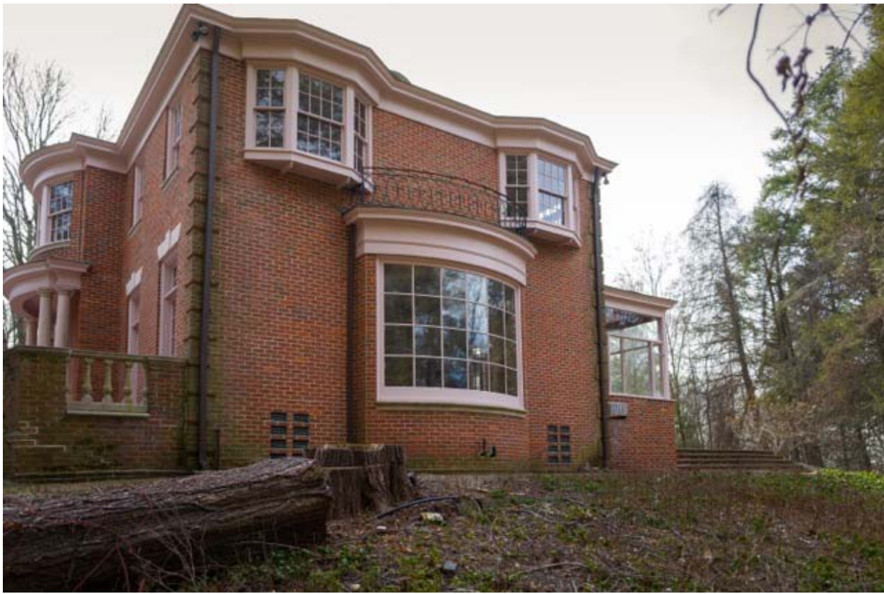
Golden Shadows, north and east façade, view: northeast to southwest
