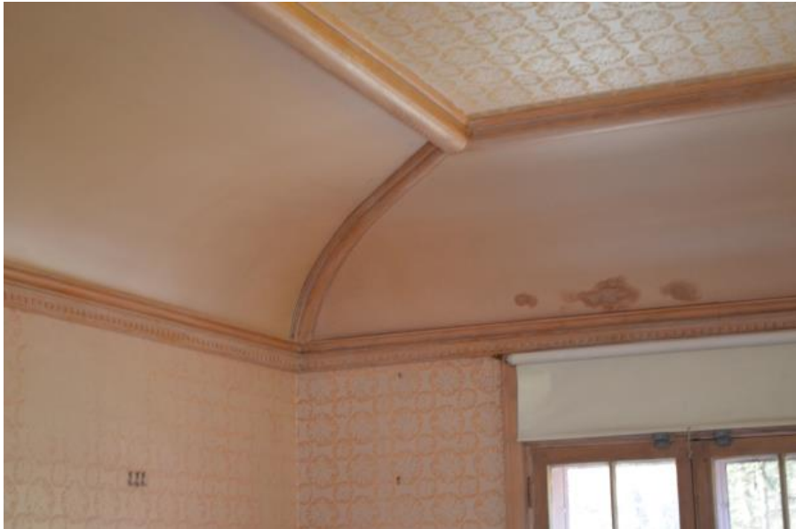
Photograph 44. Lady Evelyn's Bedroom, ceiling detail, looking northeast
