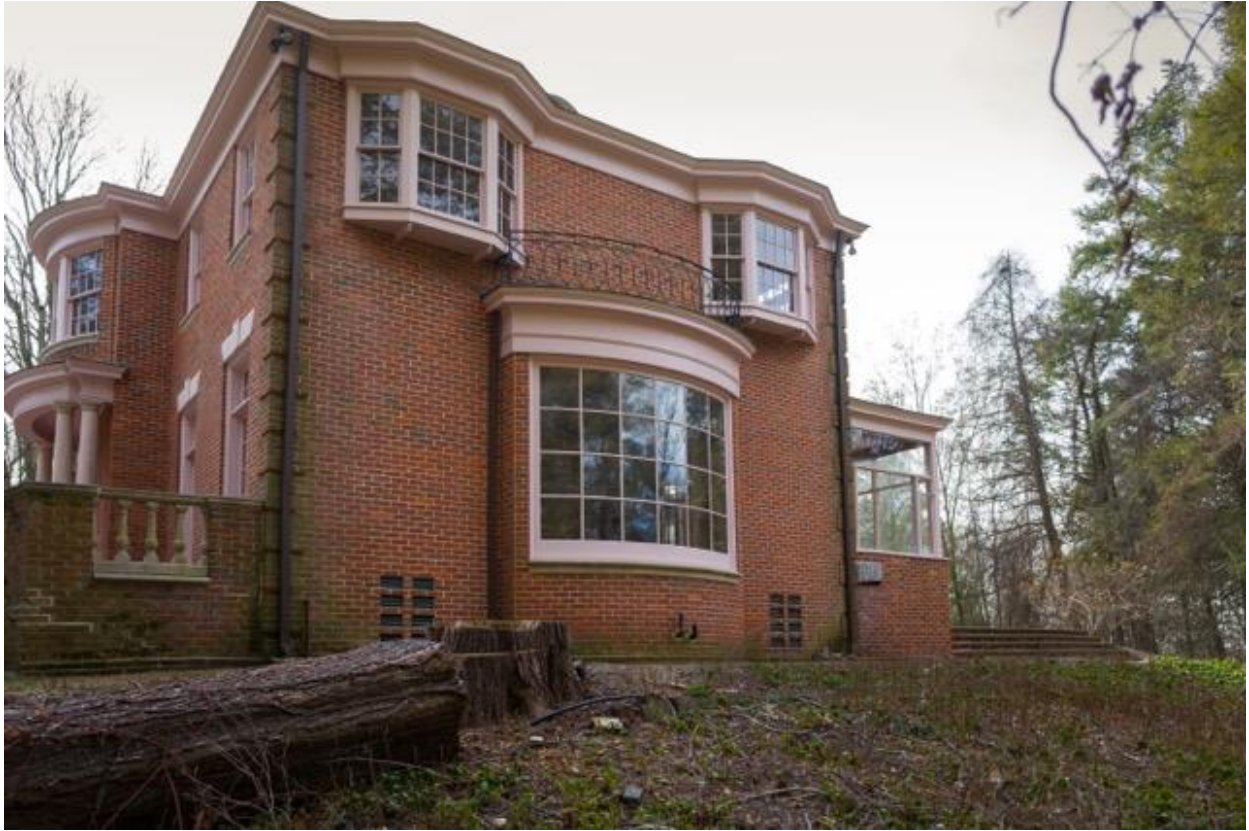
Photograph 12. North, side, elevation, looking southwest
