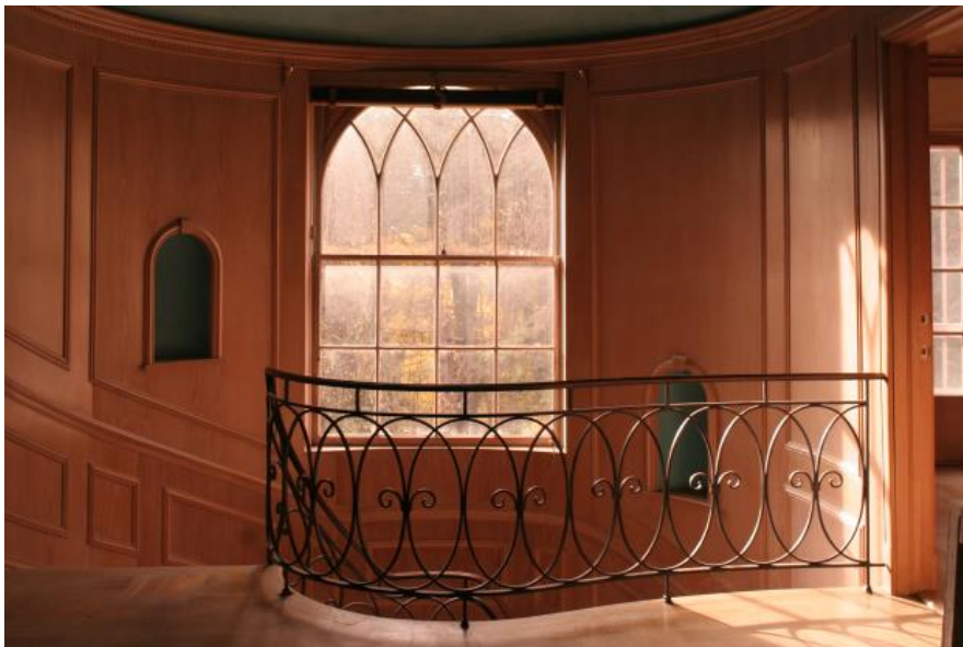
Photograph 15. Adamesque arched window at stairwell second floor, looking west
