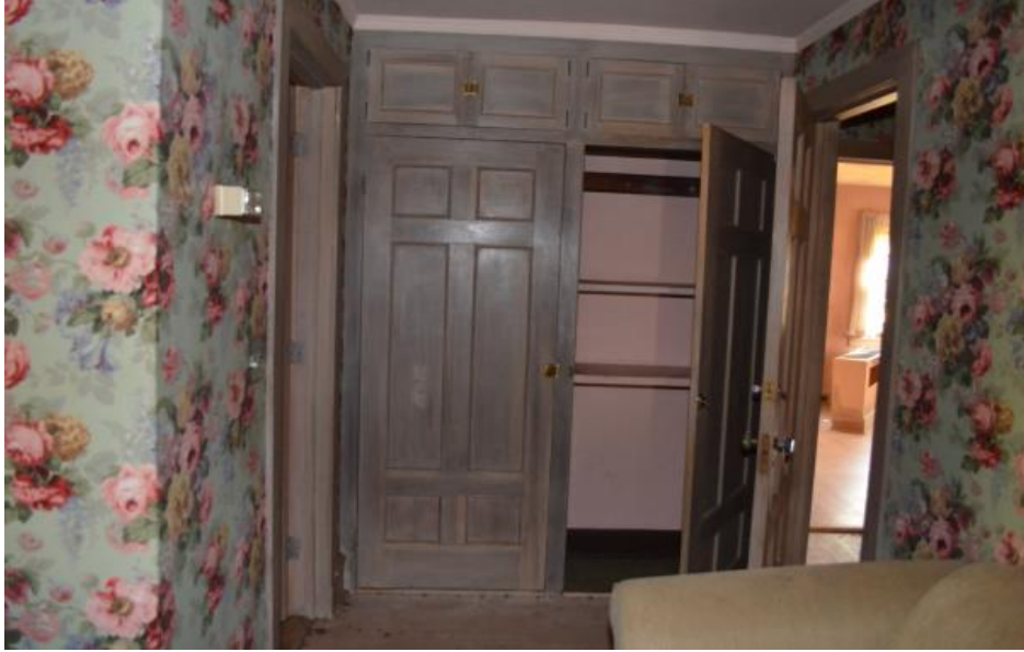
Photograph 32. Second Floor Main Hallway closet, looking east
