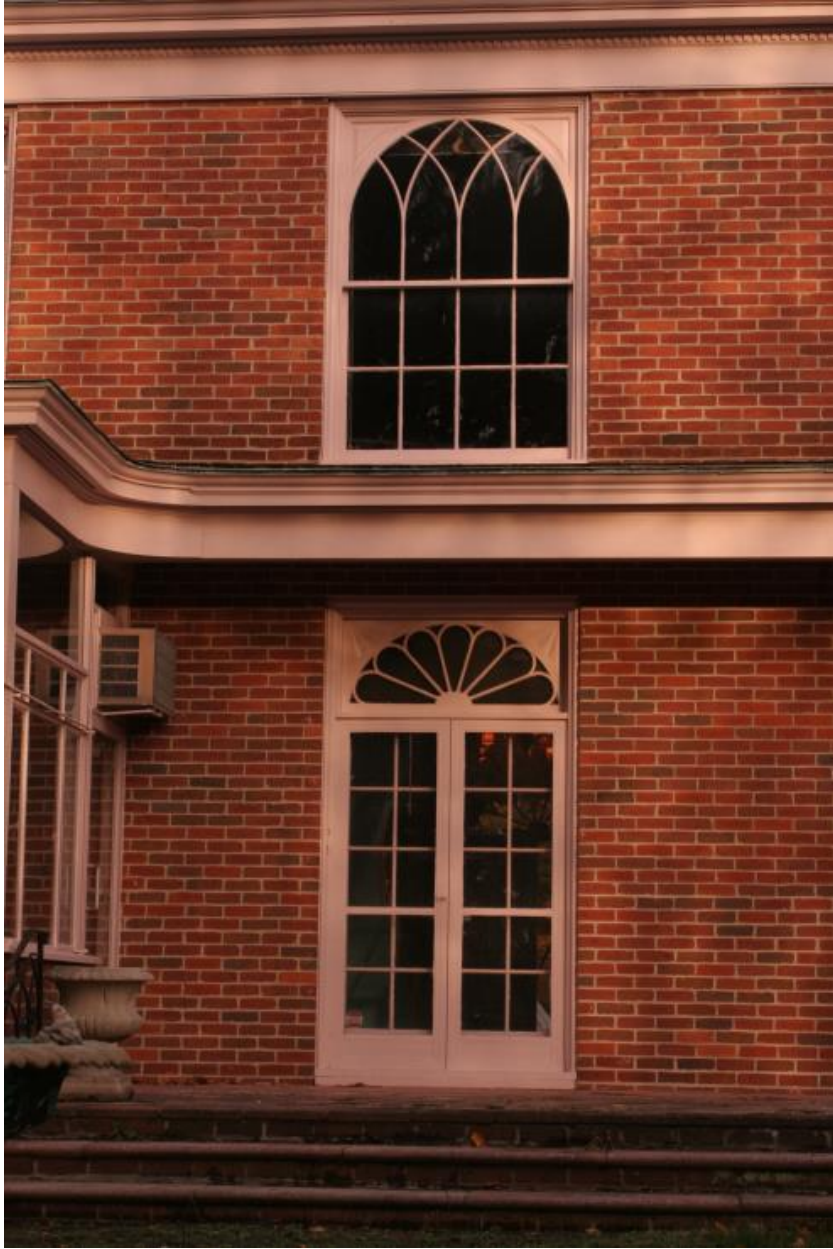
Photograph 11. West, rear, elevation, looking east
