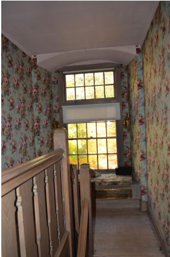
Photograph 30. Main Stair Case window, looking north from second floor landing
