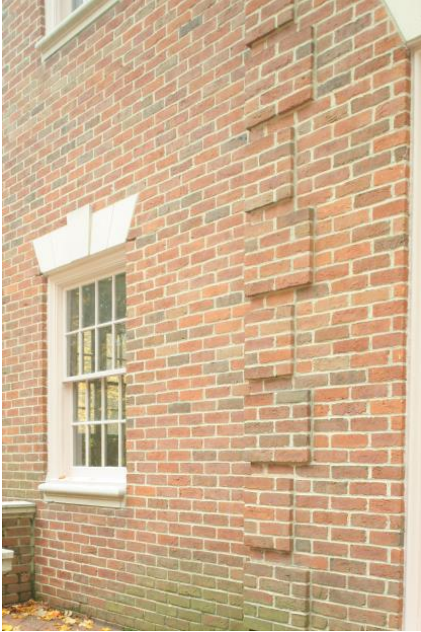
Photograph 4. Façade, east elevation, Quoining detail, looking southwest
