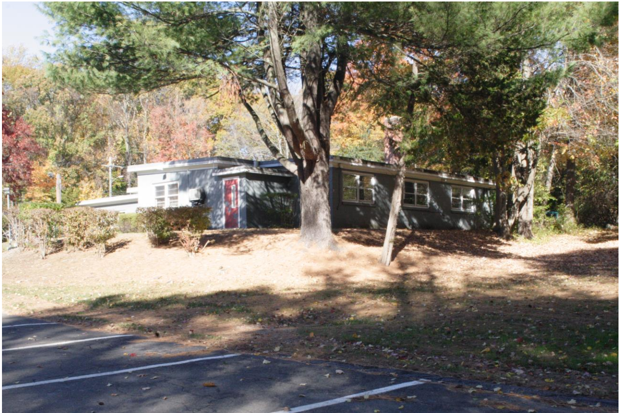
3. (ID-0453) View northeast of BR-73 Nike Hq Barracks, Offices & BOQ. Presently Westport-Weston Health District Offices
