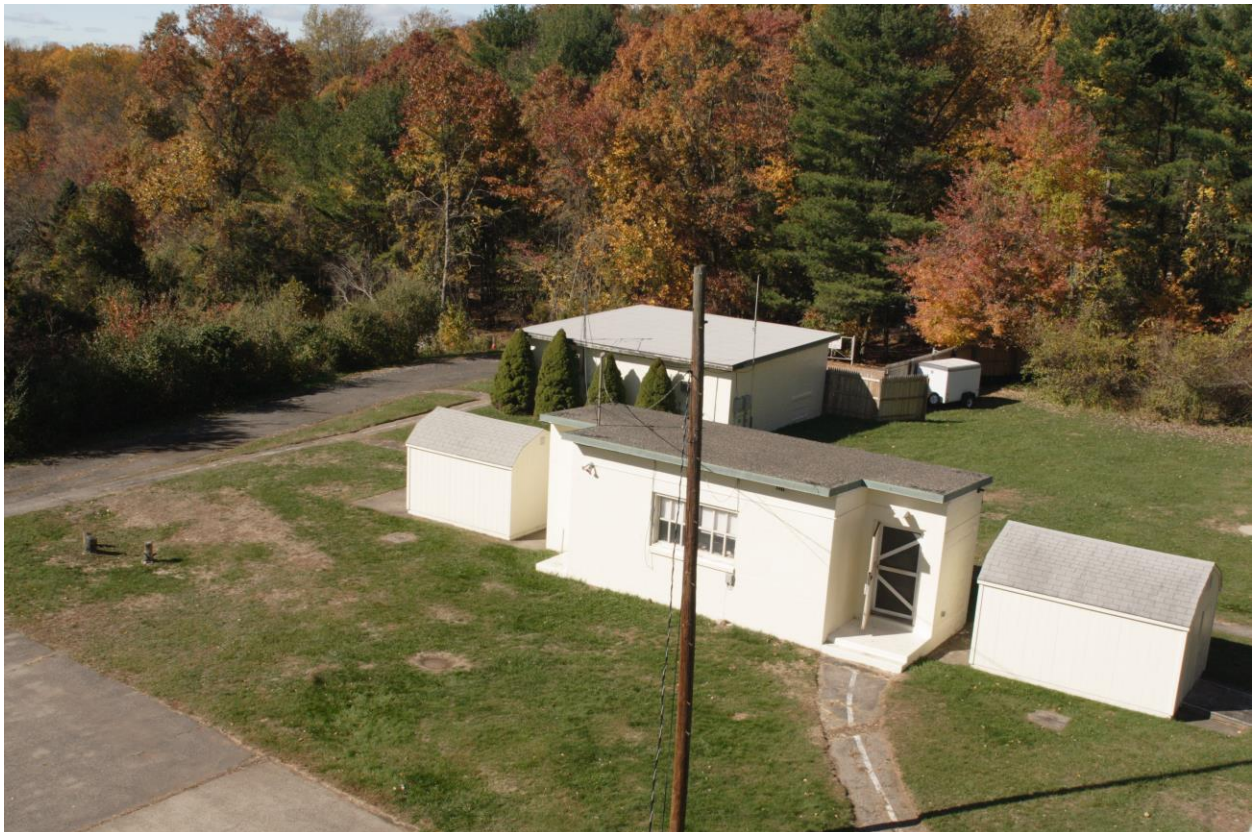
10. (ID-430) View northwest from tower of former BR-73 communications & control center. Currently offices of the Westport Astronomical Society.
