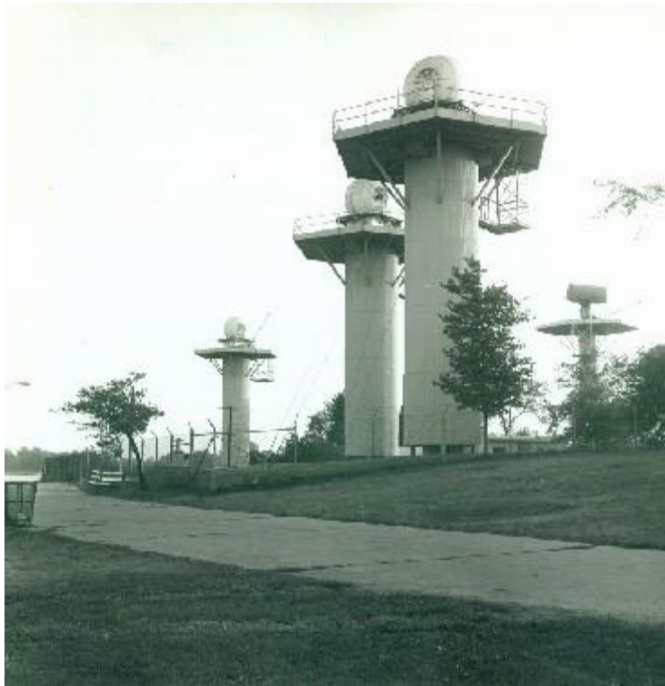
Figure 6 - View of typical Nike concrete radar towers. Similar towers formed the support for the Rolnick Observatory in Westport.
