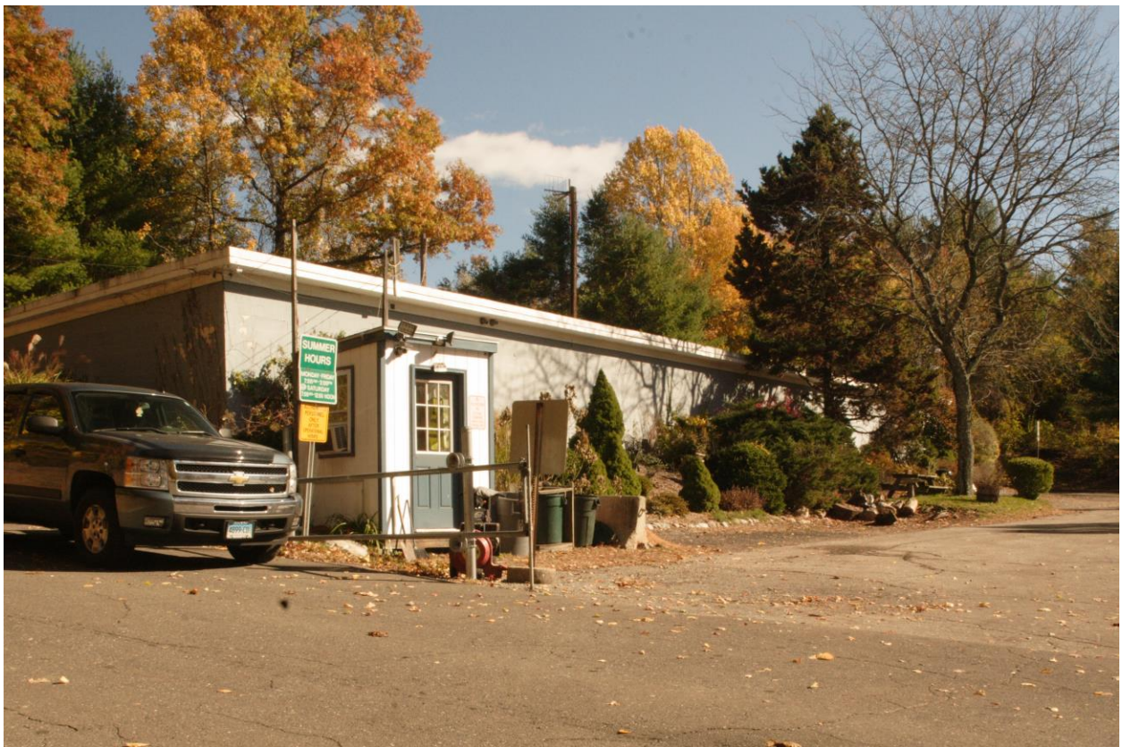
4. (ID-0450) View southeast of BR-73 Nike Mess Hall, Kitchen & Recreation Building. Presently Public Works facility and Westport archival storage.
