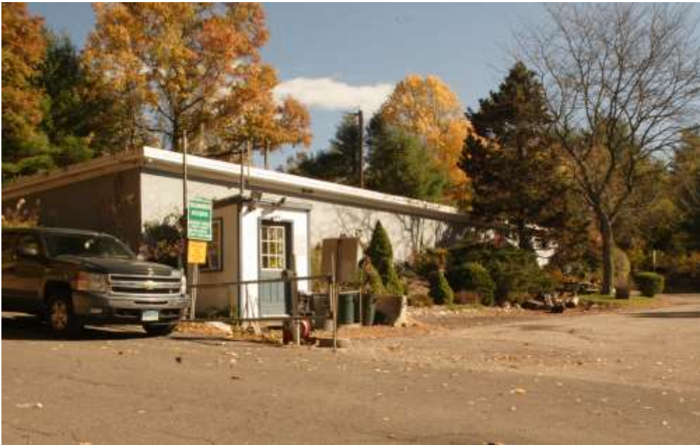
View southeast of BR-73A Nike Mess Hall, Kitchen and Recreation Building. Presently, Public Works facility and Westport archival storage.
