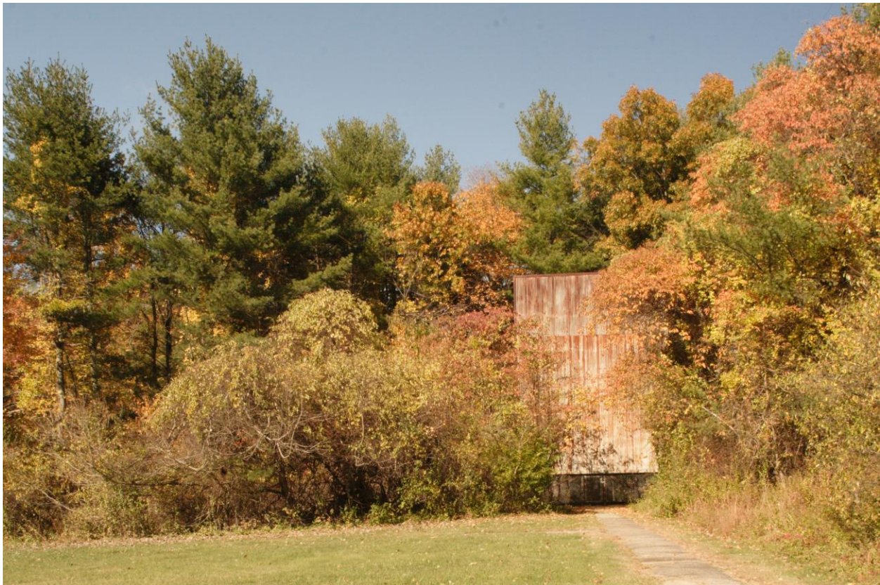
12. (ID-0414) View north of former BR-73 north radar tower. Proposed to be antenna tower for the Westport Astronomical Society's Amateur Radio Club – station KB1WLW.
