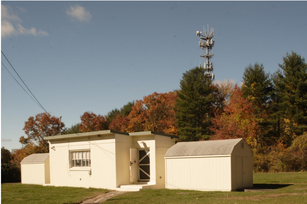
11. (ID-0412) View northwest of former BR-73 communications & control center. Currently offices of the Westport Astronomical Society.
