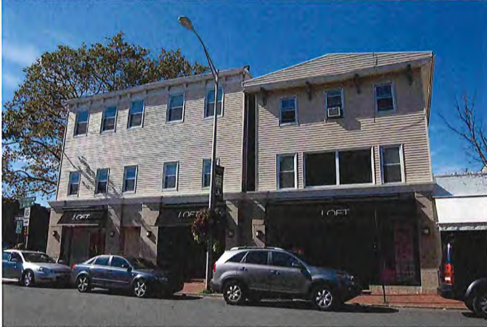
View of the east elevations.
