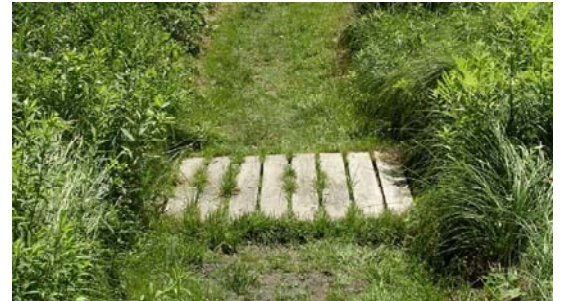
Figure 3-3. Wooden boardwalk in seasonally wet area (Gisland Farm Audubon Center, Falmouth, ME).
