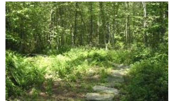
Figure 3-4 Large granite step stones through a seasonally wet area (Browning Woods Trail, South Kingstown, RI).
