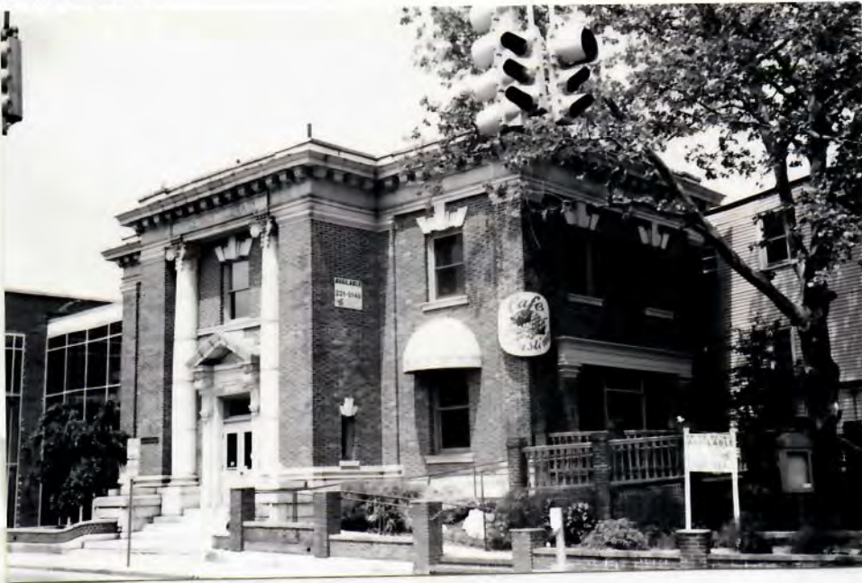
View from the southeast.
