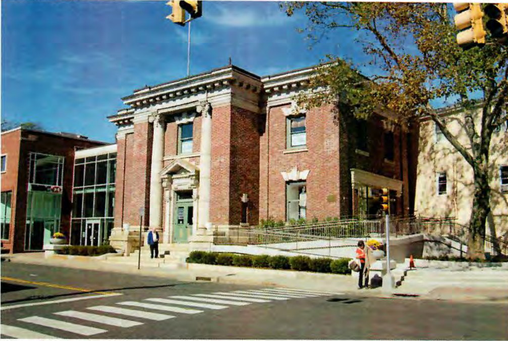
View of the south and west elevations.
