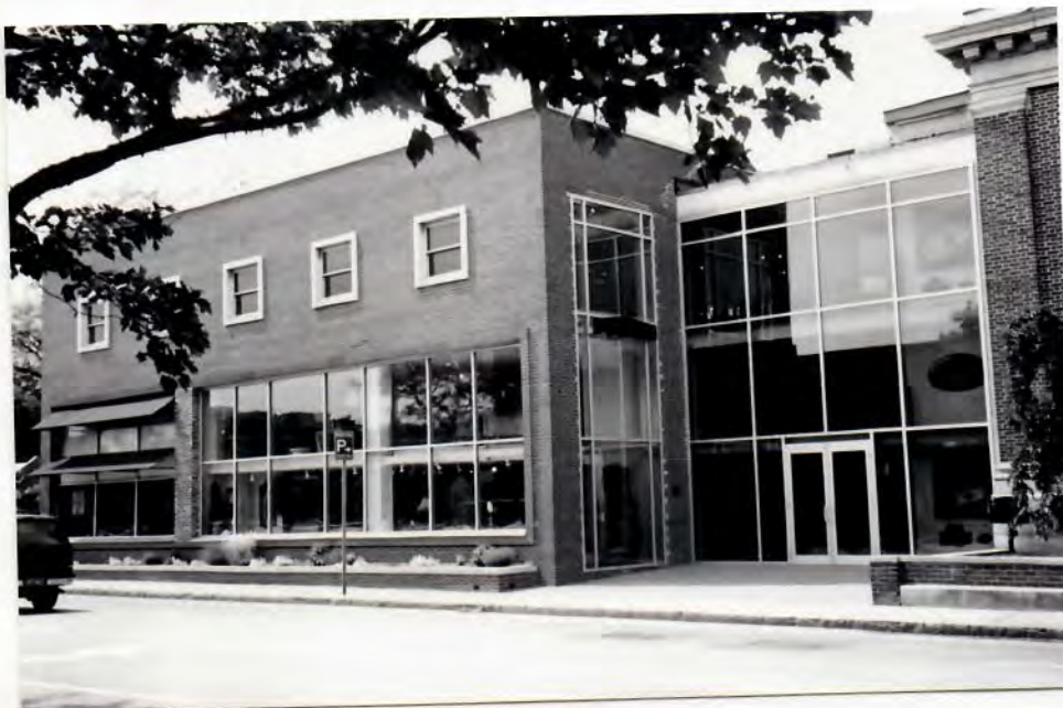
View of the south elevation of the west wing.
