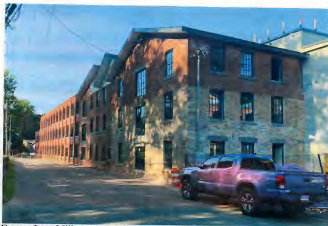
Former Lees Mill, east elevation looking south
