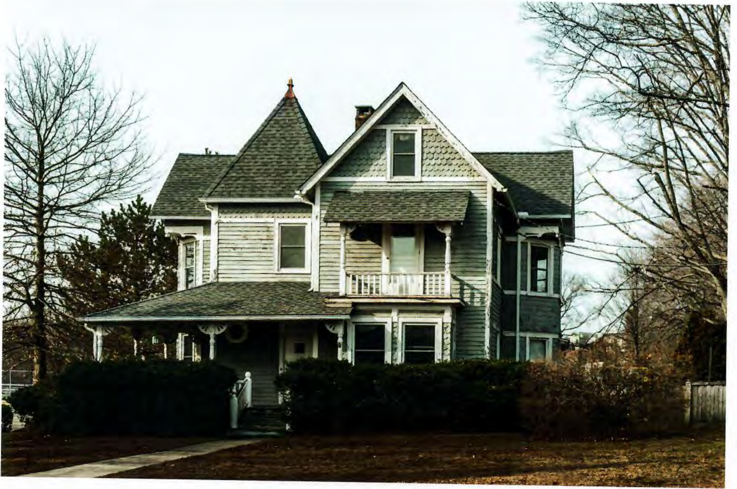
Photo 1. 136 Riverside Avenue, view southwest showing facade.
