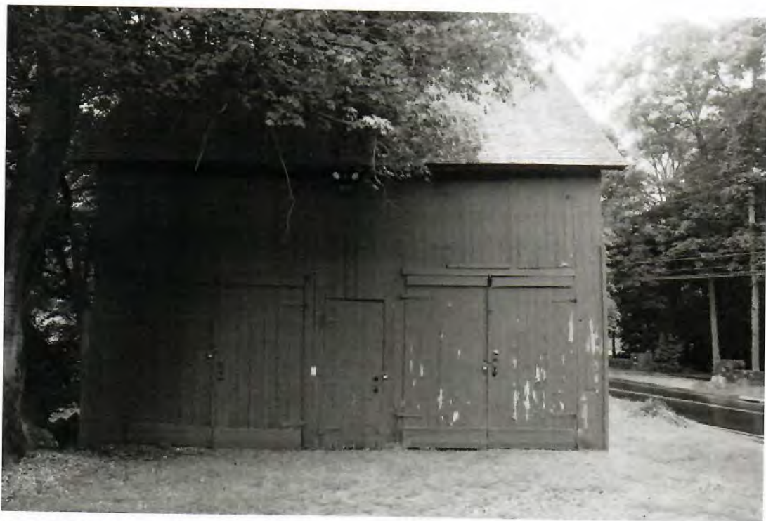
6. South view of Barn, camera facing north.
