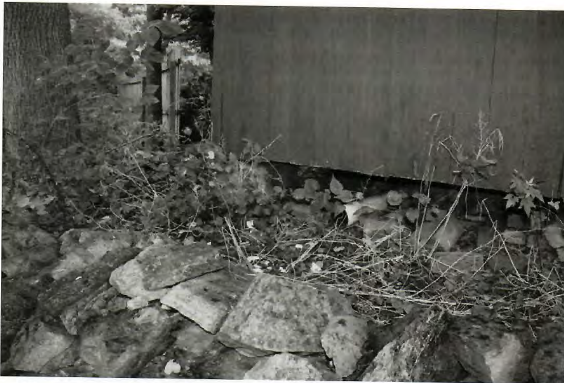
12. Detail of the exterior, northwest corner of the barn. Note the single stone pier at the corner.
