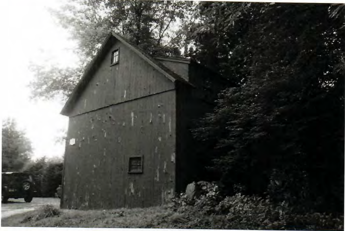
9. Northeast corner view of barn, camera facing southeast.
