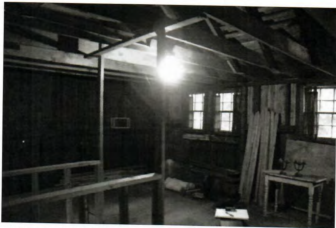
14. Attic level of barn, camera facing northwest.
