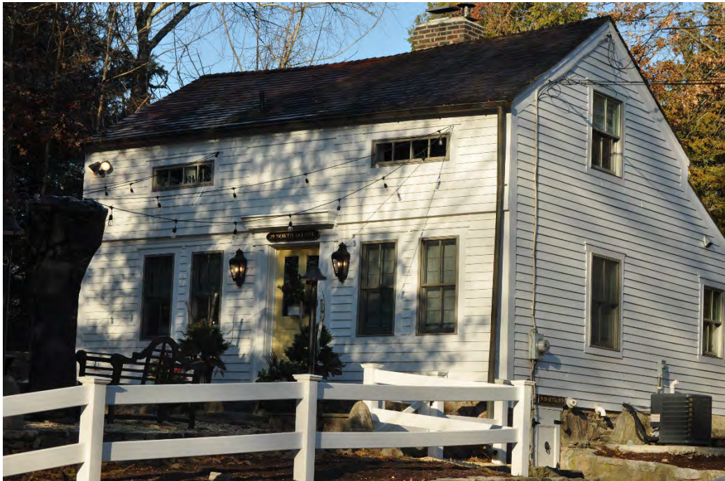
Photograph 1-2023: Post and Rail fence from North Avenue, tandem windows on top and two windows on each side of front door.
