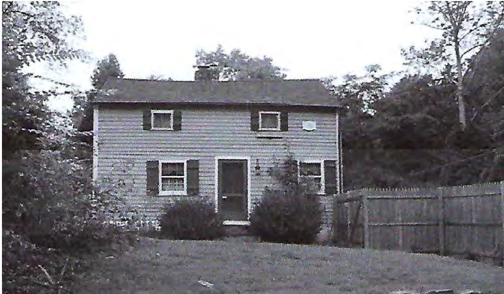
Prior to 2023 from Barn Survey – Stockade Fence on North Avenue Side and windows
