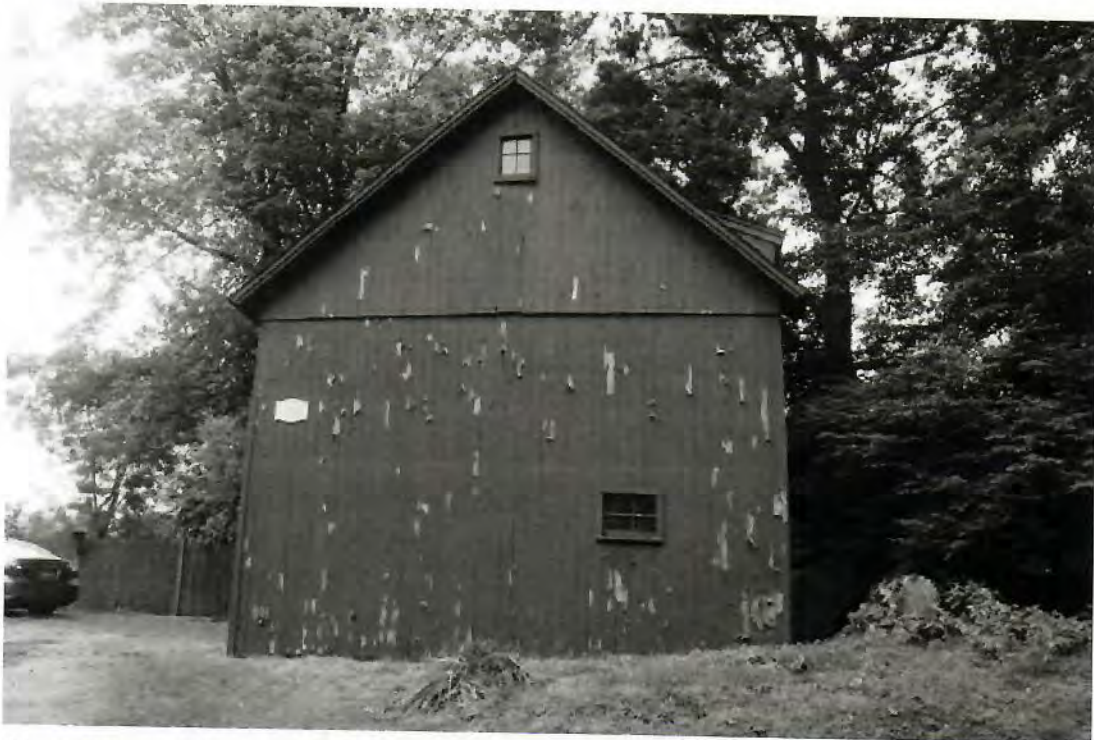
8. East gable-end view of Barn, camera facing west.
