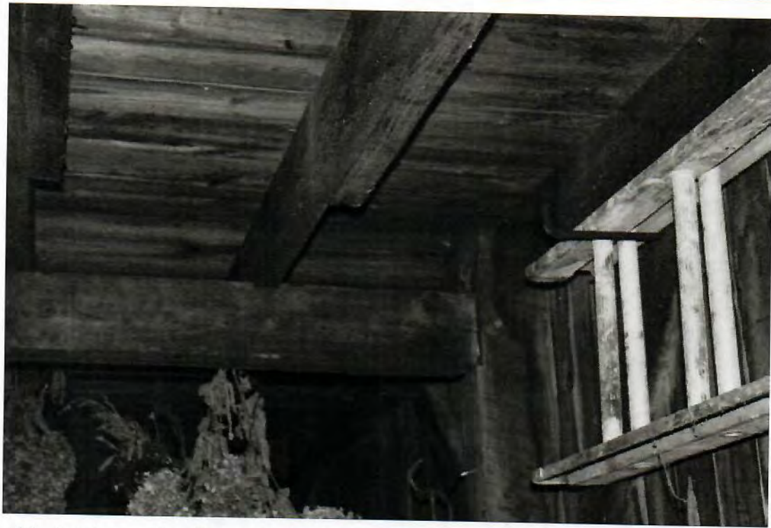
13. Detail of the interior, north wall, main level, square rule construction and circular sawn posts, camera facing east.
