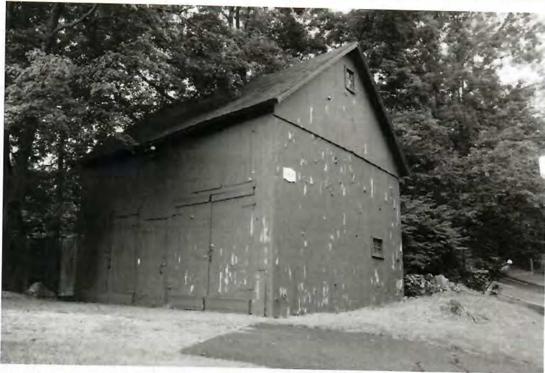
7. Southeast corner view of Barn, camera facing northwest.
