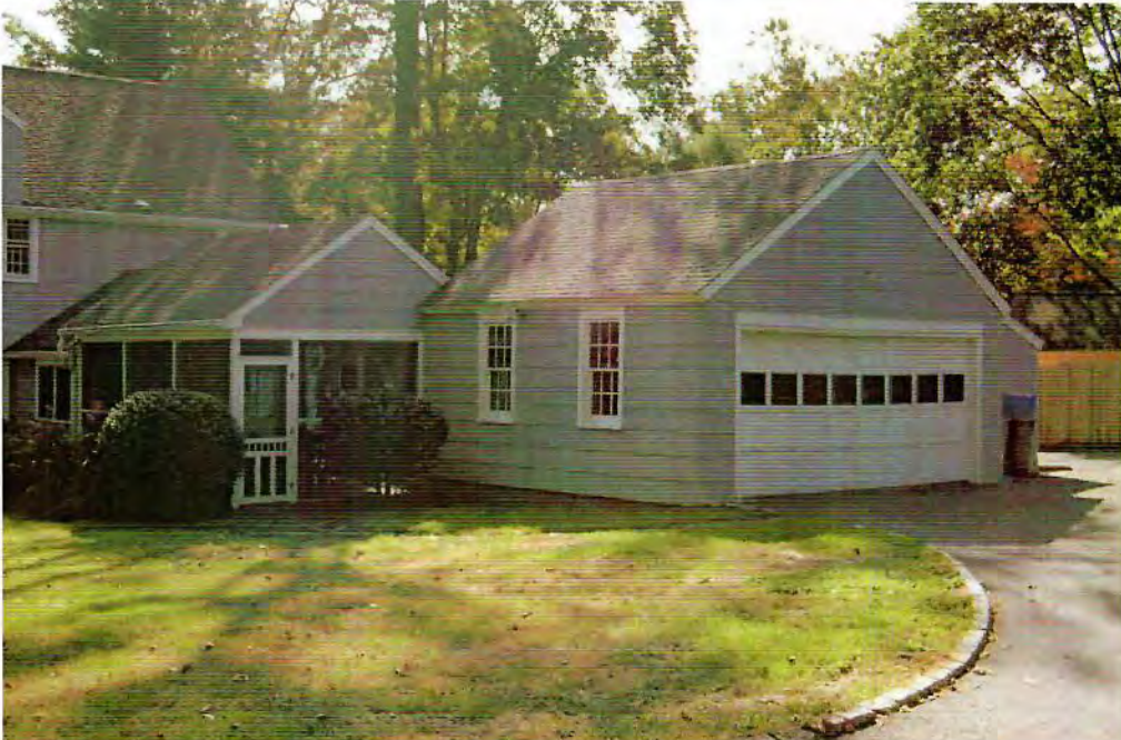
View of the west elevation of the attached garage and screened-in porch.
