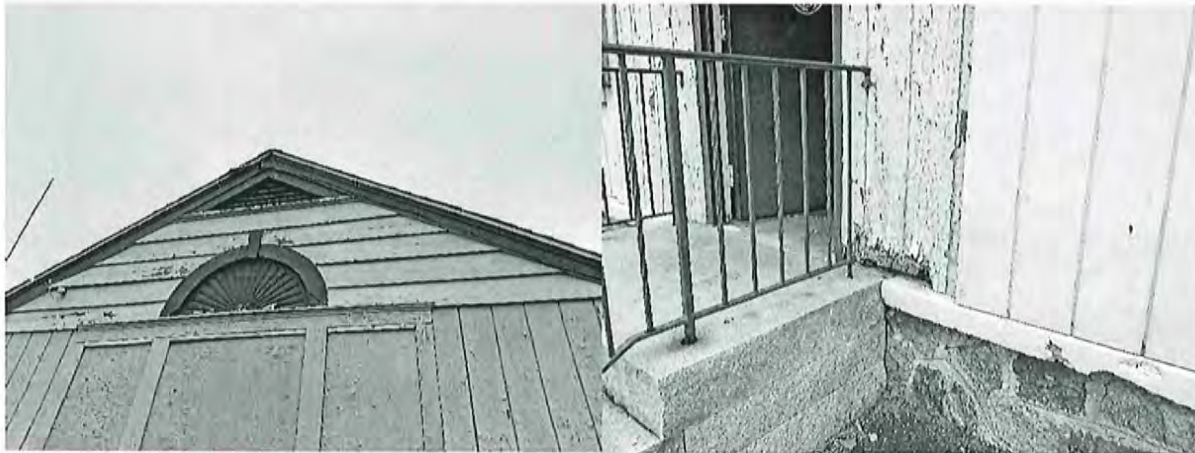
Gable venting is adequate.
