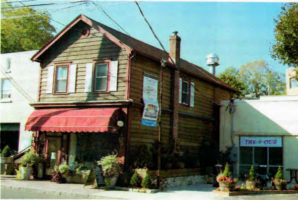
View of the east and north elevations.
