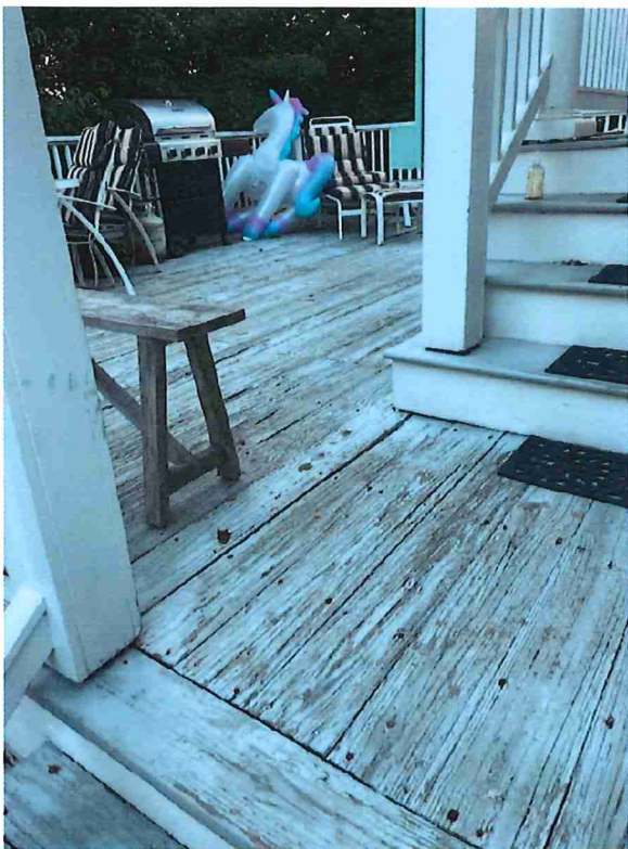
Deteriorated decking is splintered.
