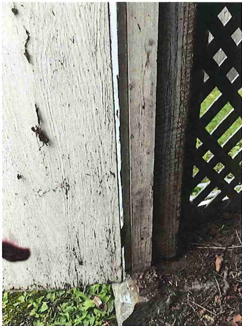
Posts sitting on stone foundations
