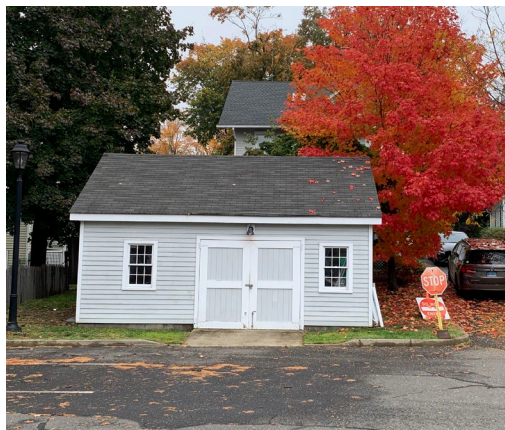
65 Myrtle Avenue, garage (wagon house), looking east
