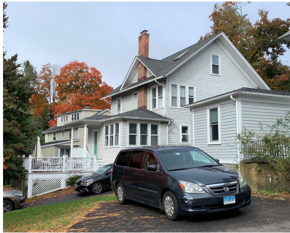
65 Myrtle Avenue looking north
