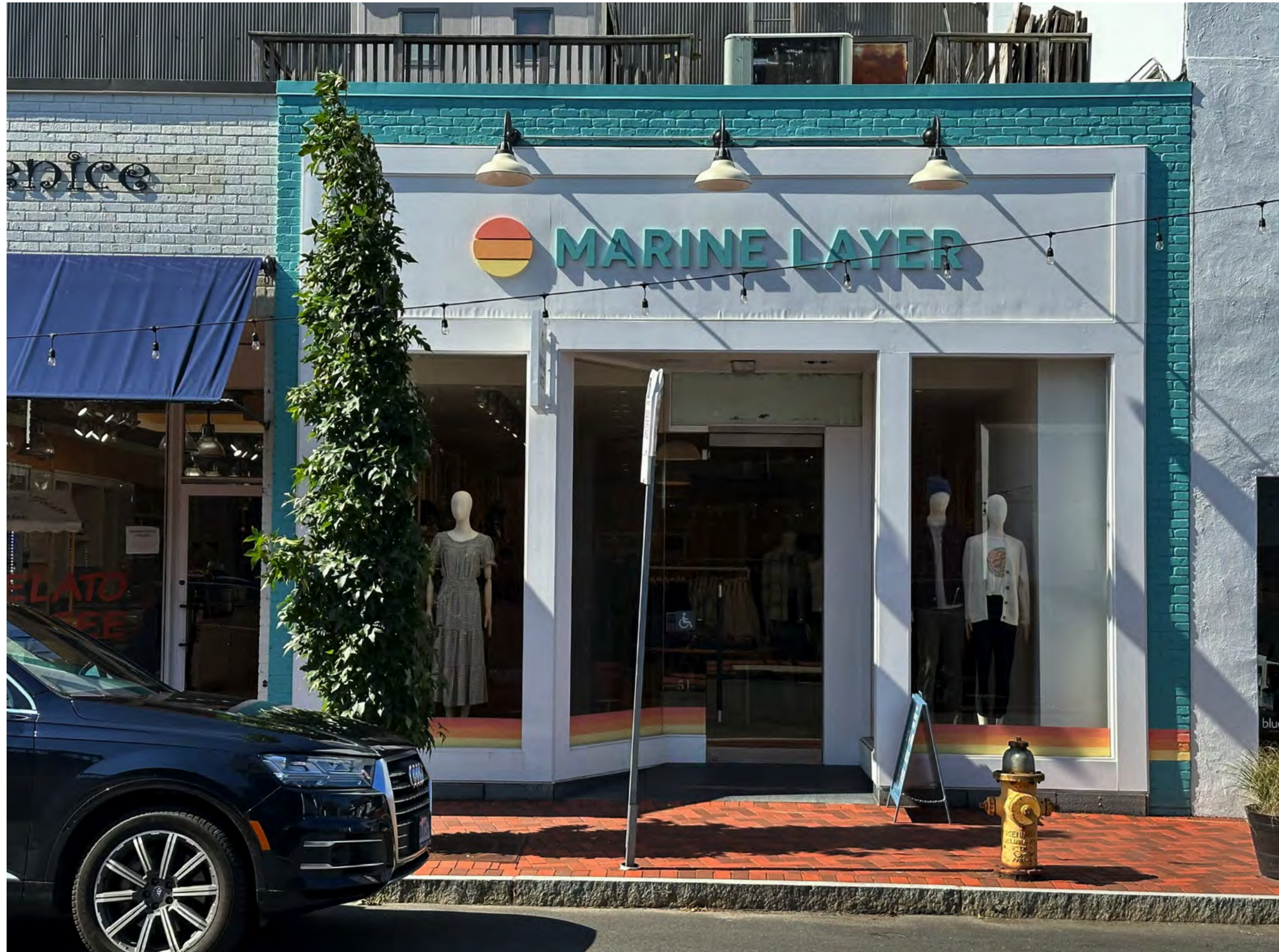
1 EXISTING MARINE LAYER FACADE
