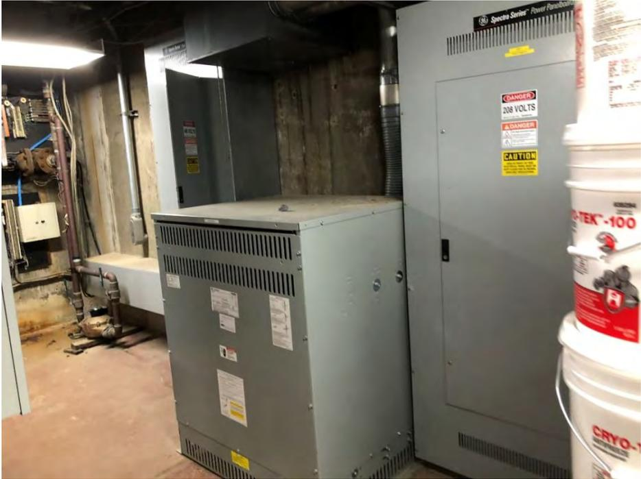
Figure E12: 225 kVA Transformer and Generator Standby Power Panel EDP-1
