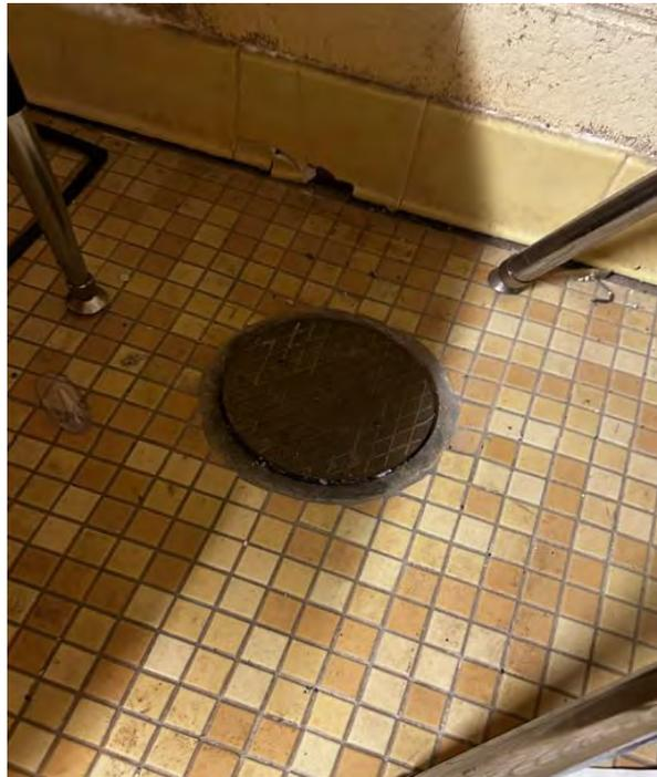
Figure P6: Raised Floor Cleanout
