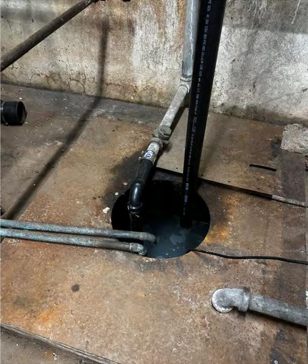
Figure P7: Basement Waste Sump Pump
