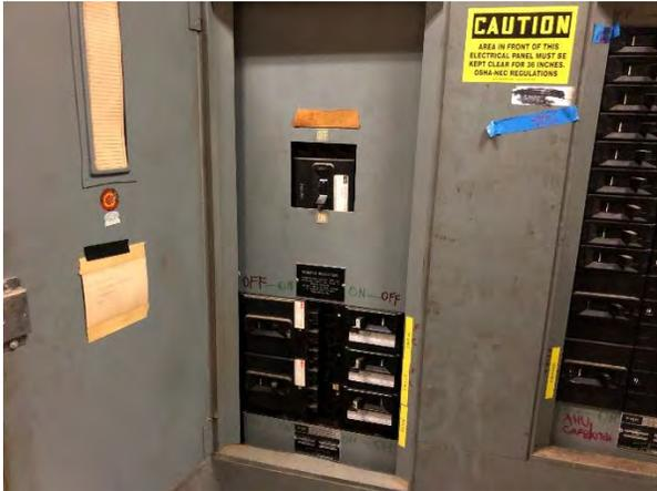
Figure E9: Recessed Wall-Mounted Power Panel in Kitchen
