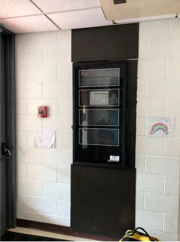
Figure E14: Notifier Fire Alarm Control Panel Notifier
