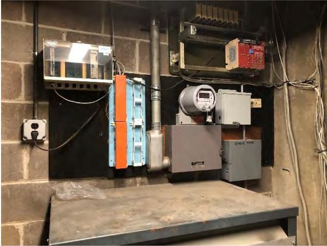
Figure E5: Utility Meter Located Above Existing Transformer in Main Electrical Room in 1953 Building
