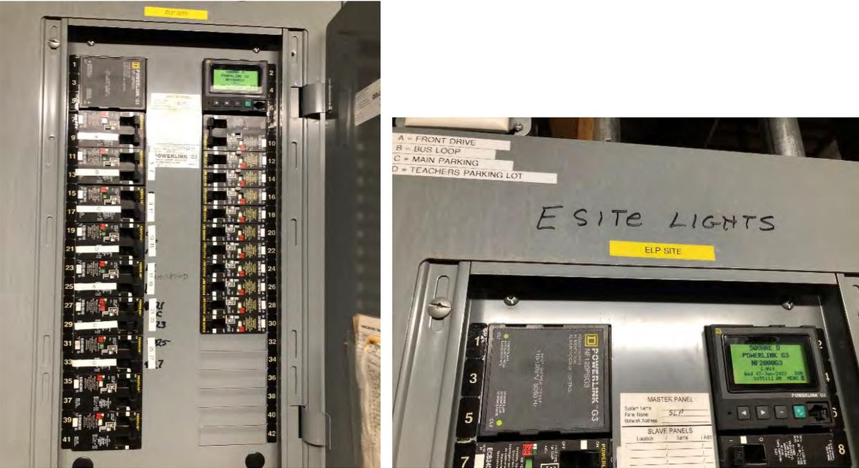
Figure E19: Exterior Site Lighting Control Panel
