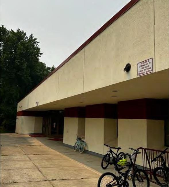
Figure P10: Storm Secondary Downspout Nozzle
