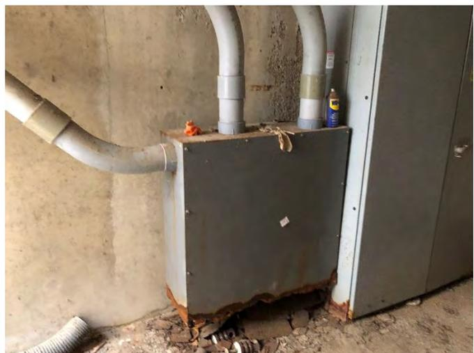
Figure E3: Main Service Entrance Rated Disconnect Switch and Pull Box
