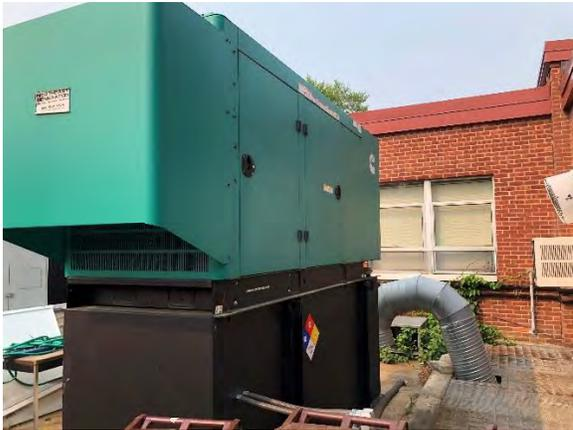
Figure E10: Exterior Site-Mounted Standby Power Generator
