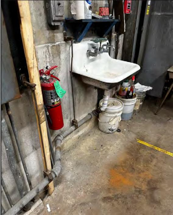
Figure P8: Basement Sink with Piping Drained into Waste Sump Pump
