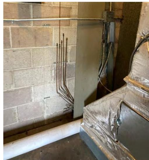
Figure M2: Pneumatic Controls (Left) and Abandoned Pneumatic Piping in Gym Penthouse (Right)
