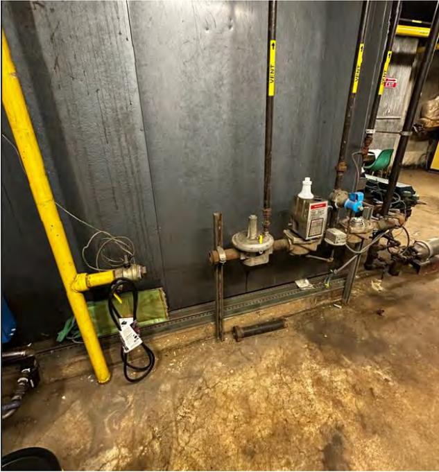
Figure P7: Gas Piping and Regulators Near Boilers
