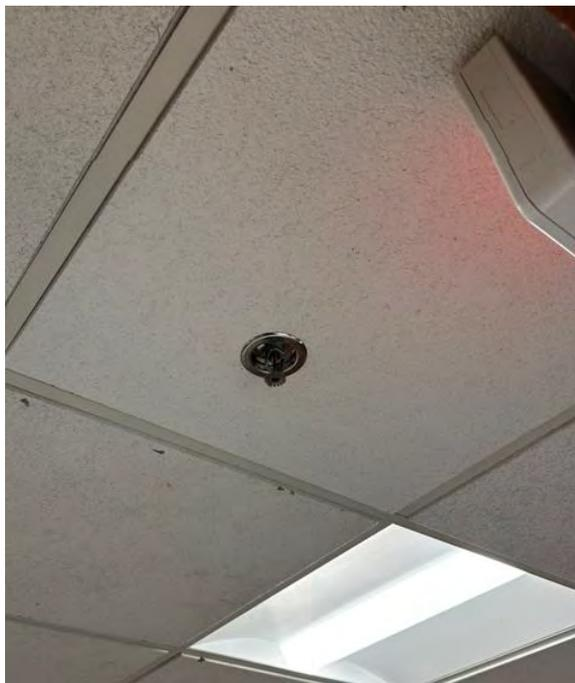
Figure FP3: Sprinkler Head Fed From Domestic Water System
