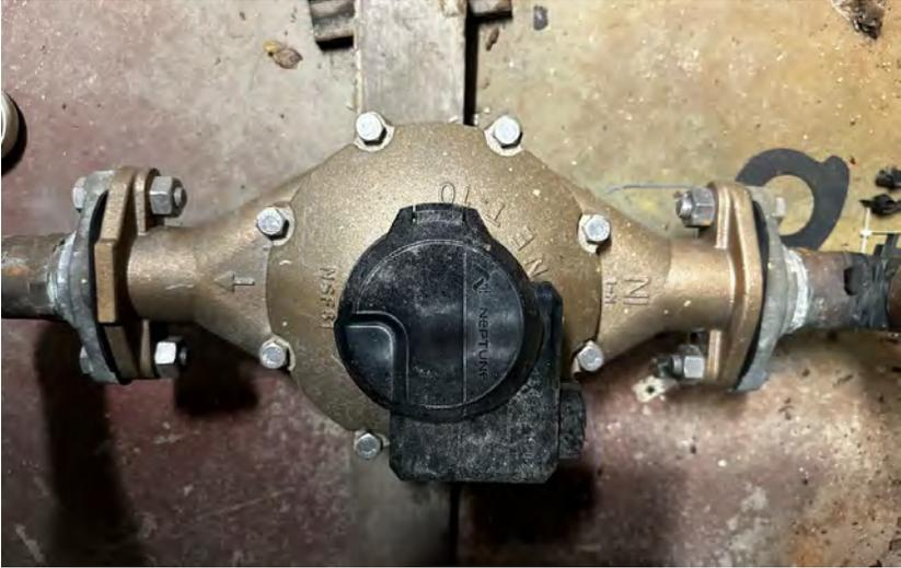
Figure P3: Domestic Water Meter
