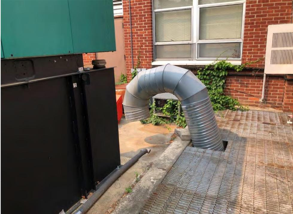
Figure M6: Combustion Air Duct Through Areaway Grating for Boilers
