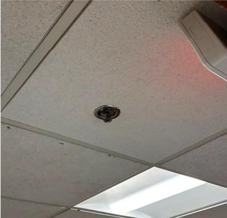
Figure FP3: Sprinkler Head Fed From Domestic Water System
