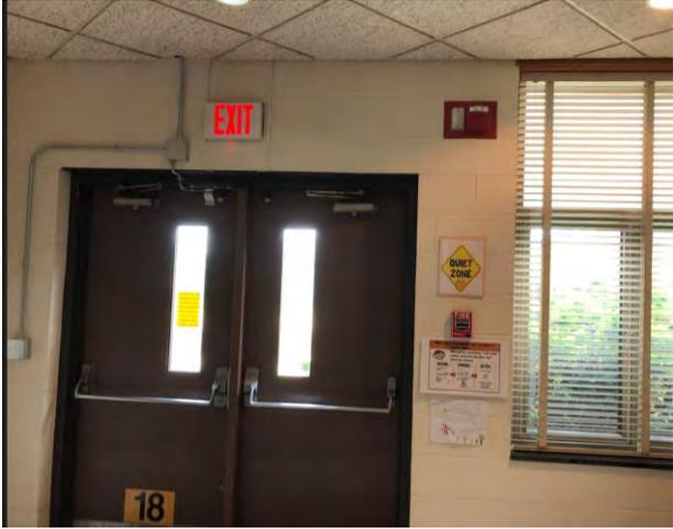
Figure E15: Fire Alarm System Horn/Strobe Unit
