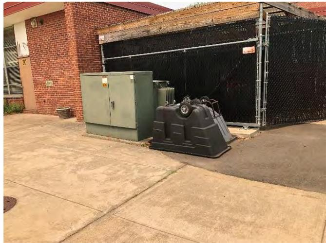
Figure E2: Pad-Mounted Utility Transformer
