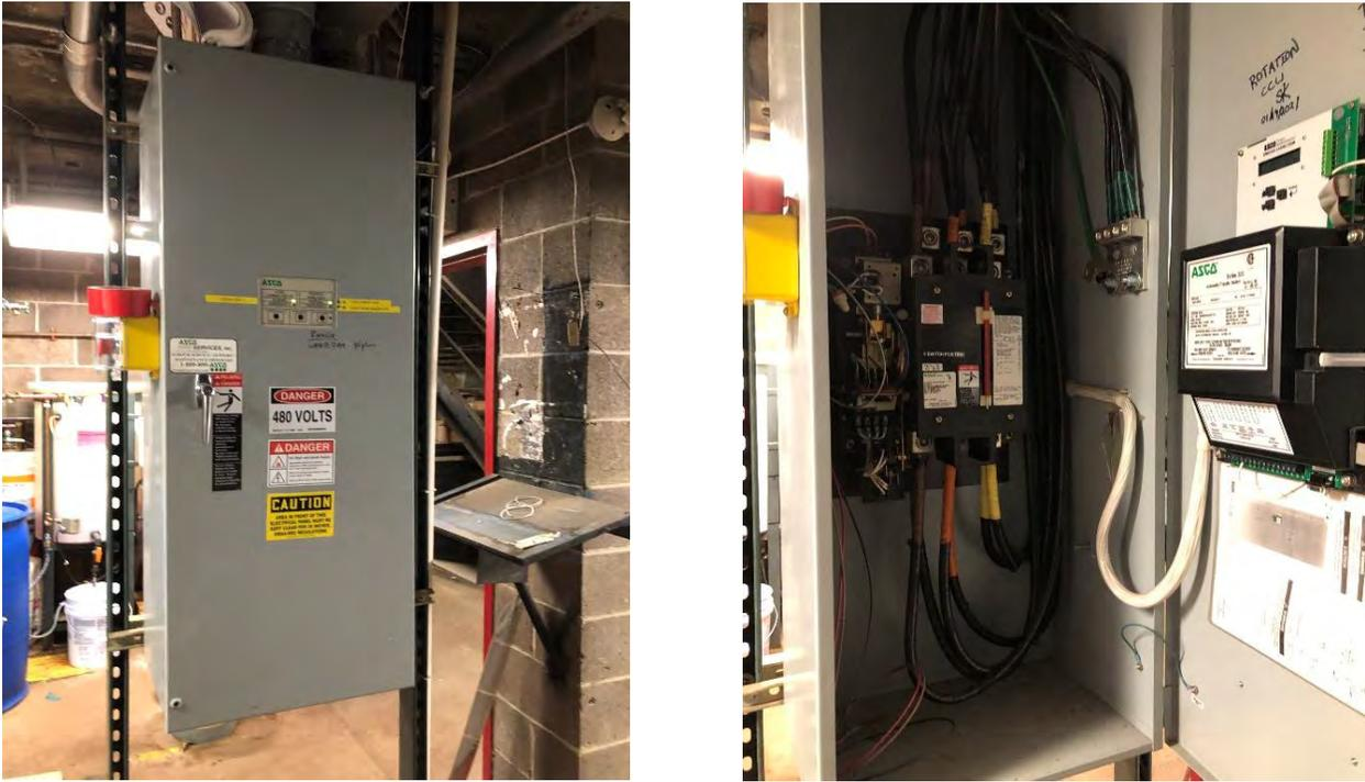
Figure E11: ASCO #300 Series Automatic Transfer Switch (ATS)
