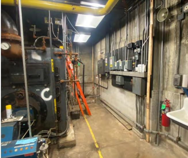
Figure E6: Electrical Panelboards and Electrical Equipment Located in Boiler Room
