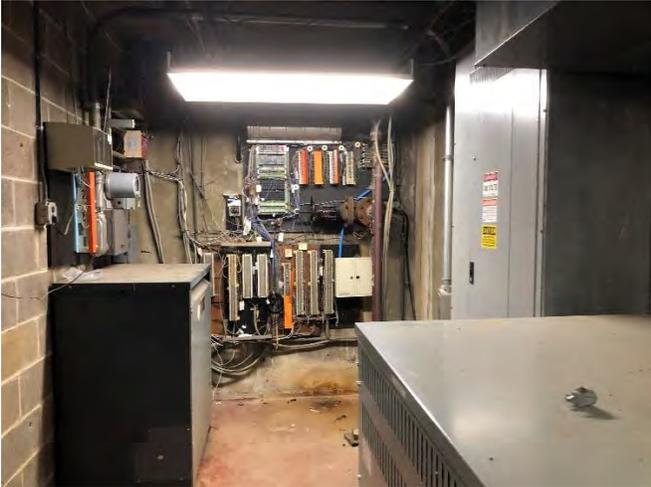
Figure E4: Main Electrical Distribution Panelboard HV-DP in Main Electrical Room in 1953 Building
