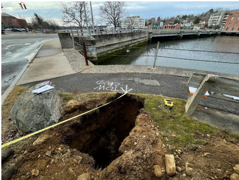
Photo 10: Test Pit TP-3, looking southwest from the walkway.
