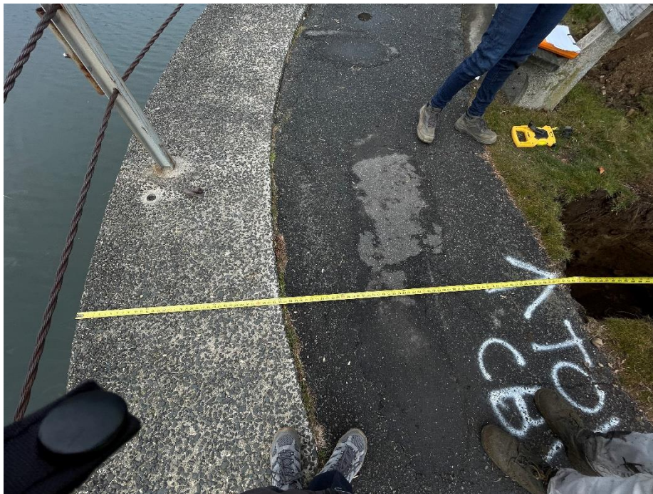
Photo 12: Test Pit TP-3, concrete seawall cap and asphalt walkway, looking northwest
