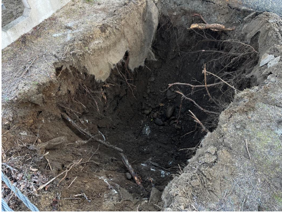
Photo 1: Test Pit TP-1, looking northeast from the seawall.
