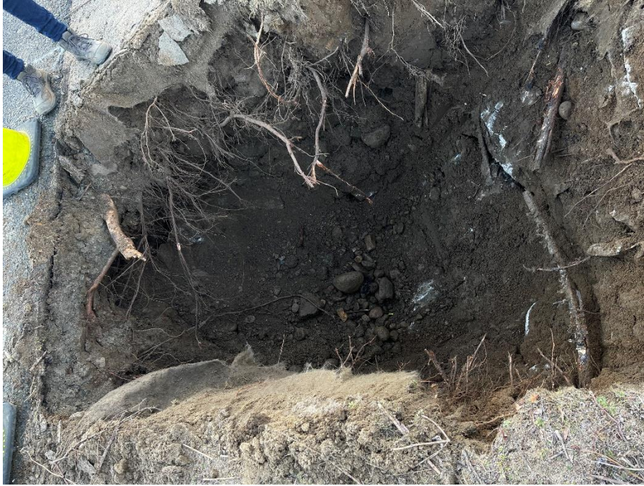
Photo 5: Test Pit TP-1, looking east.
