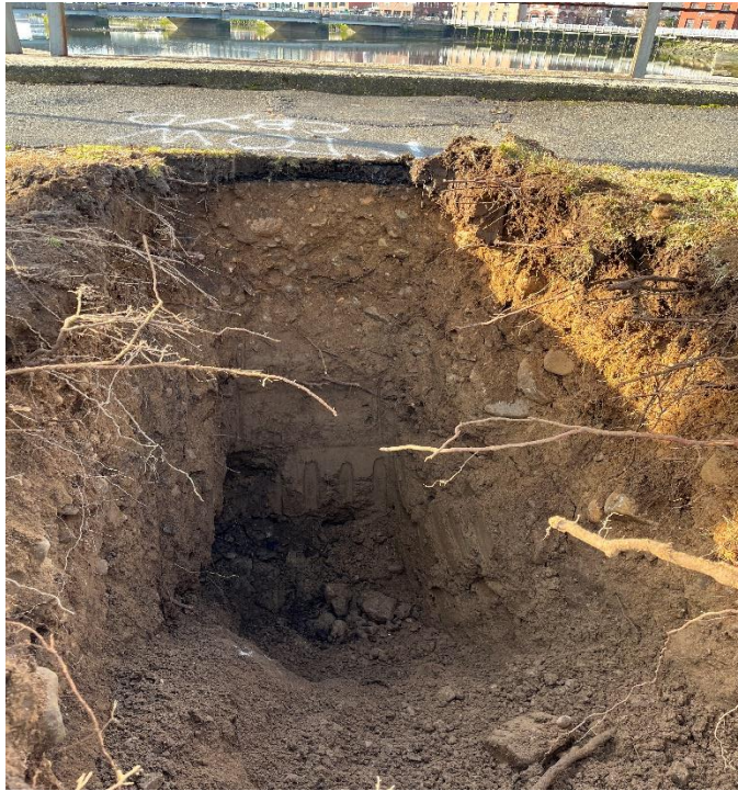
Photo 7: Test Pit TP-2, looking southwest toward the seawall.
