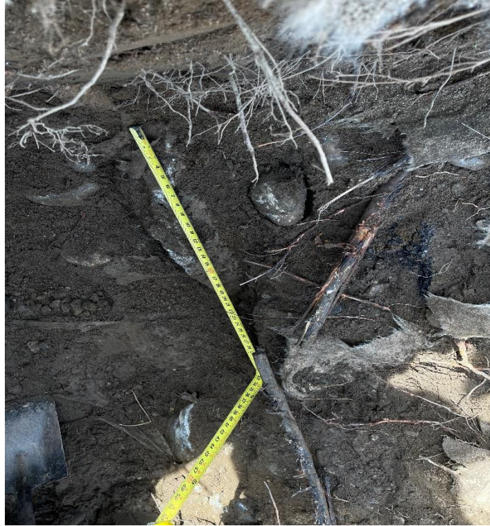
Photo 3: Test Pit TP-1, looking southwest toward the back of the seawall.
