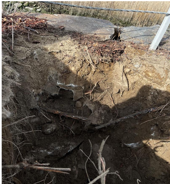
Photo 2: Test Pit TP-1, looking southwest toward the back of the seawall.
