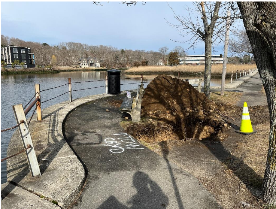
Photo 6: Test Pit TP-2, looking northwest from the walkway.
