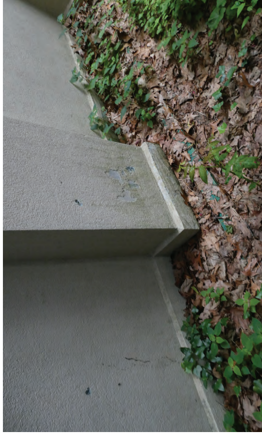
SOME EFIS PATCHING AND PAINTING NEEDED.
