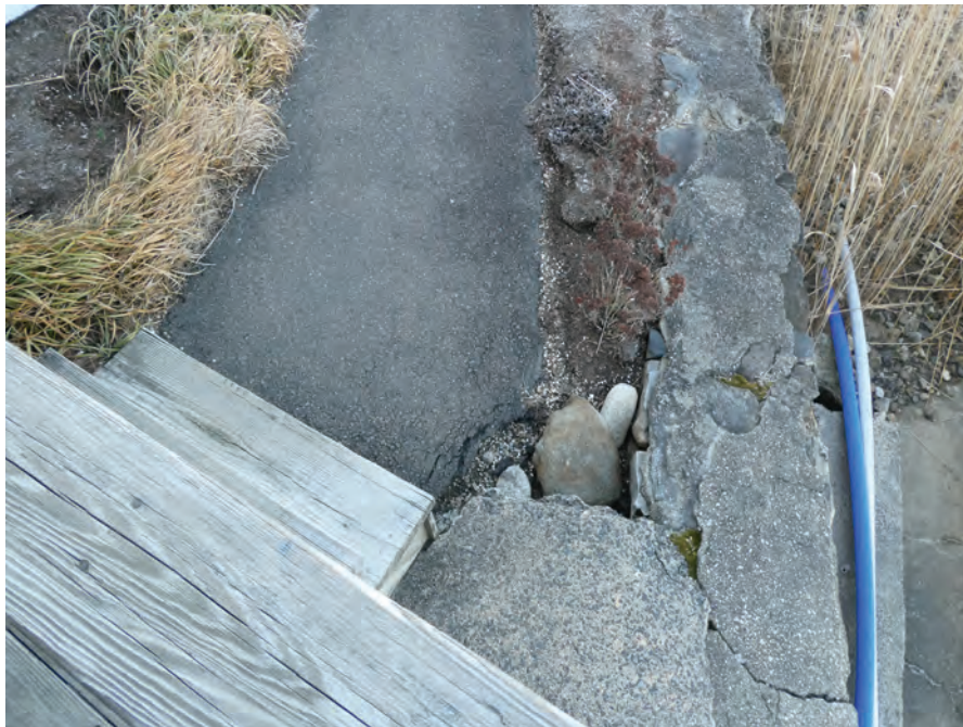
STEP/WALL NON UNIFORM LANDING AREA
