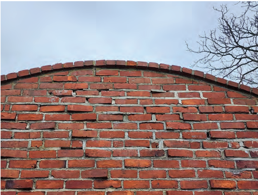
FAILING REPOINTING
