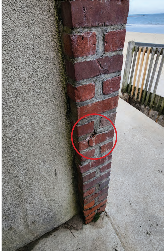
SPALLING BRICK
