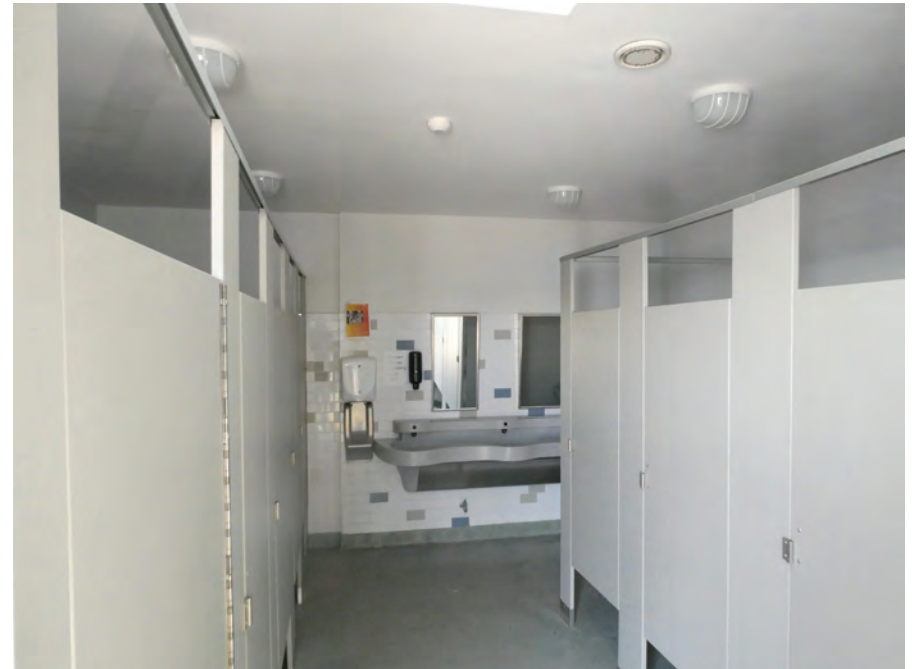
REHABILITATED MEN'S AND WOMENS ROOMS - NORTH END
