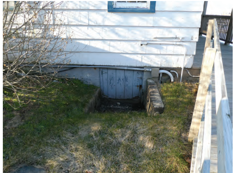
REPLACE CRAWL SPACE DOOR.
