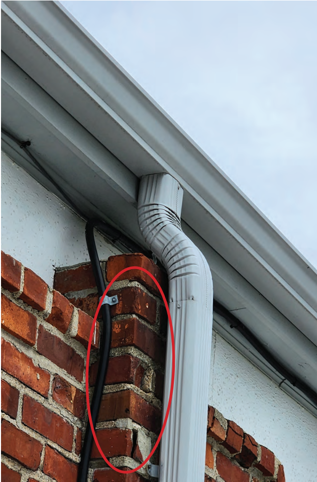
REPOINTING AT COLUMN CAP
