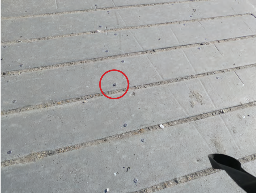
SHARP EDGES SCREWS
