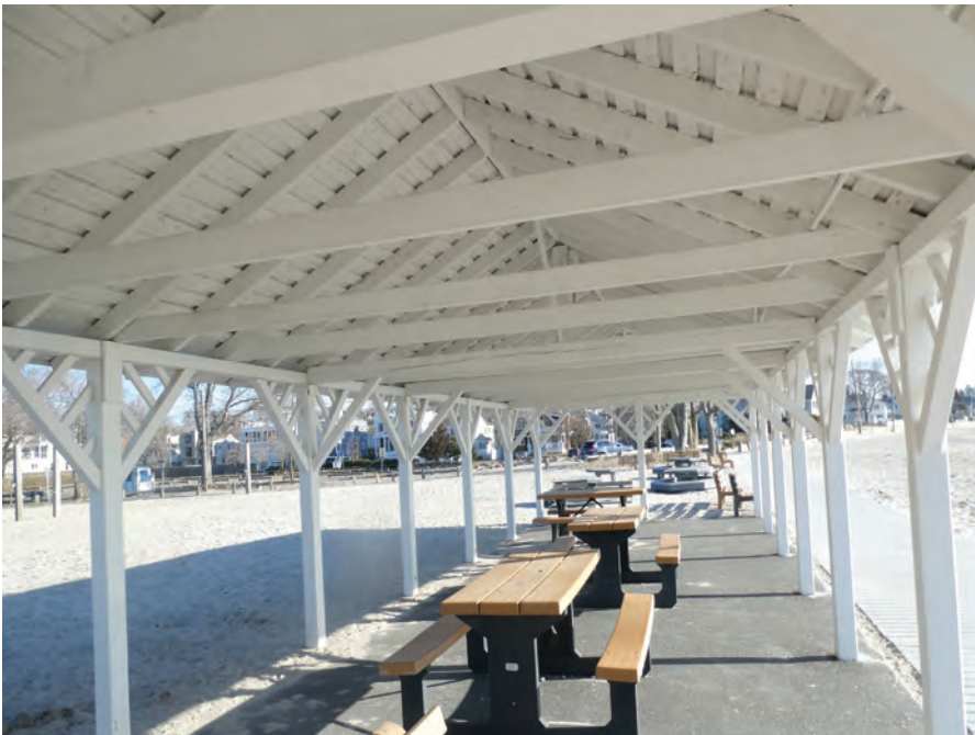
FIX SOME BEAMS
