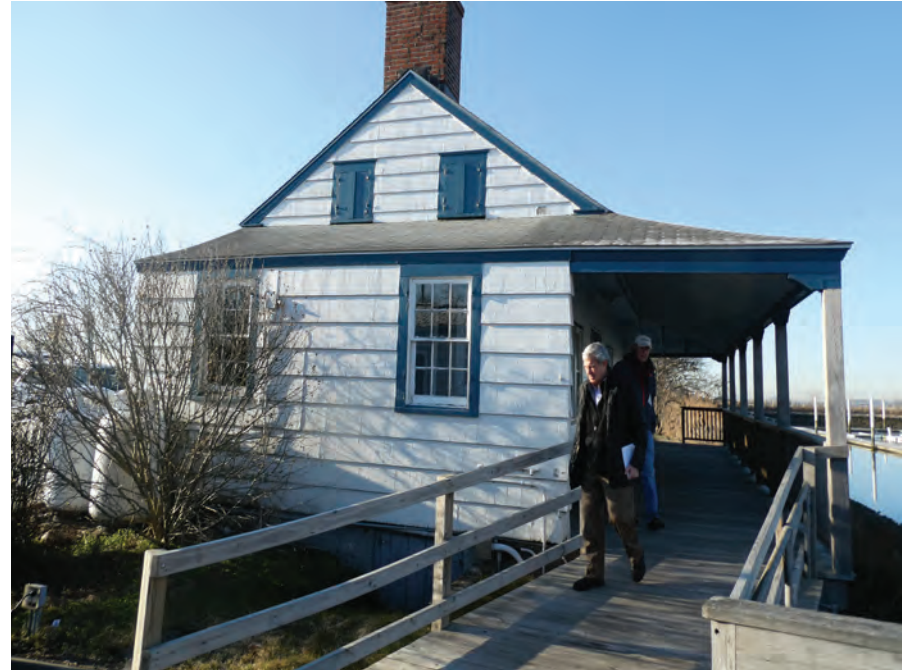
OVERALL NORTH ELEVATION SATISFACTORY.
