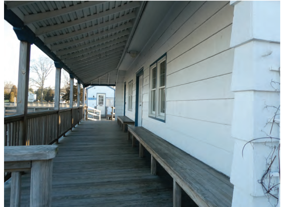
DECK SATISFACTORY - POWERWASH AND STAIN
