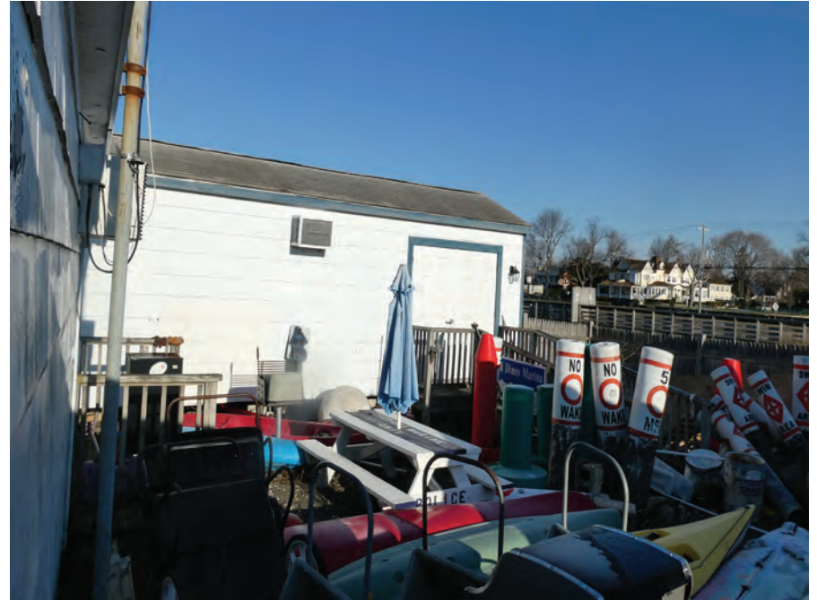
COURTYARD STORAGE AREA - ROOF REQUIRED.
