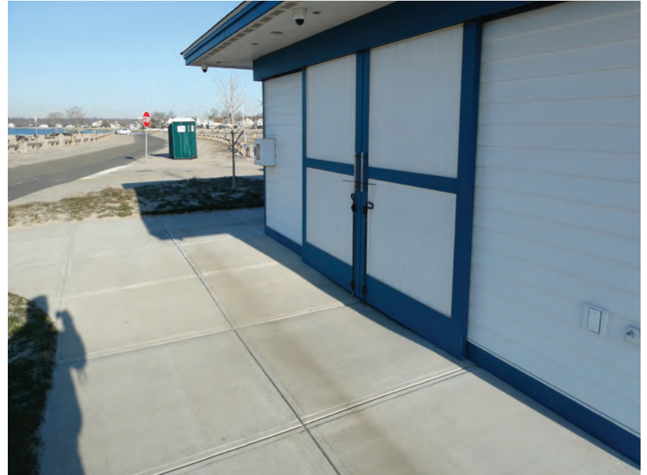
CONCRETE PAVING - GOOD SHAPE
