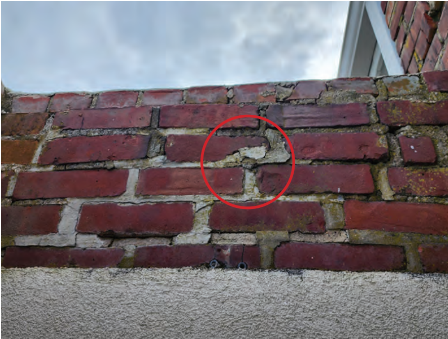
SPALLING POINTING
