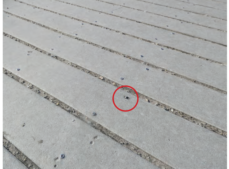
SHARP EDGES SCREWS
