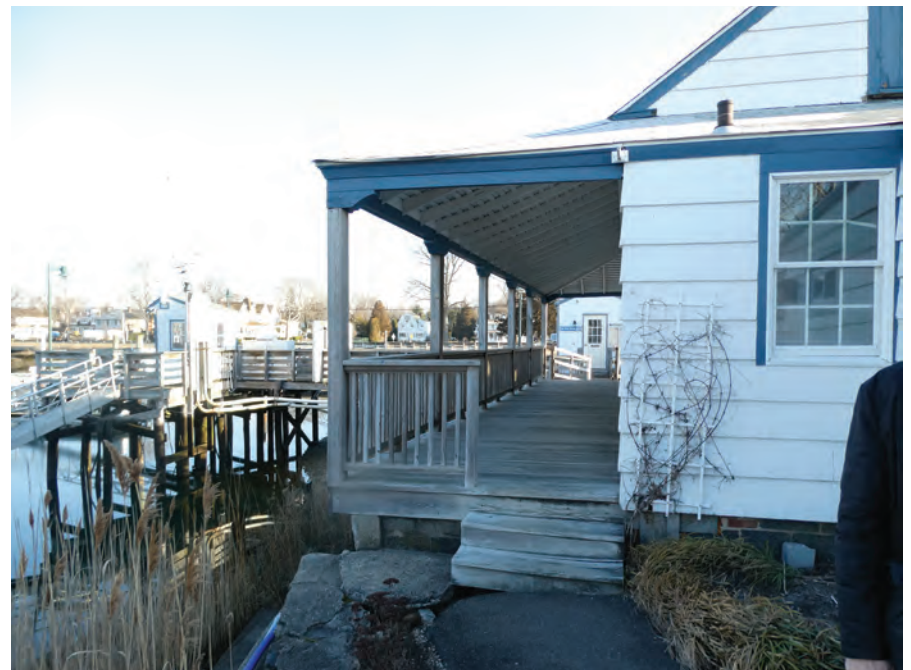
STEPS PORCH TO GRADE REBUILD WITH HANDRAIL.
