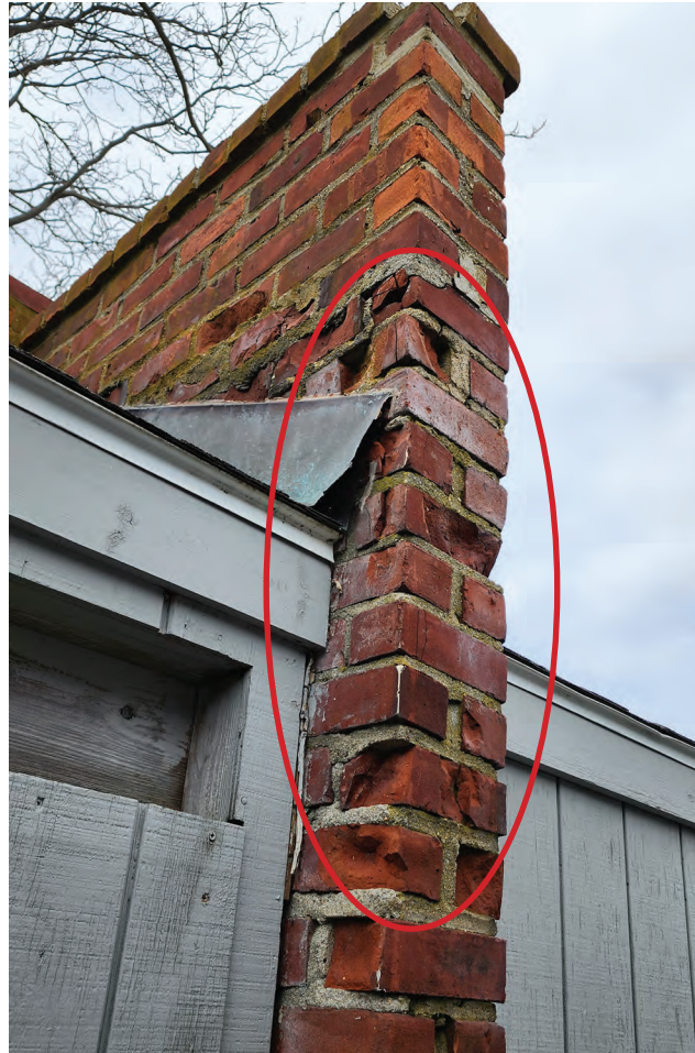
SPALLED BRICK
