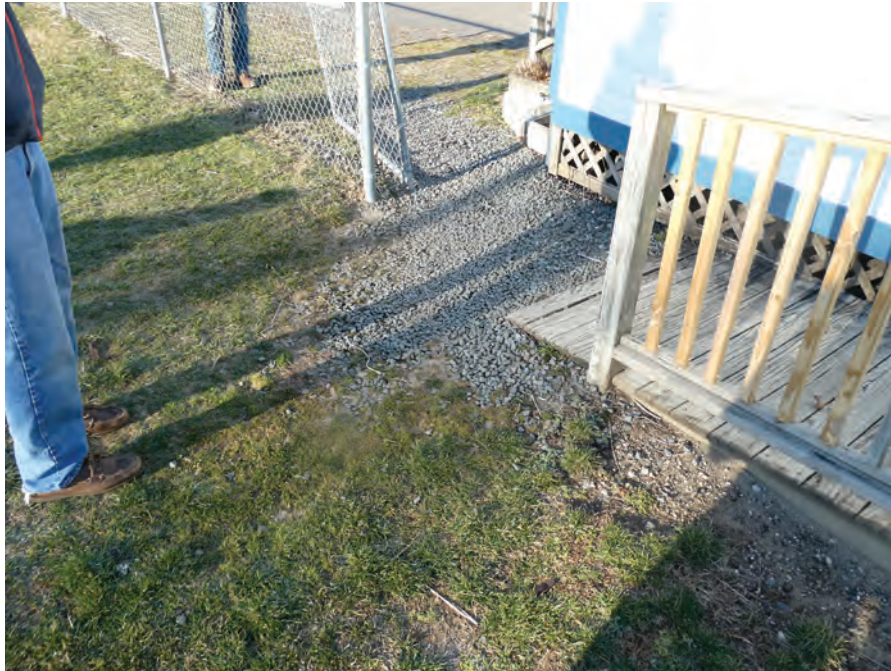
GRAVEL AREA SHOULD BE PAVED.
