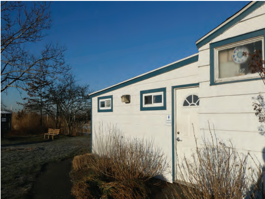
NEWER RESTROOM DOORS
