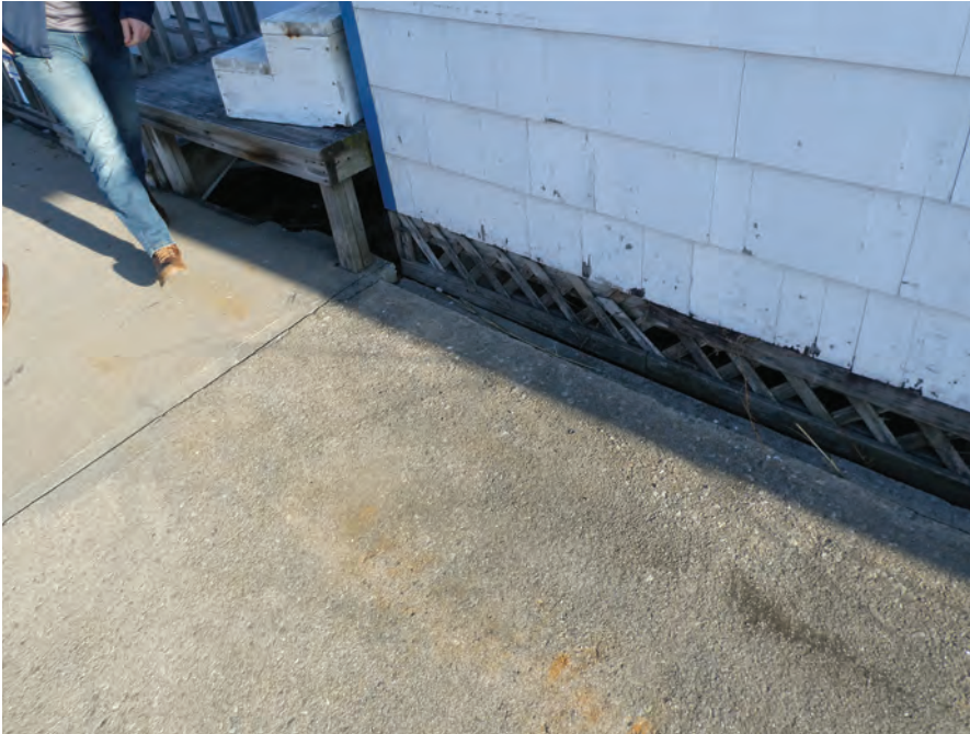
REPAIR SIDING AND PAINT.
