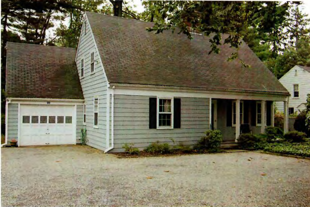
View of the west elevation.
