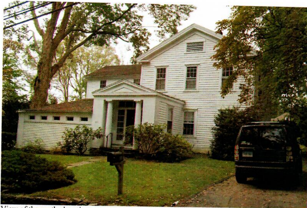
View of the north elevation.
