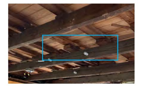
Ceiling joists supporting second floor are woefully undersized for span and are failing.
