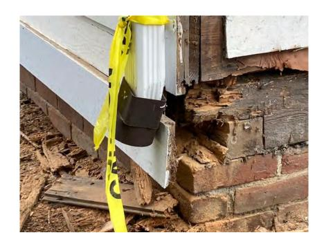
Sill plate on top of that foundation is rotted through.
