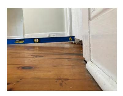
Primary load bearing wall on first floor is 2 inches down and continuing to sink.
