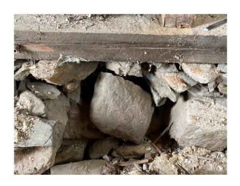
Rubble foundation under rear of house is collapsing (inside view)
