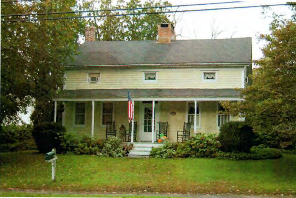
View of the east elevation.
