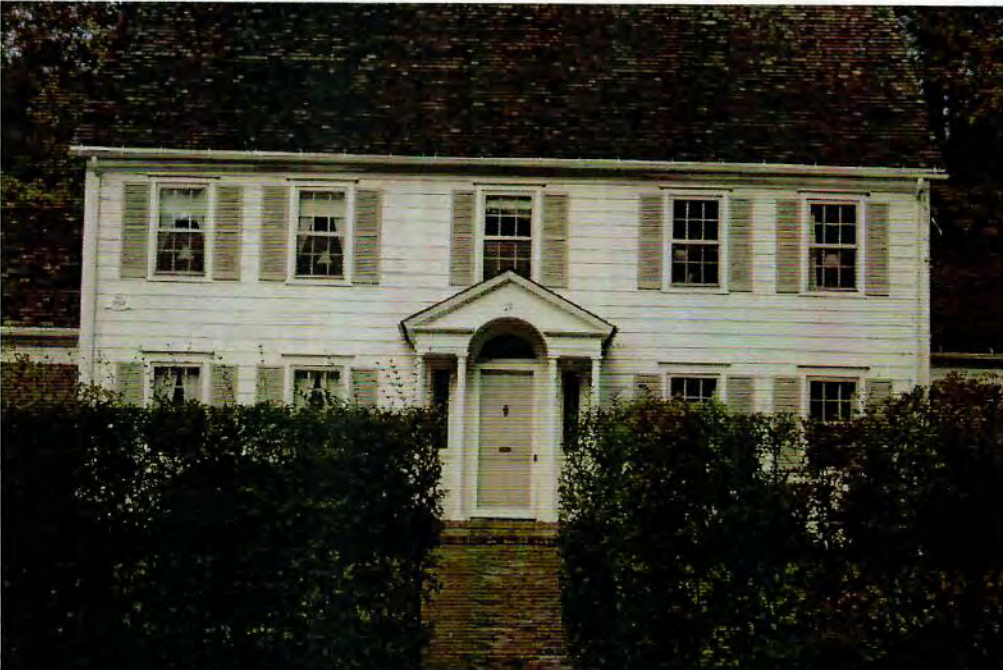
View of the east elevation.
