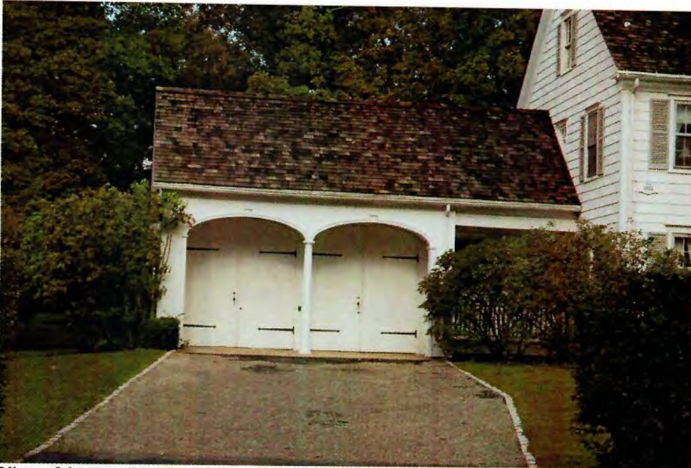
View of the east elevation of the attached garage.
