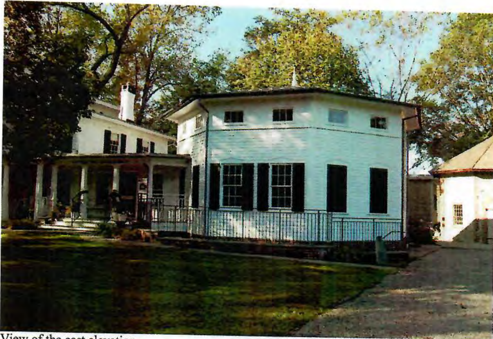
View of the east elevation.
