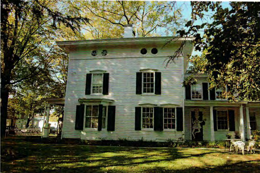
View of the east elevation.
