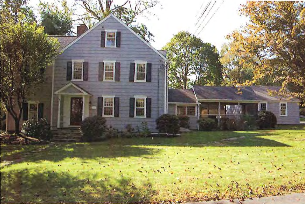
View of the north elevation.
