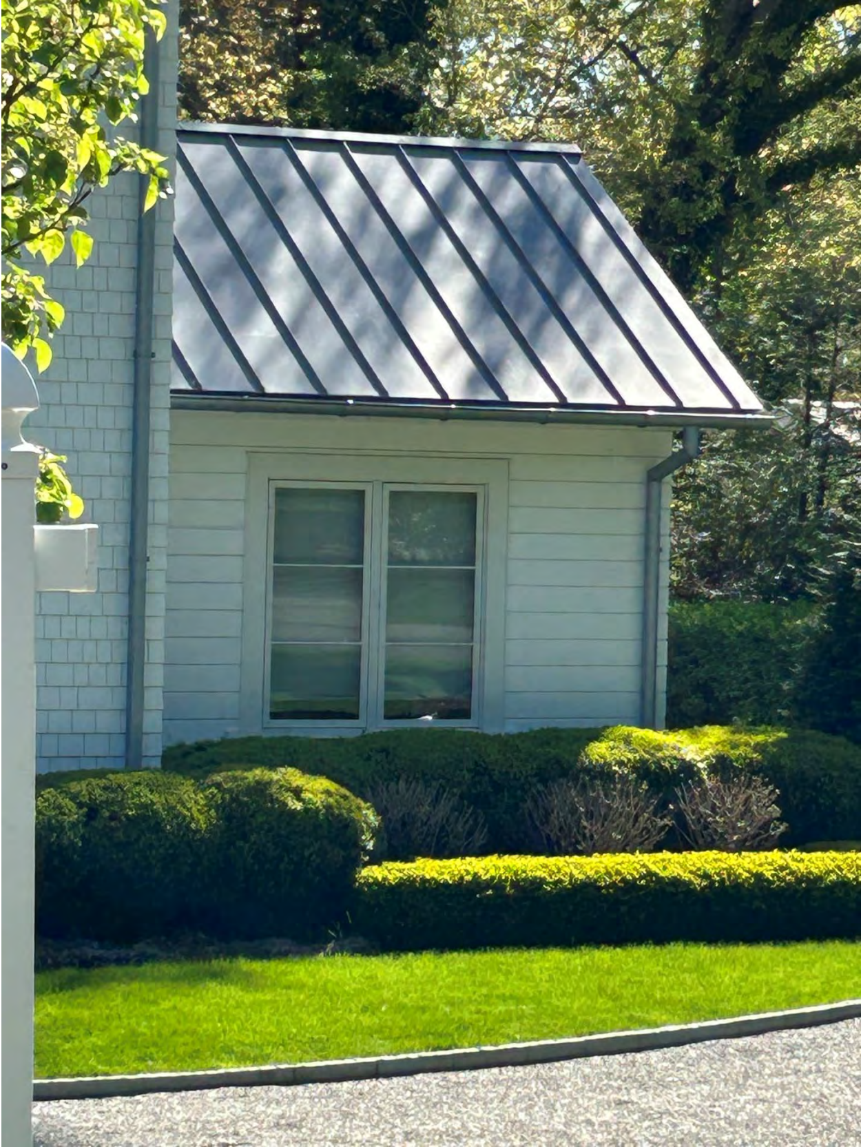
Roofing of seam metal roof in a charcoal grey.
