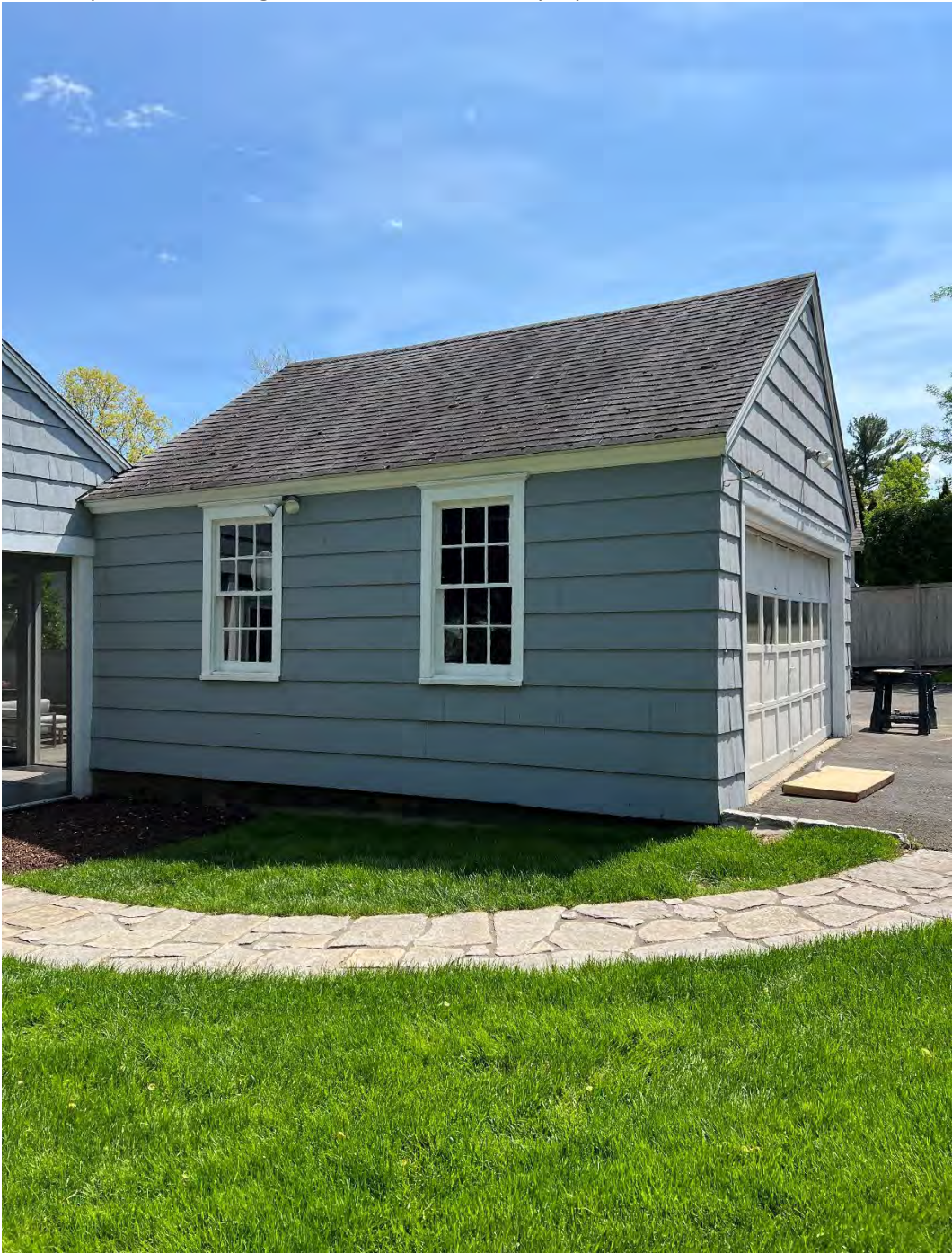
Current photo of existing elevation where work is proposed.
