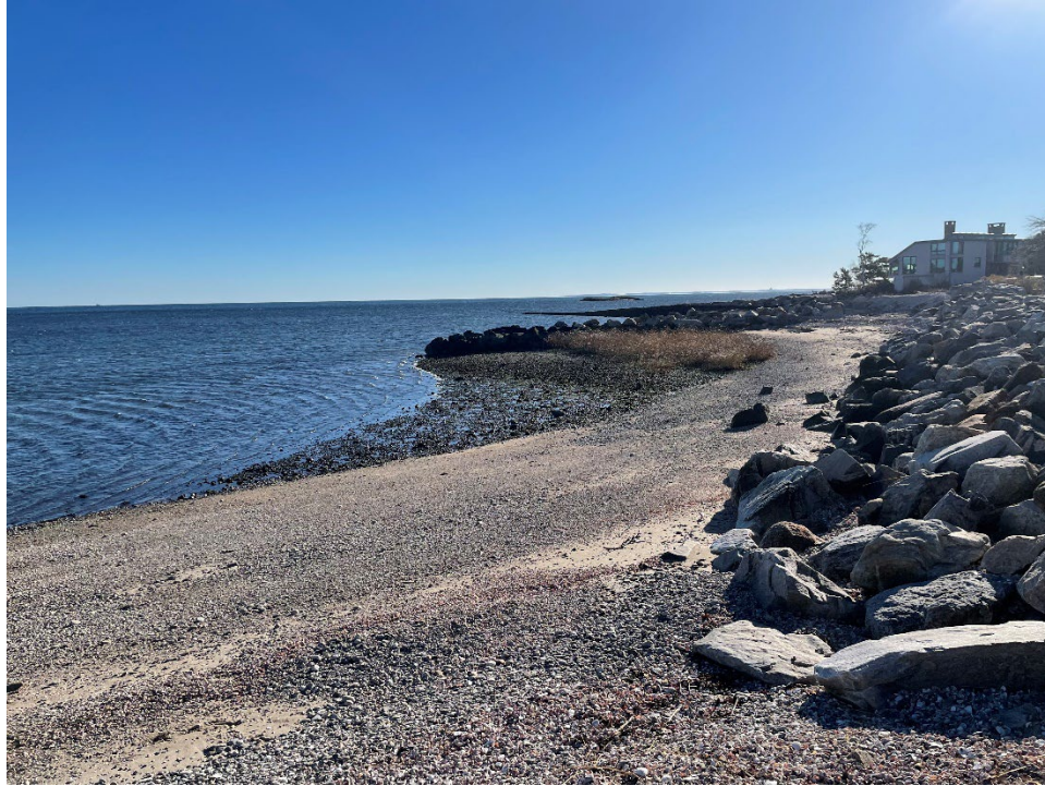
Figure 5: East Beach looking southeast
