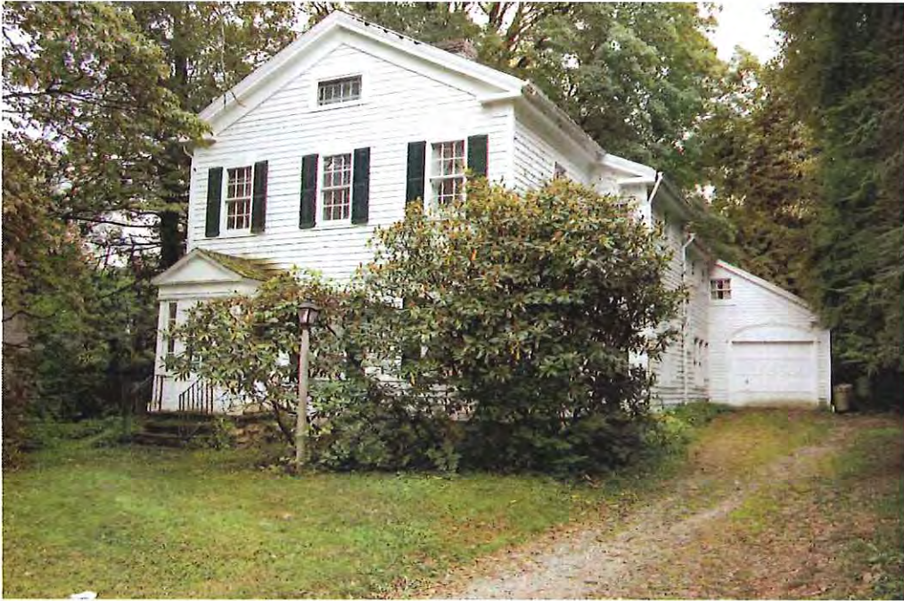
View of the north elevation.
