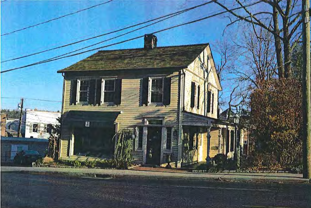
View of the west and south elevations.
