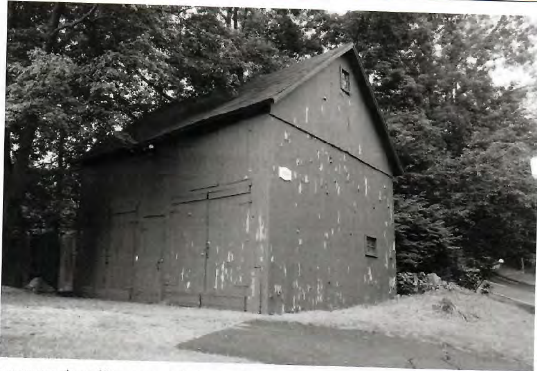
7. Southeast corner view of Barn, camera facing northwest.
