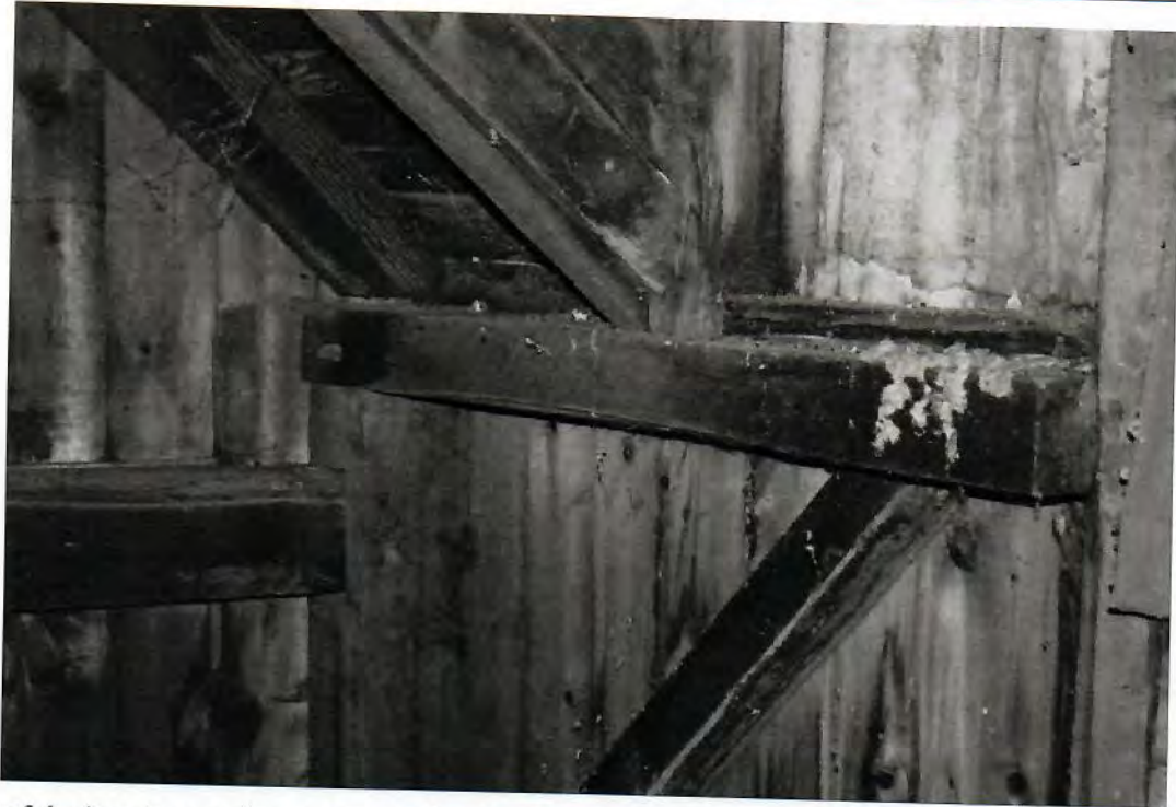
15. Detail of the interior, northwest corner, showing dropped tie-girt in end wall. Note how the rafter plate is truncated for the shed dormer.
