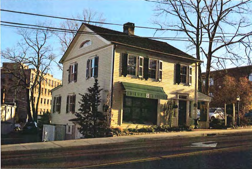
View of the north and west elevations.
