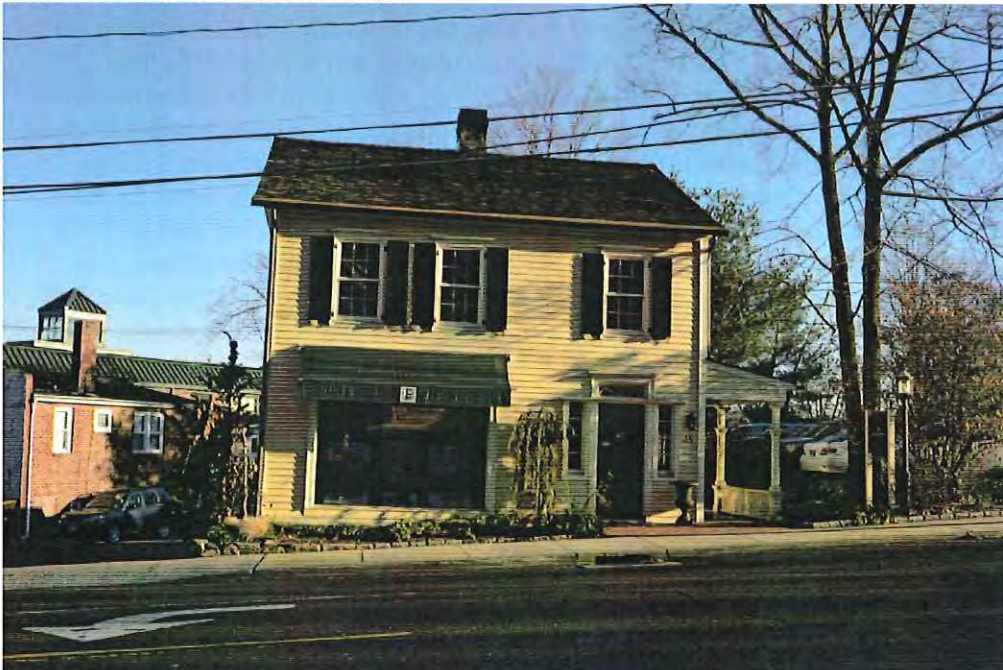
View of the west elevation.
