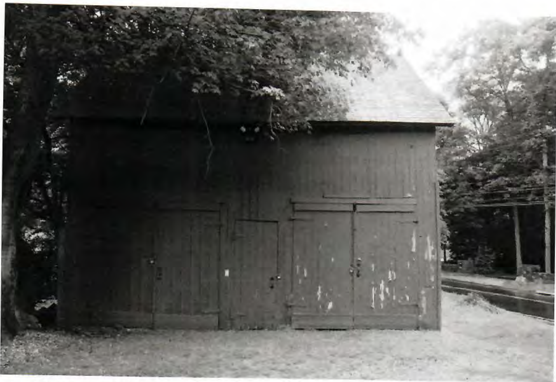
6. South view of Barn, camera facing north.
