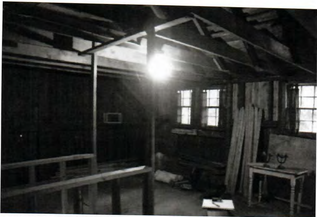
14. Attic level of barn, camera facing northwest.
