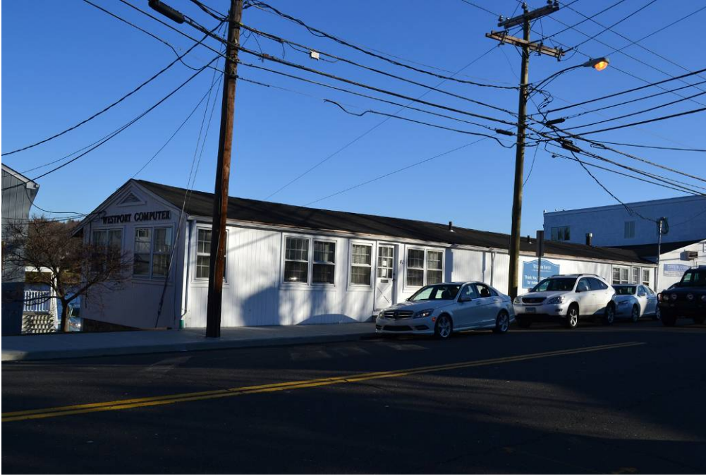
View of the north and west elevations.
