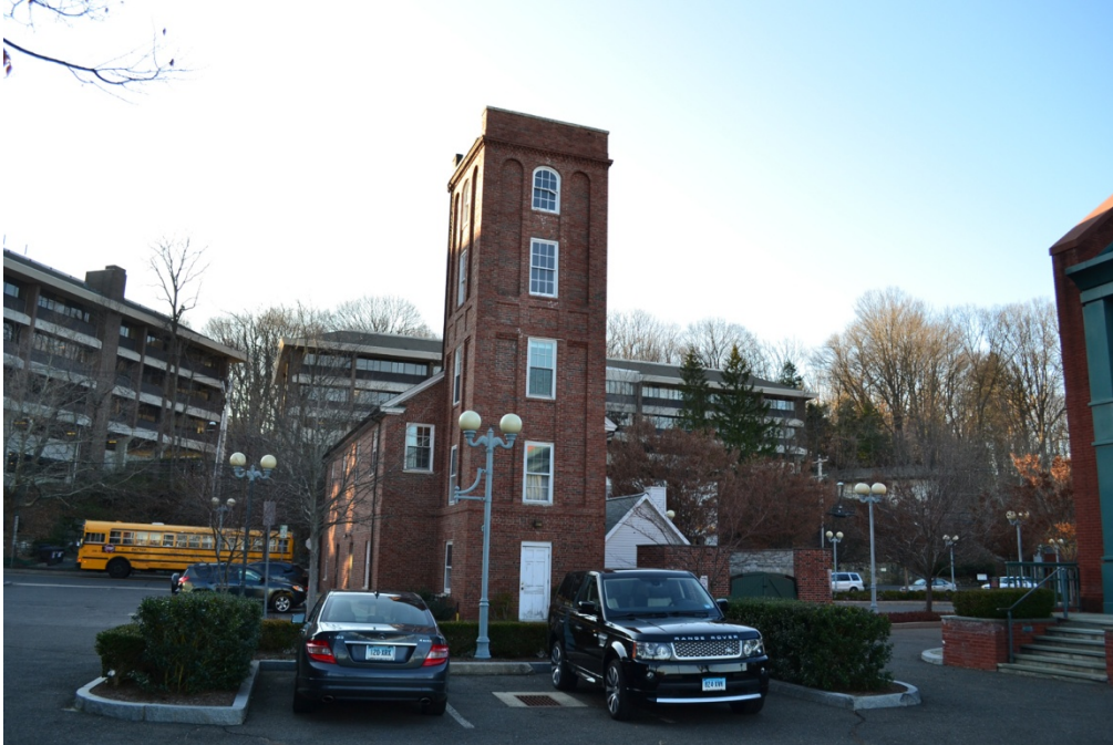
View of the east elevation.
