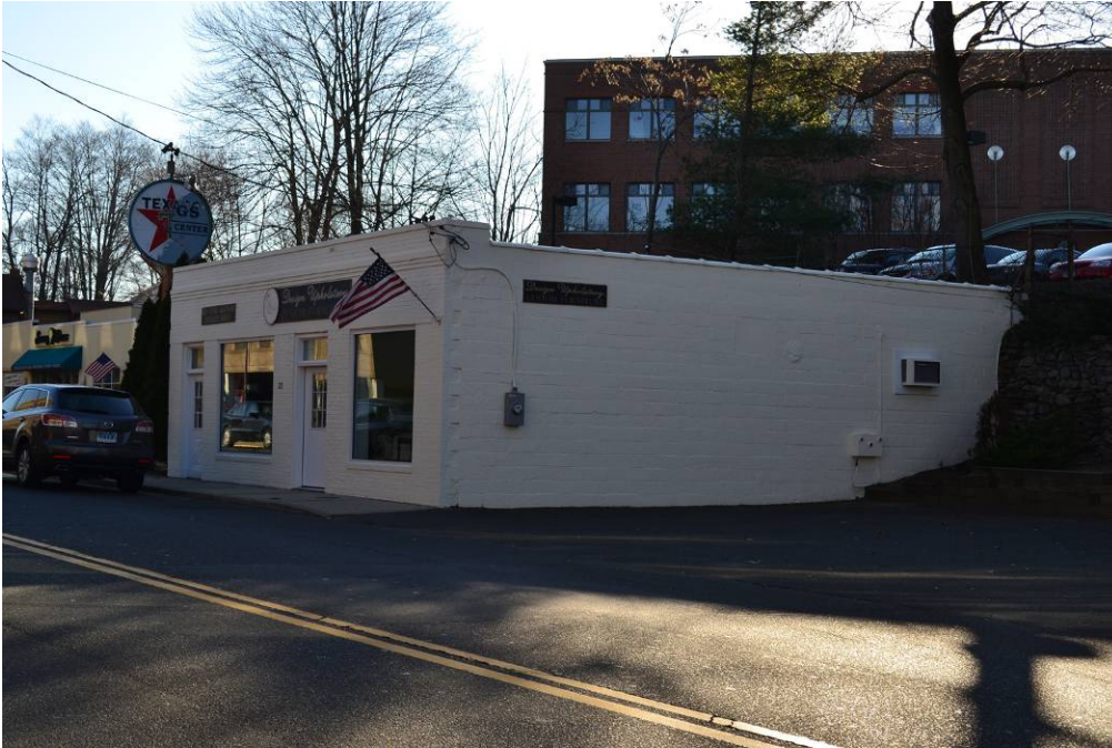
View of the north and east elevations.
