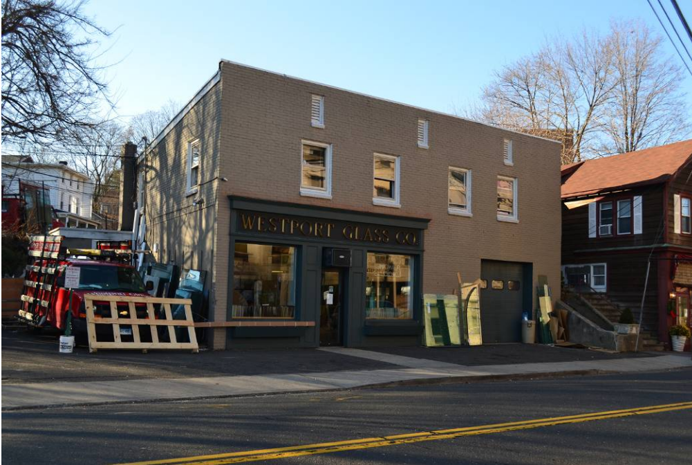
View of the east and south elevations.
