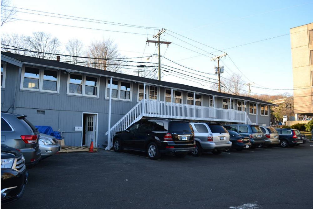
View of the east elevations.
