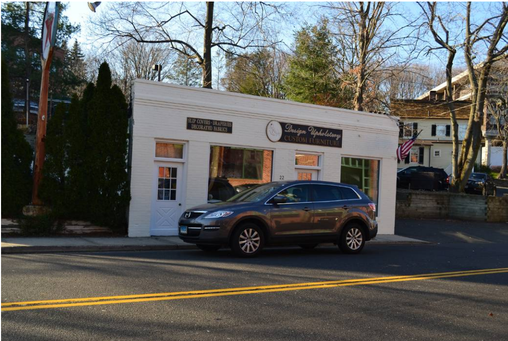
View of the east elevation.
