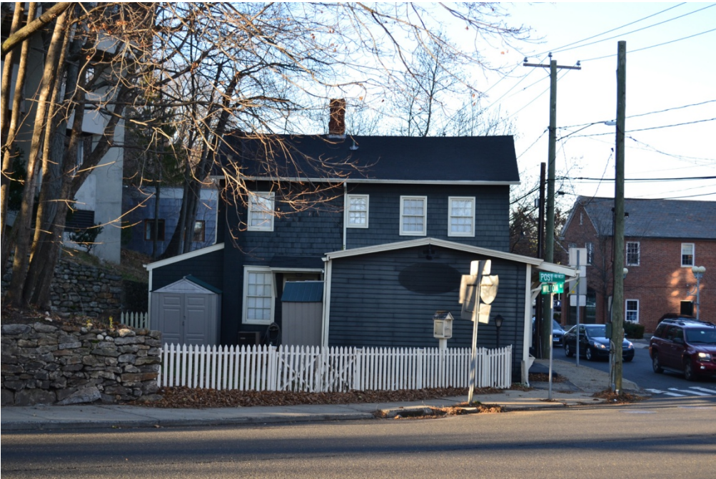
View of the south elevation.
