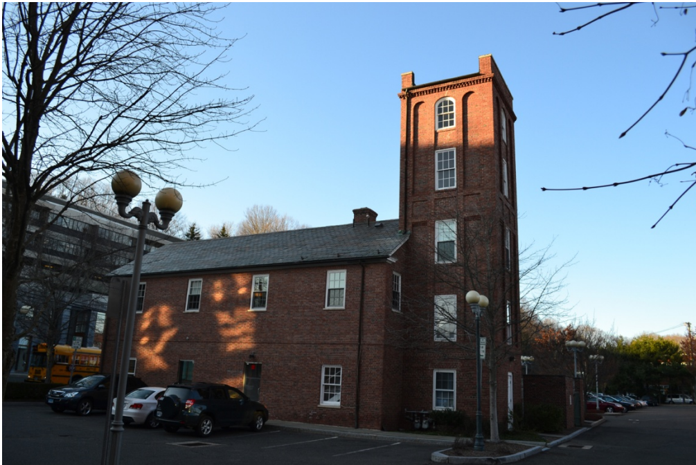
View of the north and east elevations.
