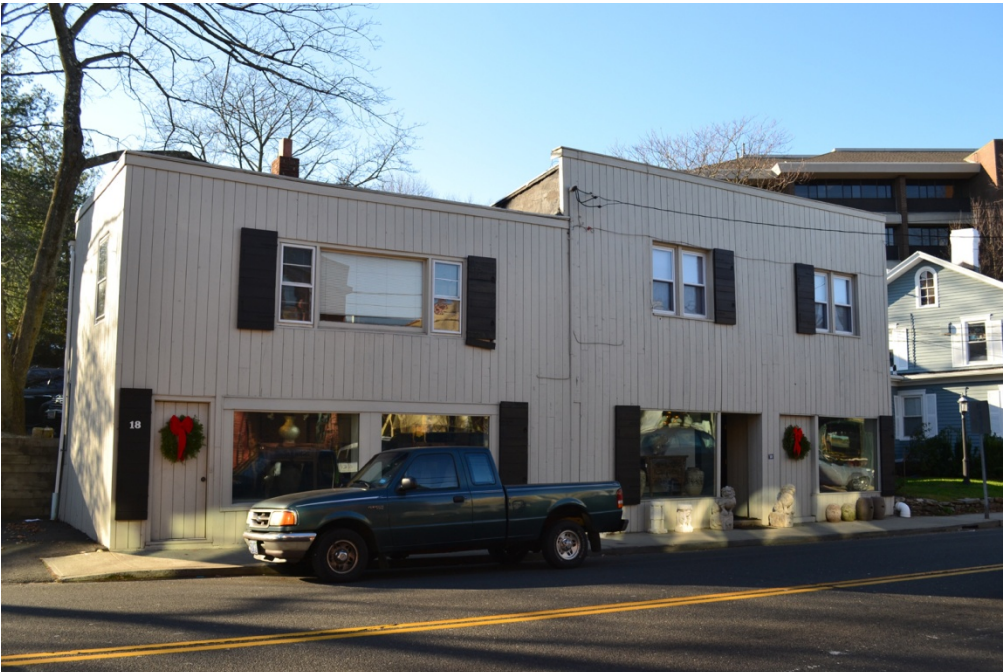
View of the east and south elevations.
