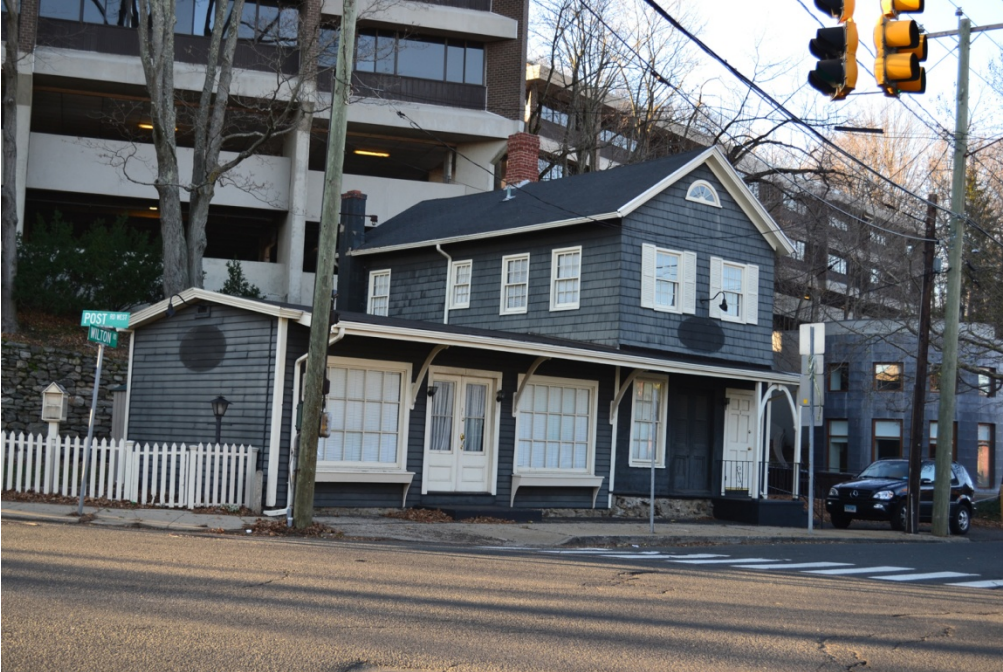
View of the south and east elevations.
