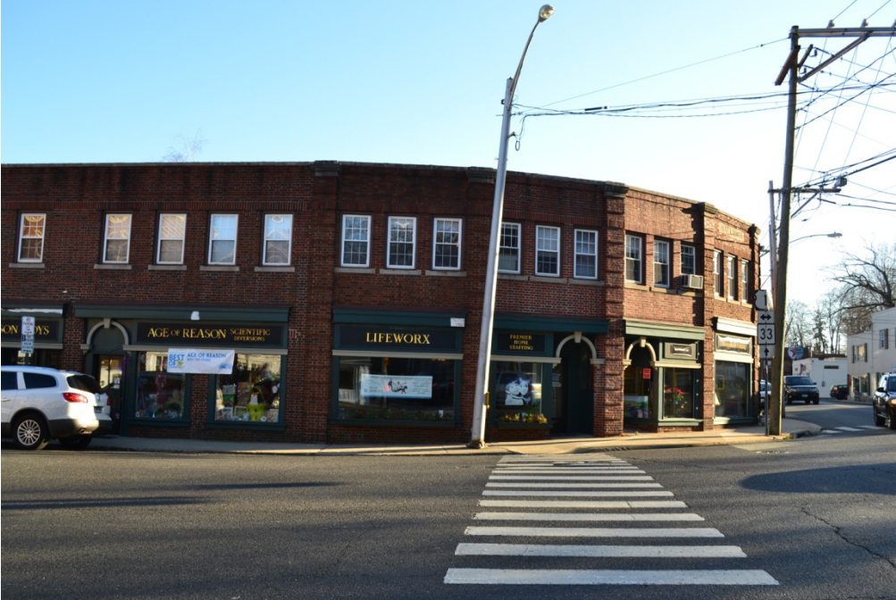
View of the northwest elevation.
