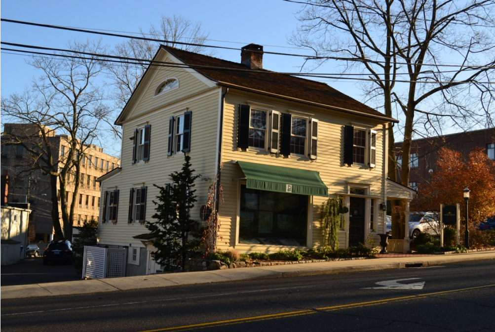
View of the north and west elevations.
