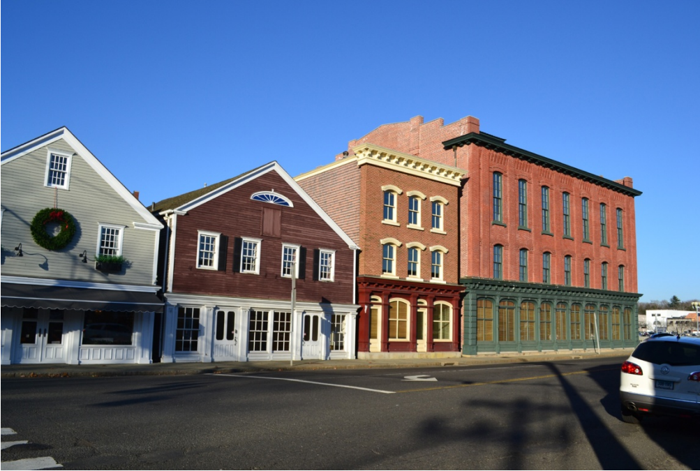
View of the south elevation.
