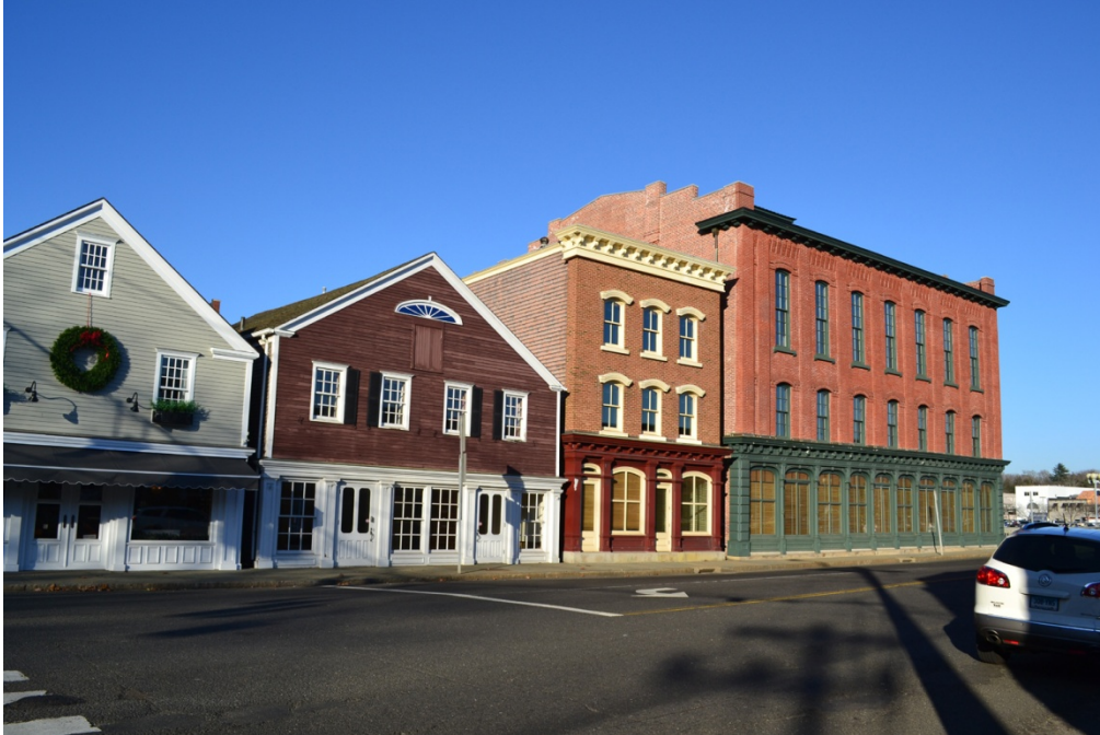
View of the south elevation.
