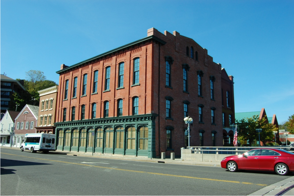
View of the south and east elevations.
