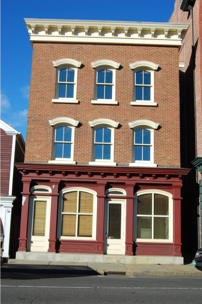
View of the south elevation.
