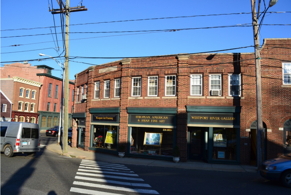
View of the southwest elevation.
