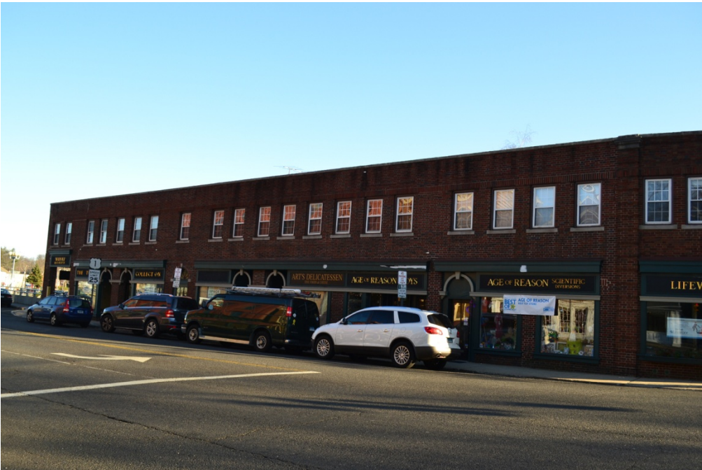
View of the north elevation.
