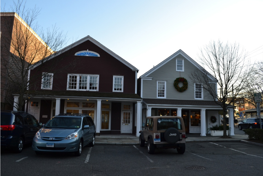
View of the north elevation.
