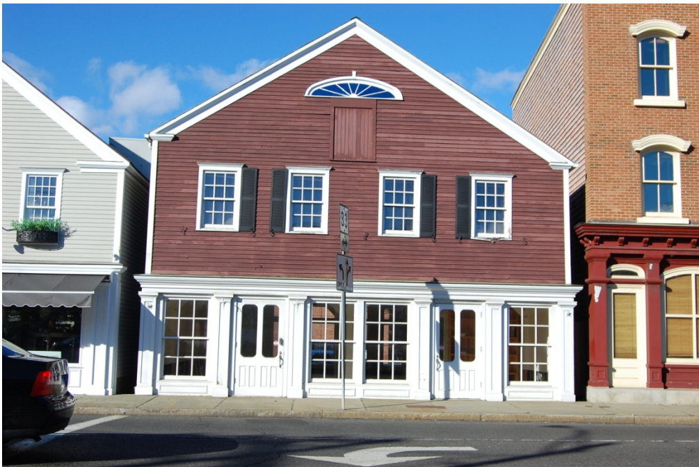
View of the south elevation.
