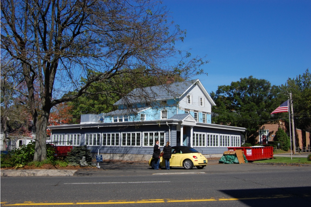
View of the west and south elevations.
