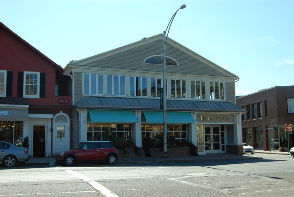
View of the north elevation.
