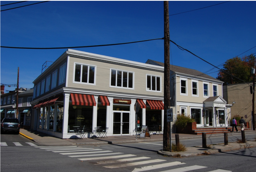
View of the south and west elevations.
