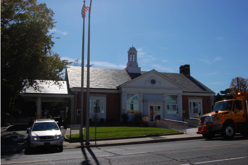
View of the north elevation.
