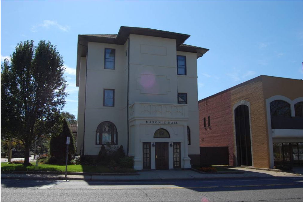
View of the north elevation.
