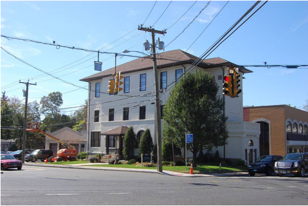
View of the north and east elevations.
