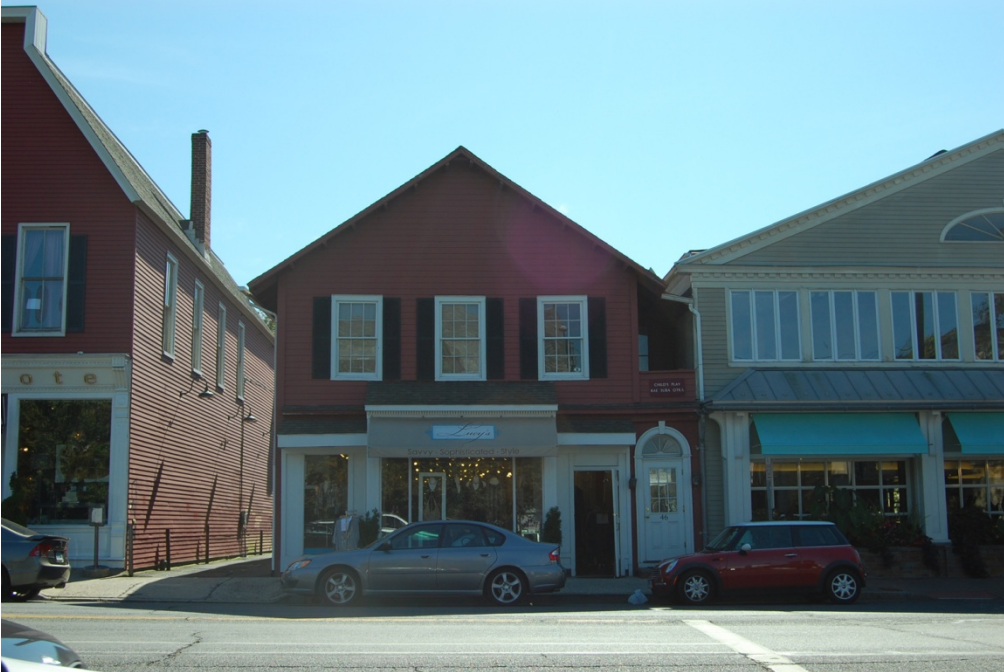
View of the north elevation.
