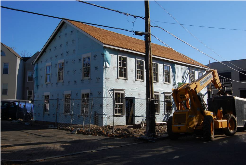
View of the northwest and northeast elevation (10/6/2011).
