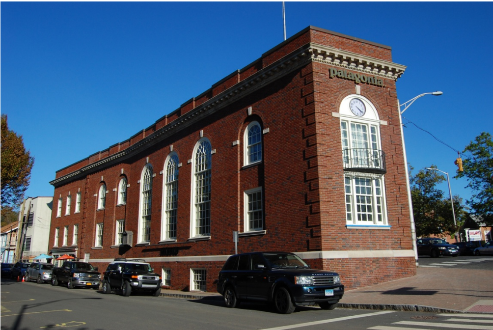
View of the north and east elevations.
