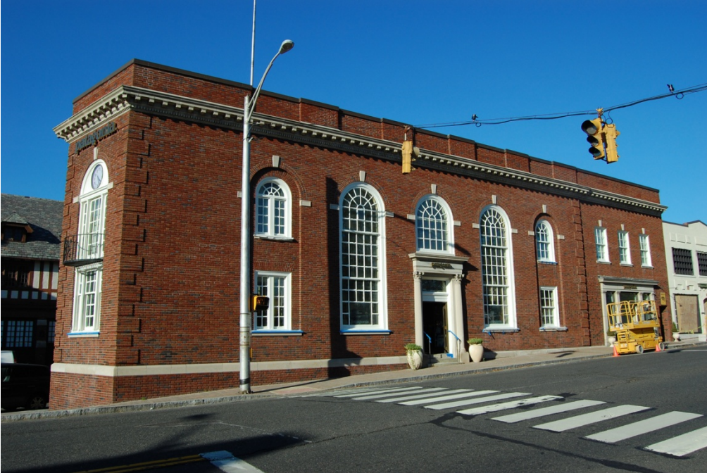
View of the west elevation.
