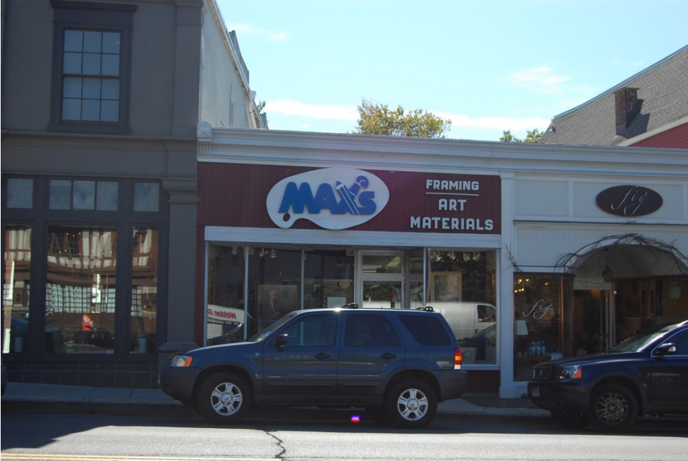
View of the north elevation.
