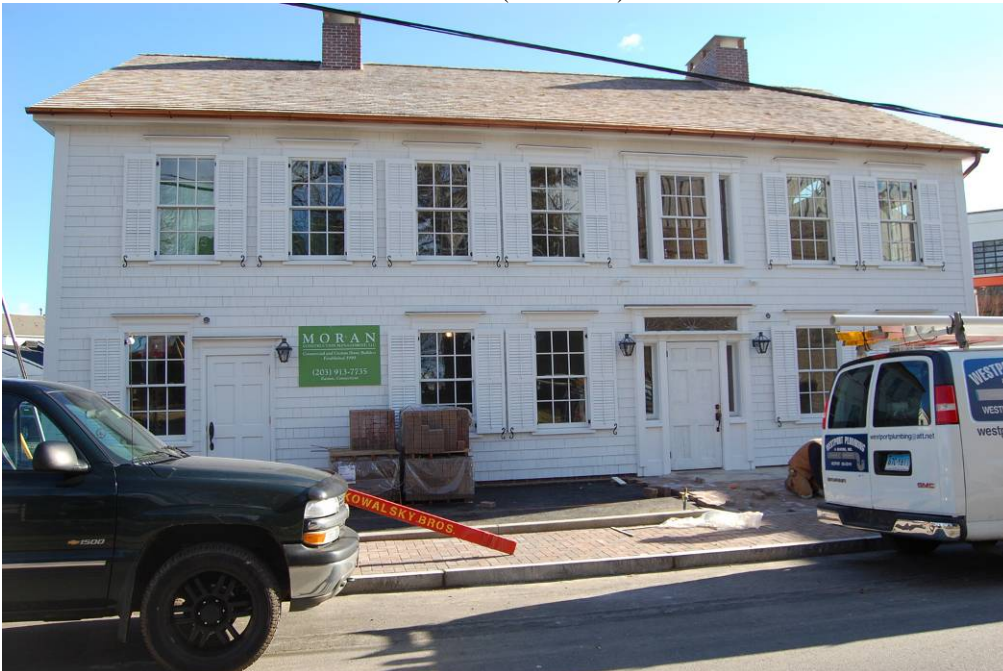
View of the northeast elevation (1/18/2012).
