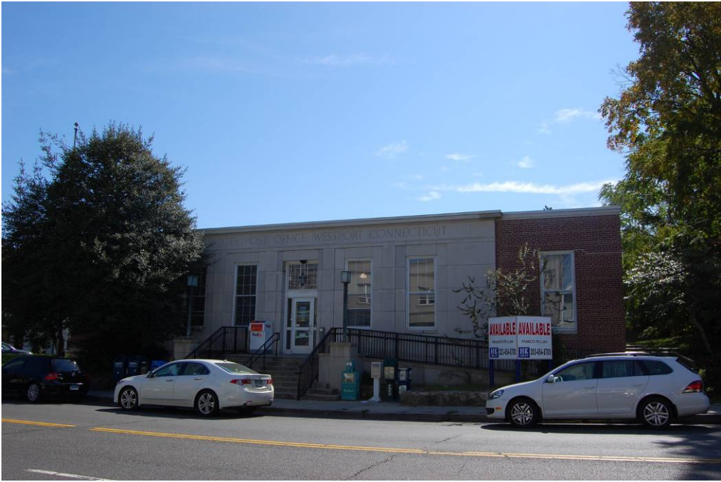
View of the north elevation.
