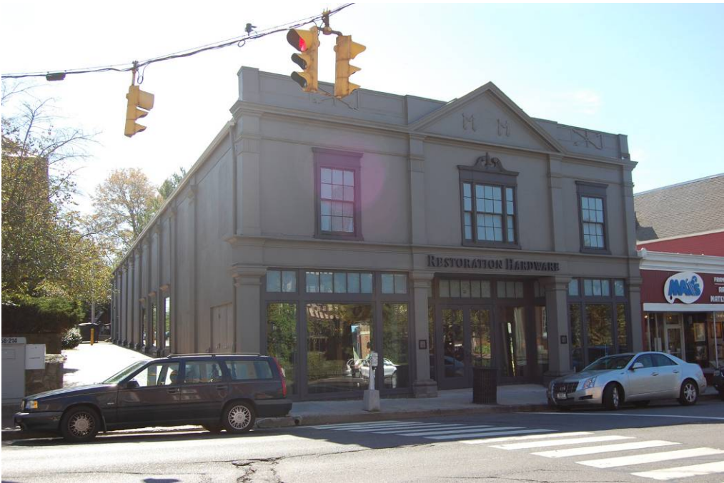
View of the north and east elevations.
