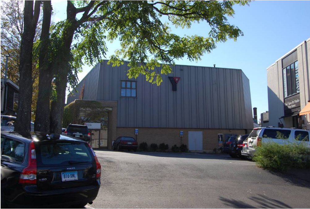
View of the north elevation.
