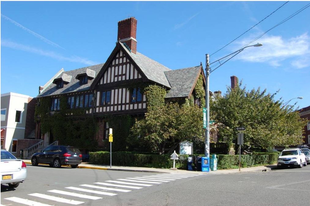
View of the west elevation.
