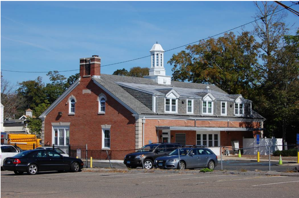
View of the south and west elevations.
