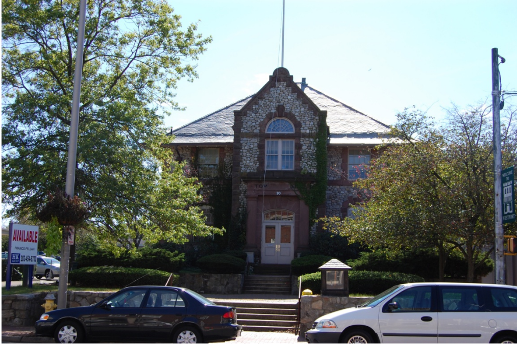
View of the north elevation.
