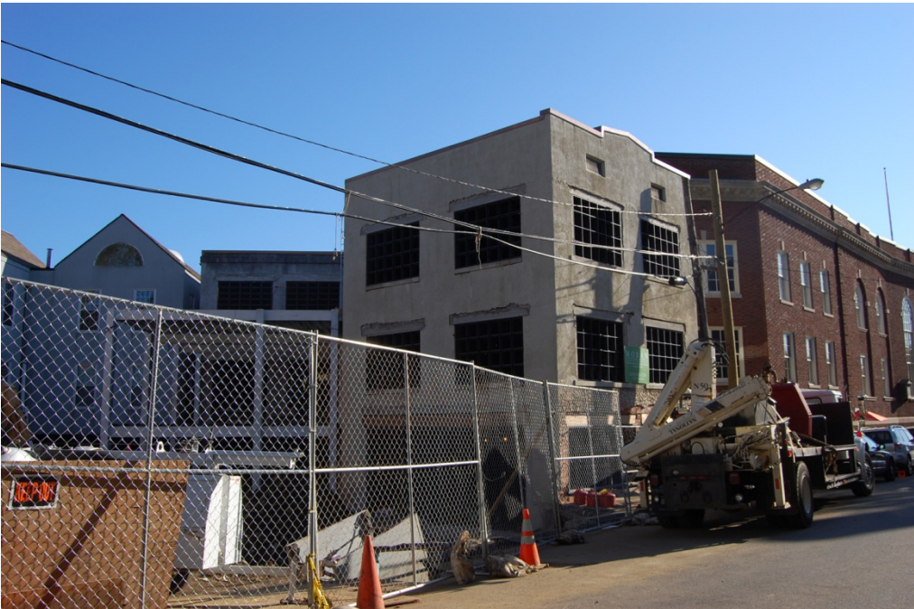
View of the northwest and northeast elevations.
