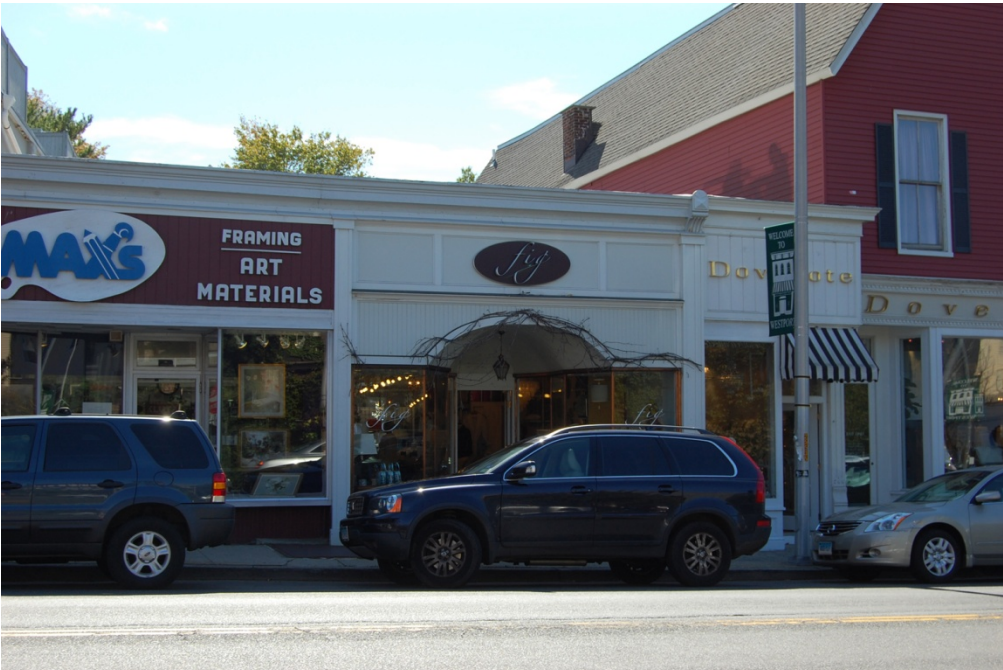
View of the north elevation.
