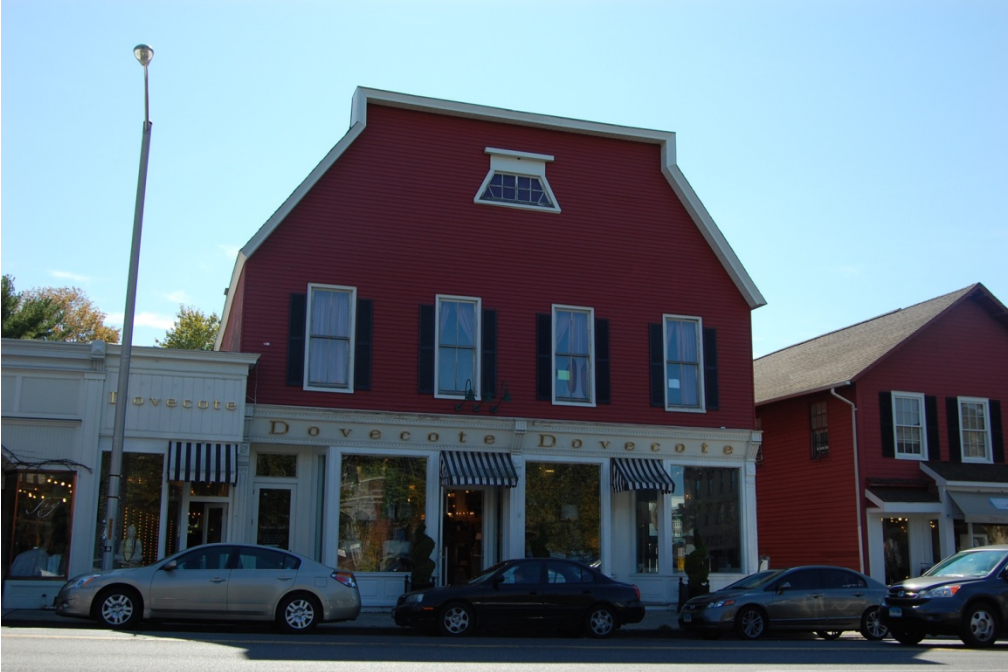
View of the north elevation.
