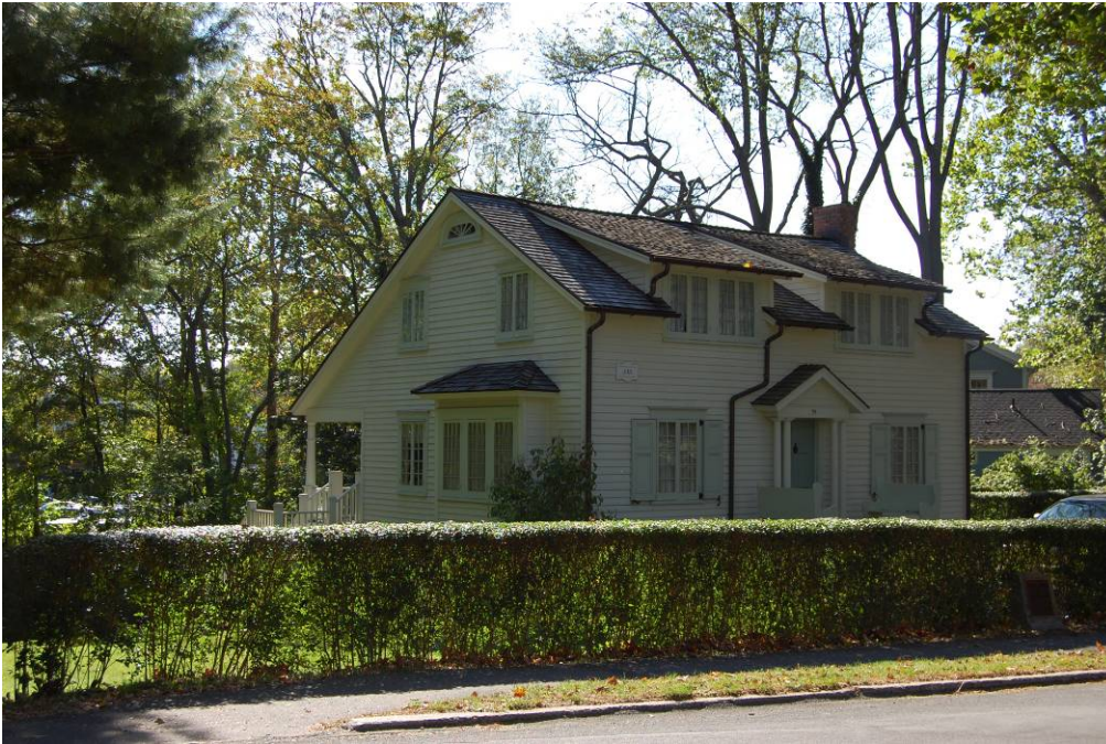
View of the north and east elevations.
