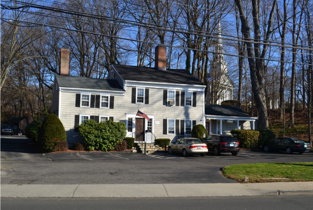
View of the west elevation.
