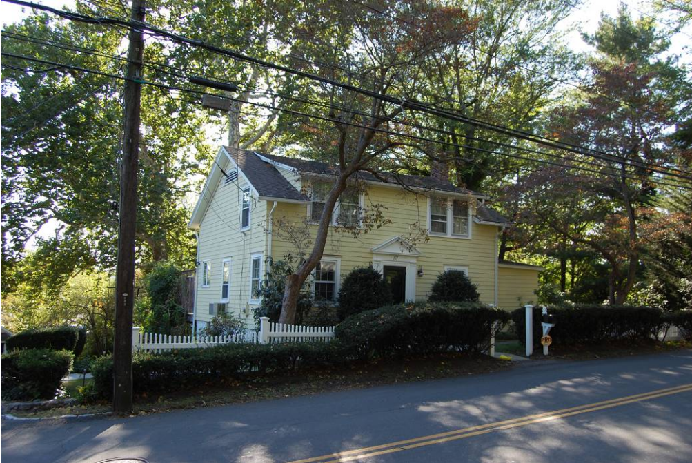
View of the north and east elevations
