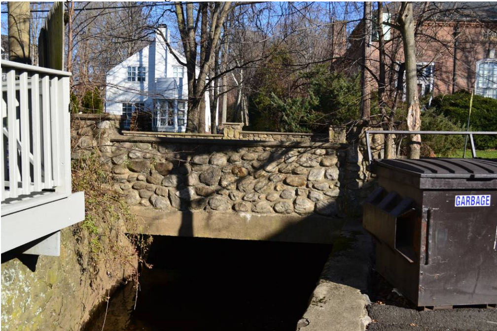
View of bridge's west face.
