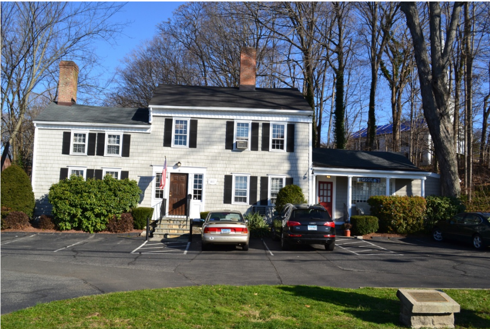
View of the west elevation.
