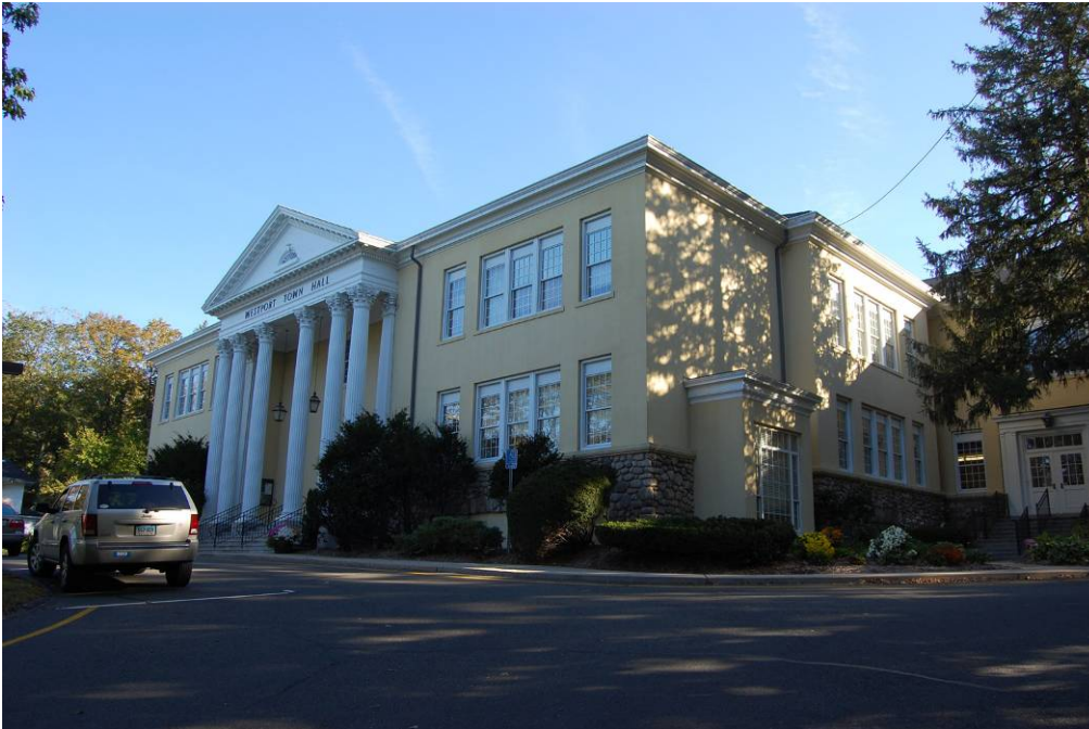
View of the west and south elevations.
