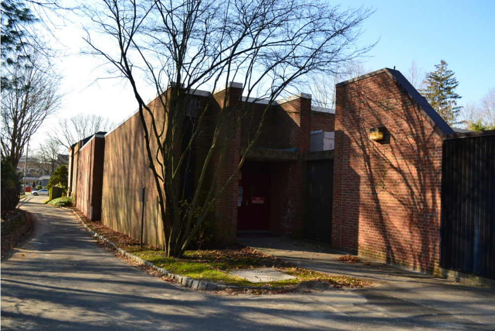
View of the south and east elevations.
