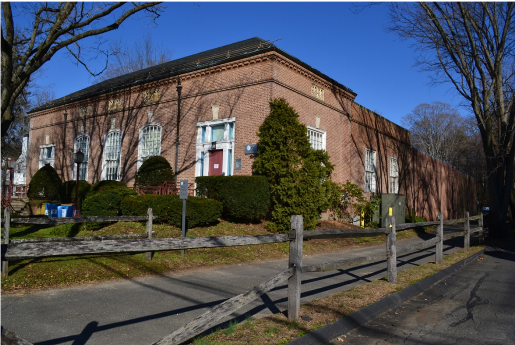
View of the west and south elevations.
