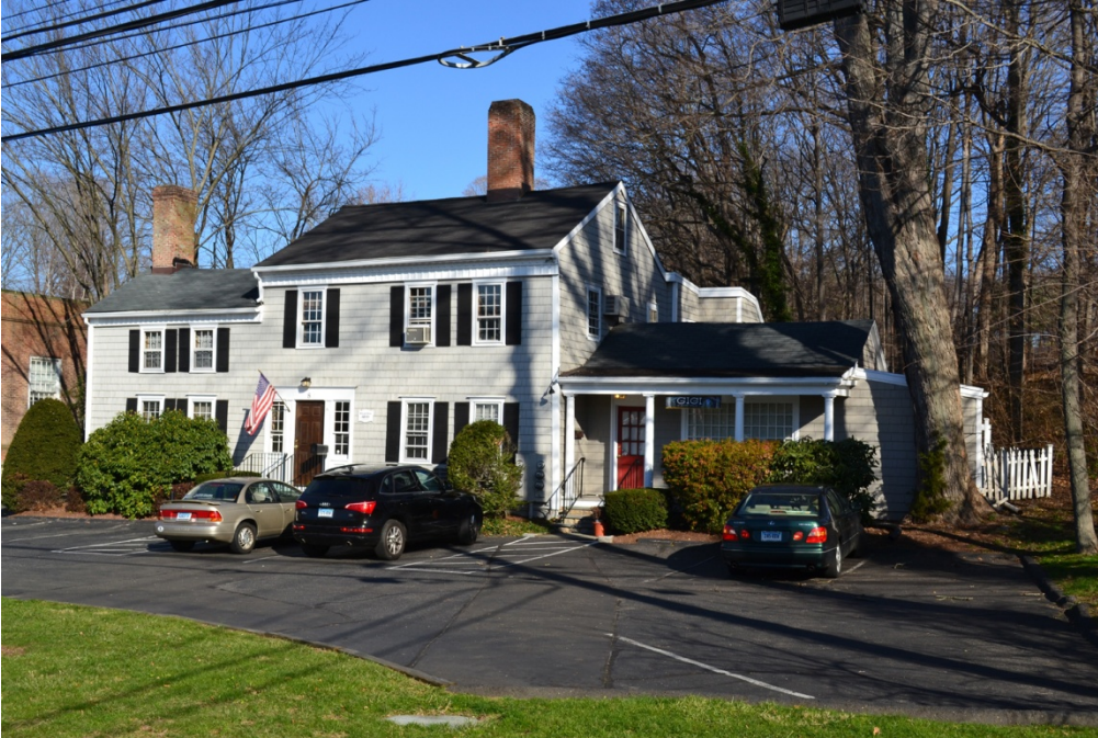
View of the south and west elevations.
