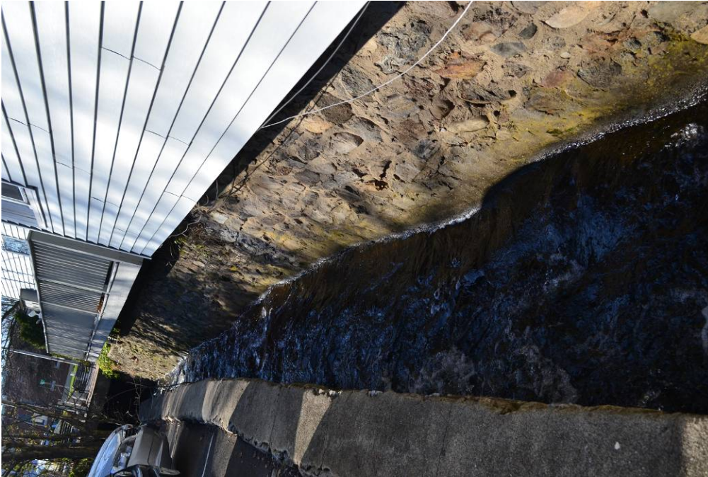
View of the channel looking west.
