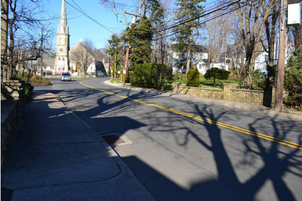
View looking north across bridge.
