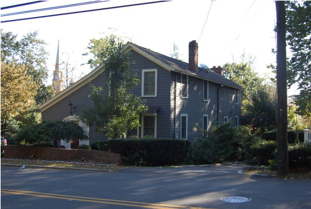
View of the north and west elevations.
