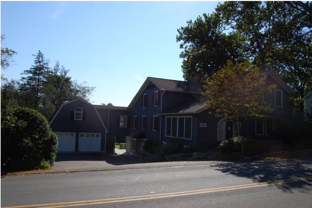
View of the north and east elevations.
