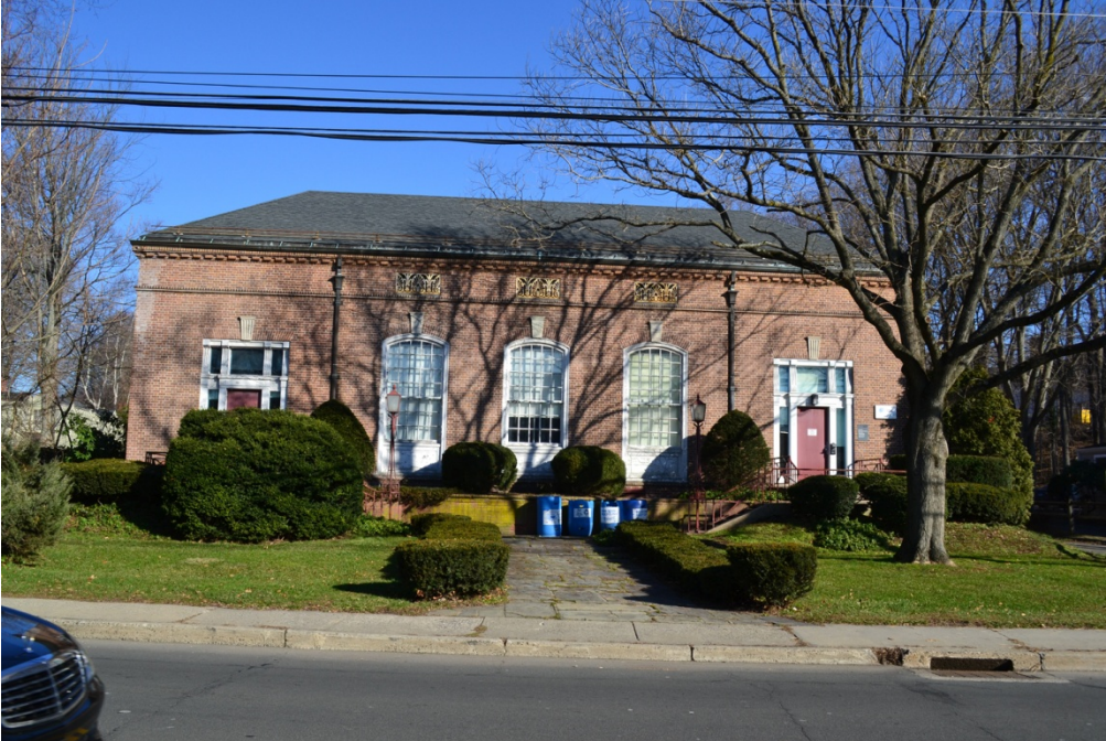
View of the west elevation.
