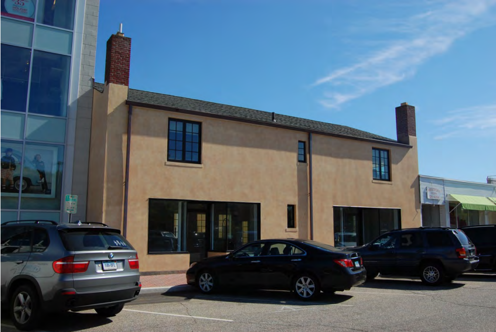
View of the west elevations of the rear building.
