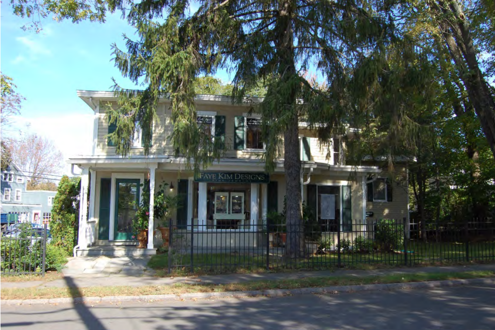
View of the south elevation of the main building.
