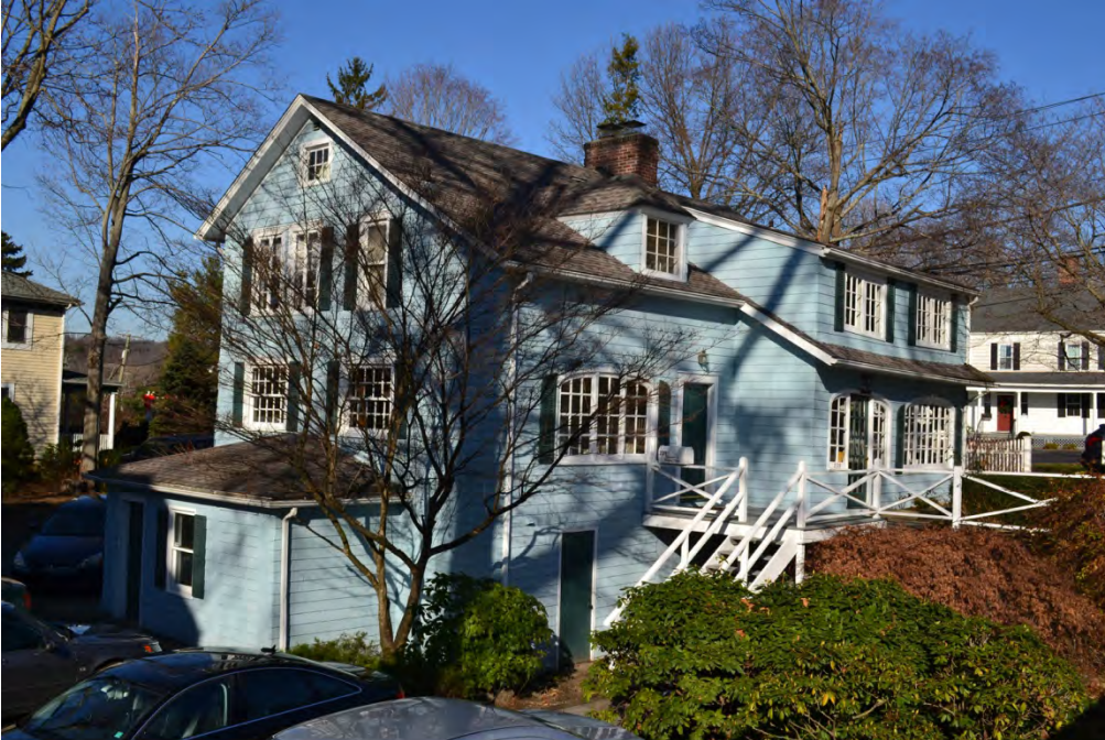
View of the south and west elevations.
