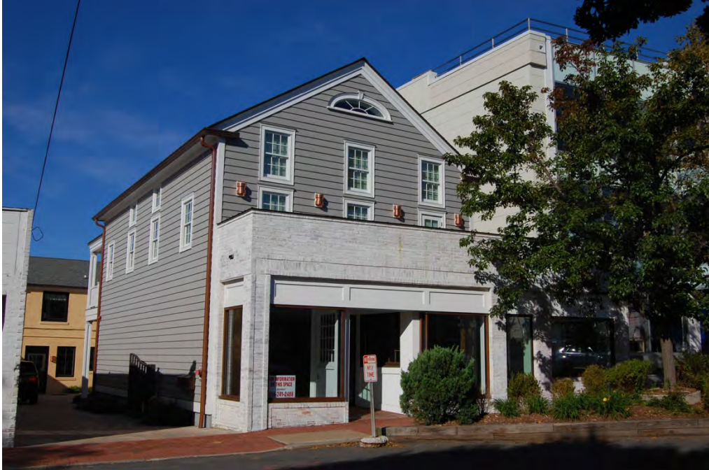
View of the east and south elevations.
