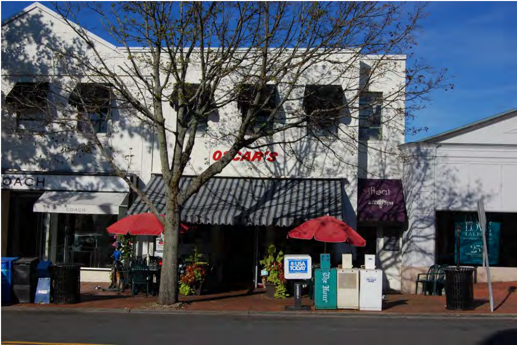
View of the east elevation.
