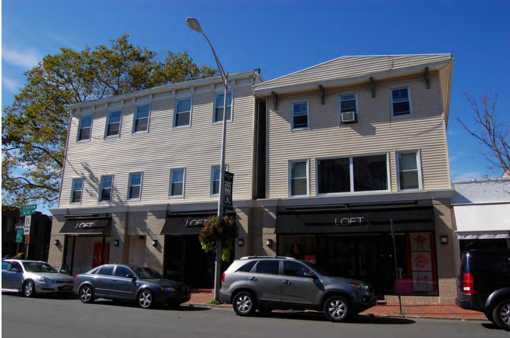
View of the east elevations.
