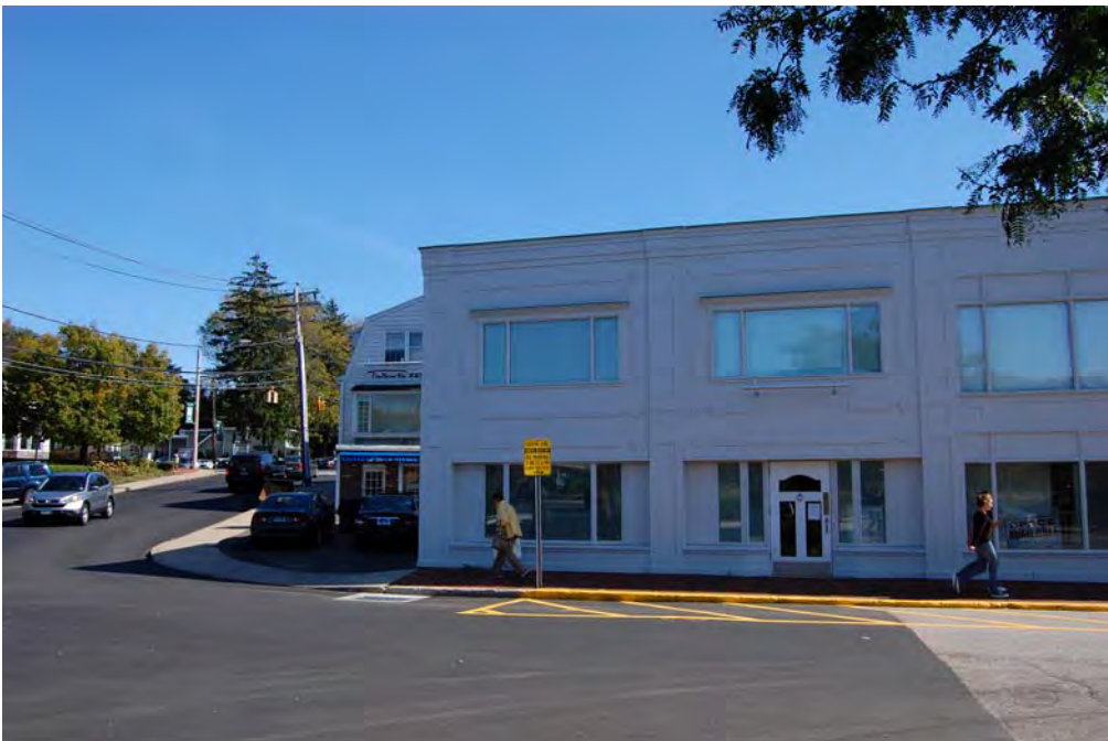
View of west elevation.
