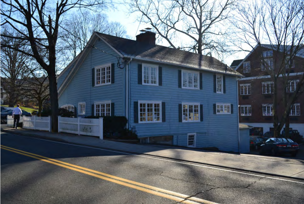
View of the north and east elevations.
