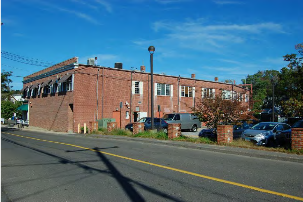
View of the east elevation.
