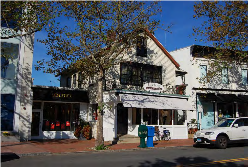
View of the east elevation.
