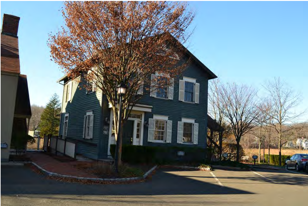
View of the east and south elevation.
