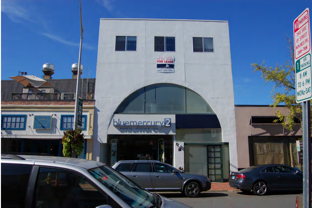
View of the east elevation.
