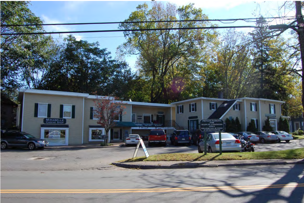
View of the west elevation of the main building and second building.
