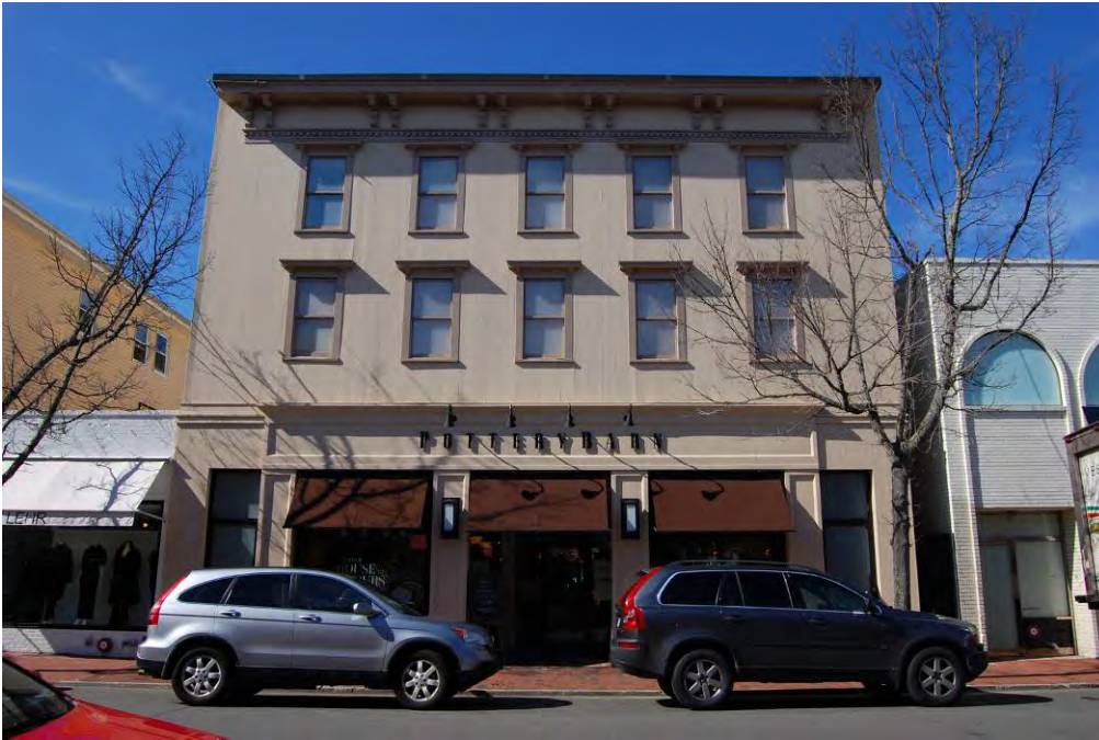
View of the east elevation.
