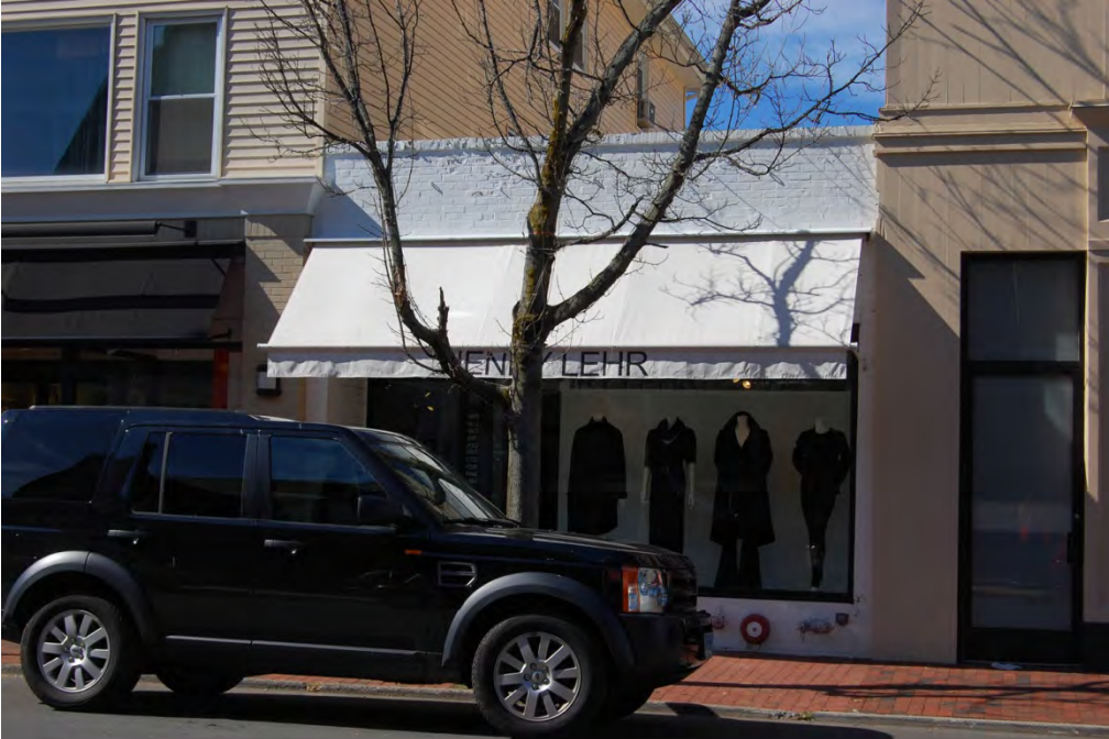
View of the east elevation.
