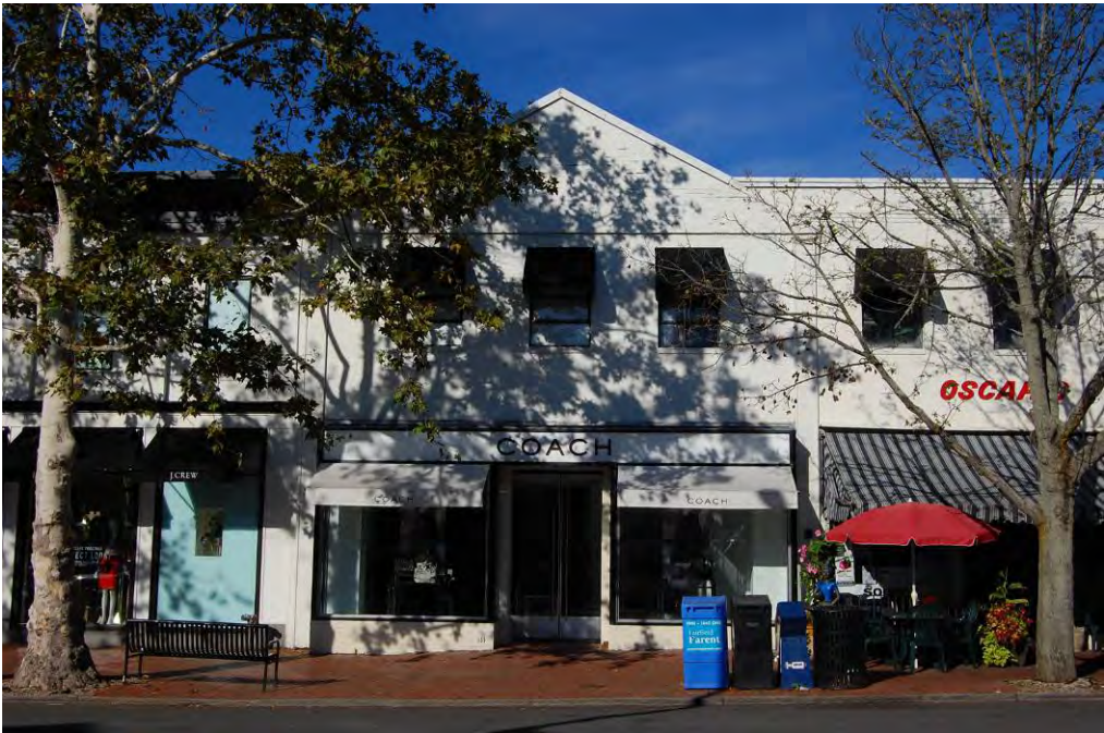
View of the east elevation.
