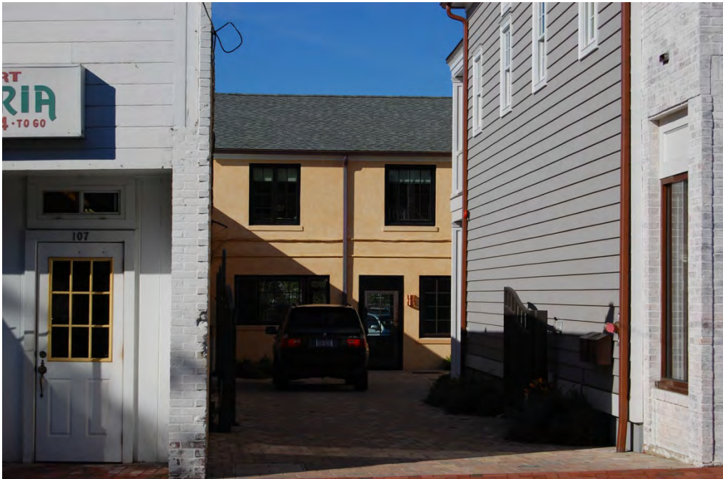
View of the south elevation and the east elevation of the rear building.
