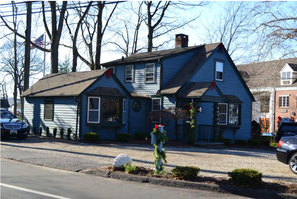
View of the north and west elevations.
