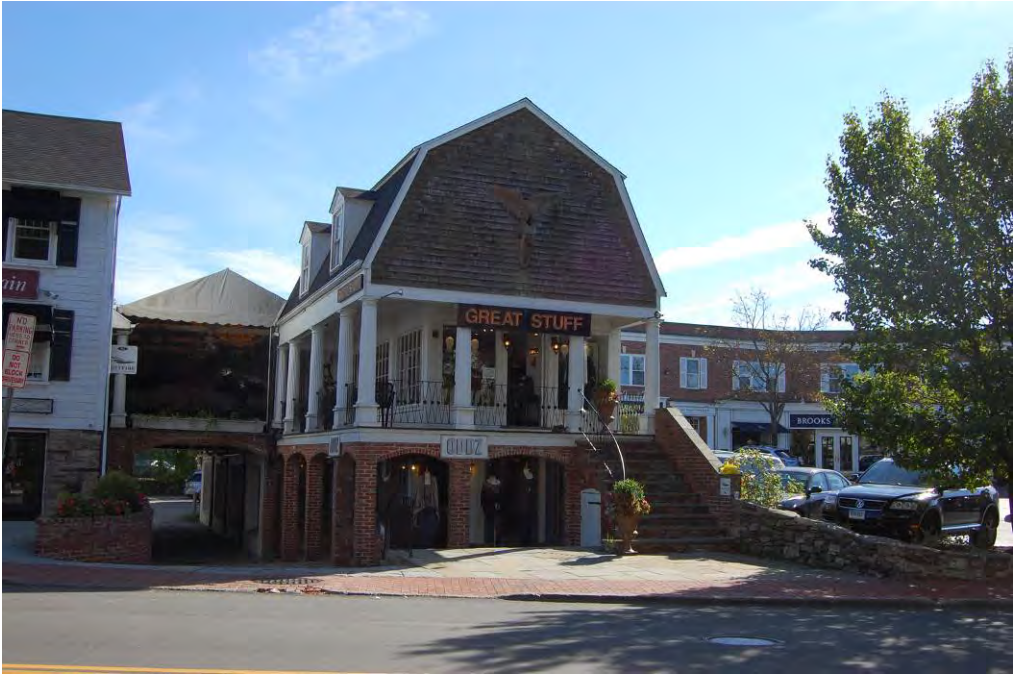
View of the west and north elevations of the addition at 146 Main Street.
