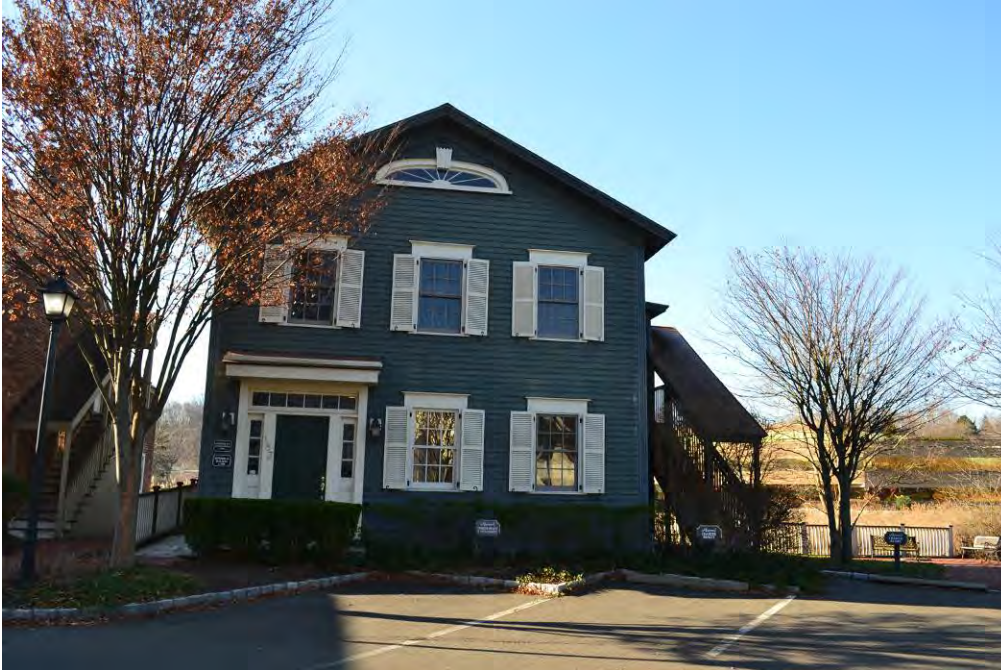
View of the east elevation.
