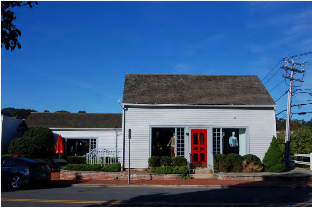
View of the east elevation.
