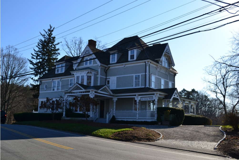
View of the northeast and northwest elevations.
