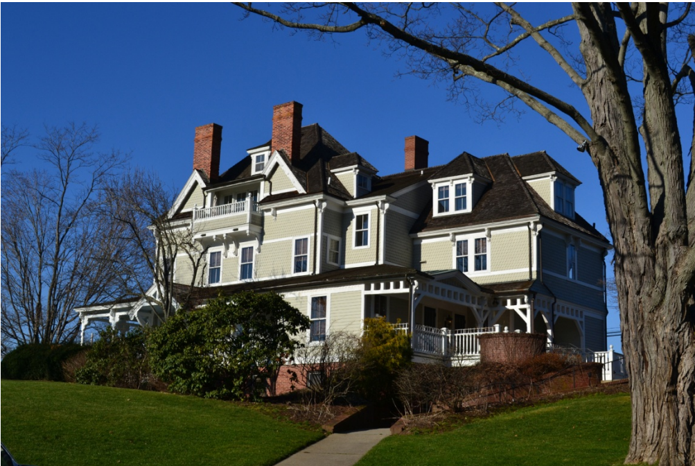
View of southwest and southeast elevations.
