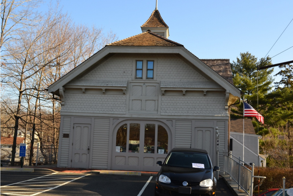
View of the west elevation.
