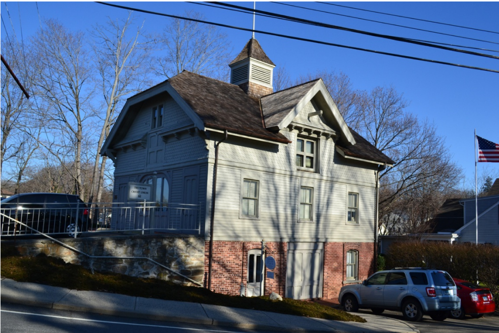
View of the south and west elevations.
