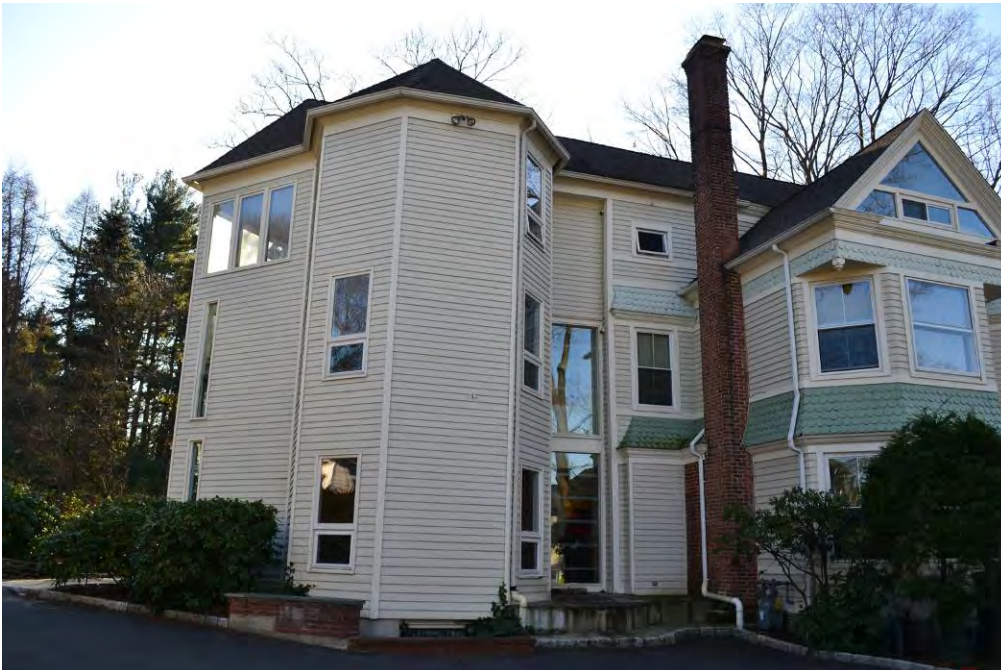
View of the west elevation.
