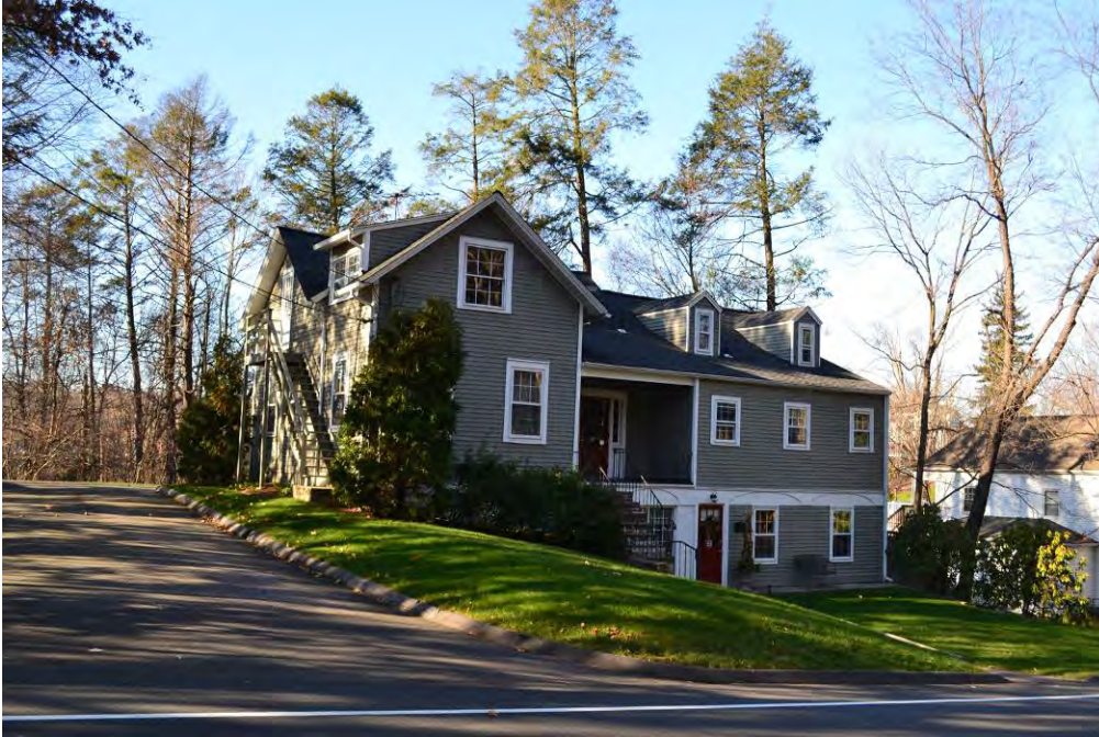
View of the east and south elevations.
