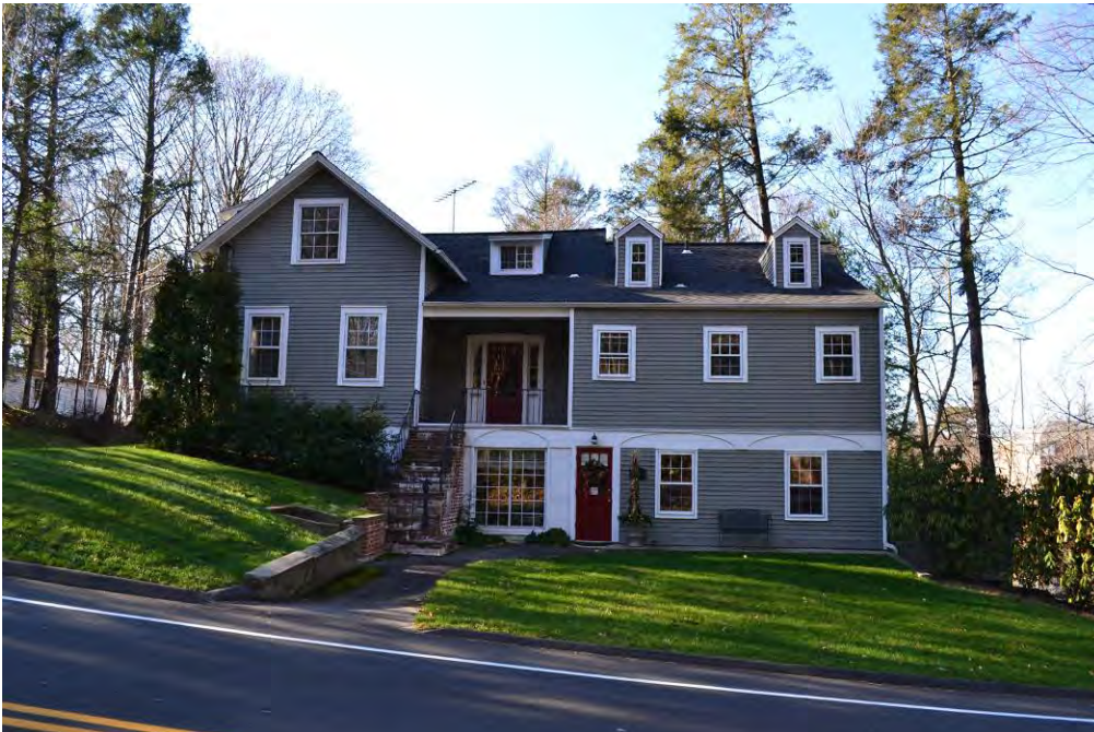
View of the east elevation.
