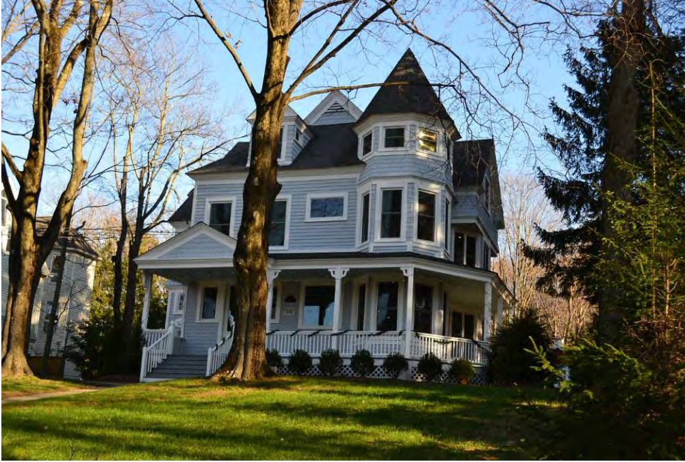
View of the west and south elevations.
