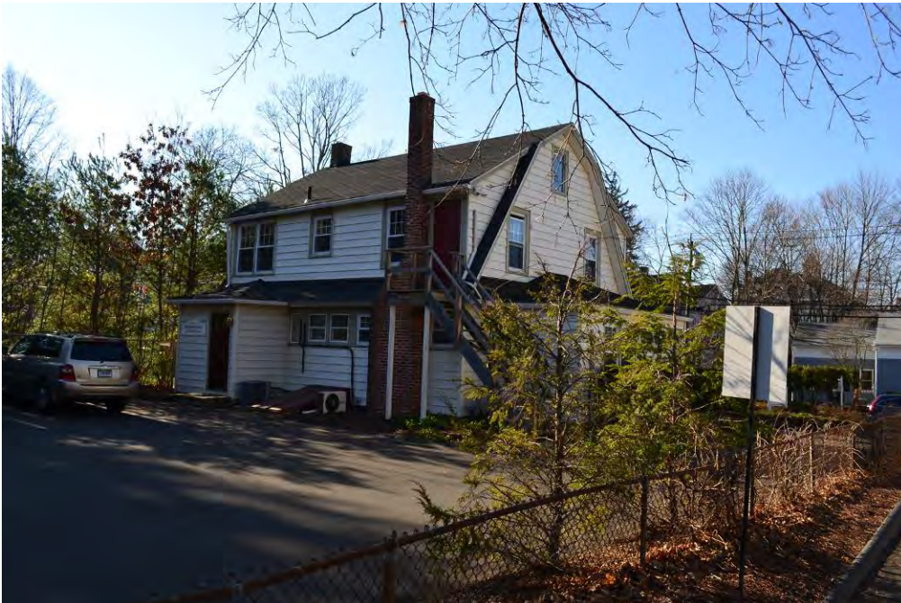
View of the south and east elevations.
