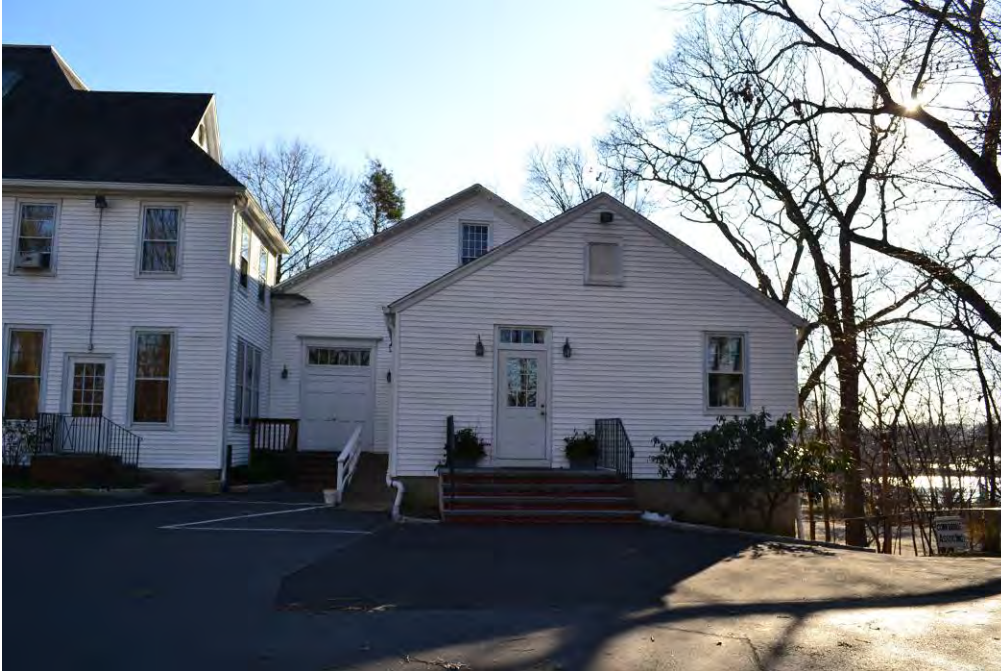
View of the north elevation.
