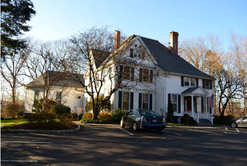
View of the east and south elevations.
