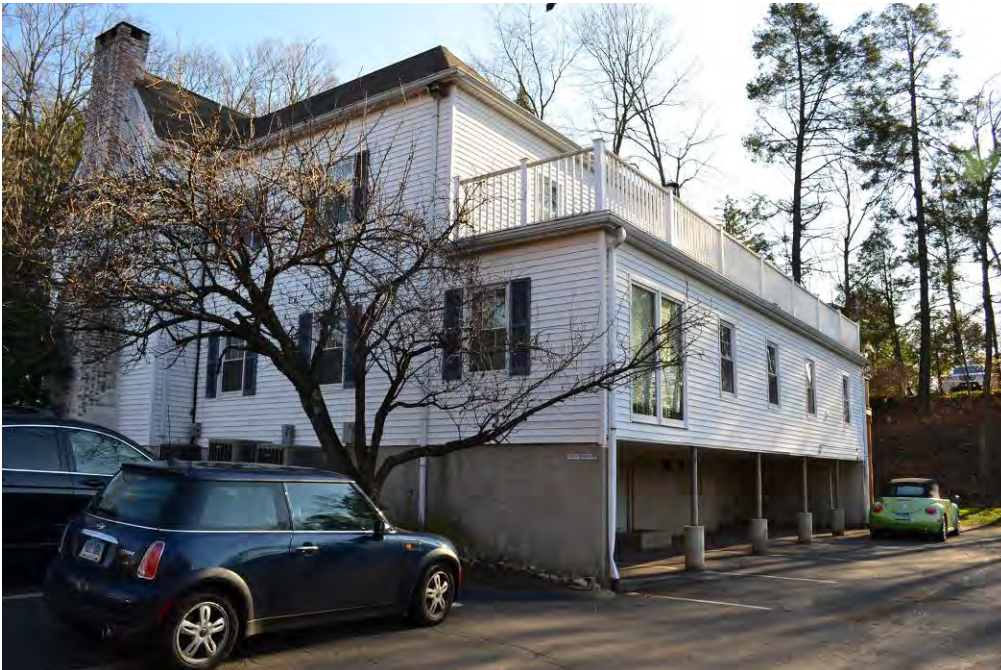
View of the north and west elevations.
