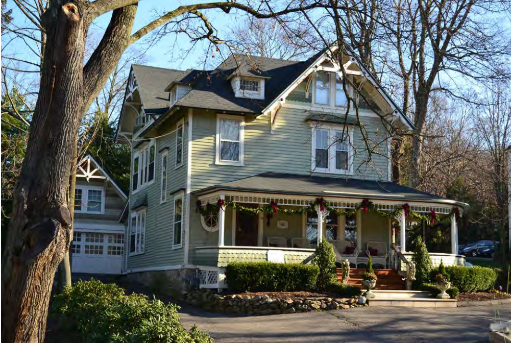
View of the west and north elevations.
