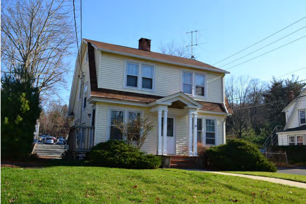
View of the west and north elevations.
