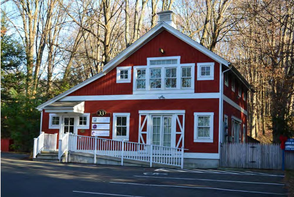
View of the west and south elevations of the converted barn.
