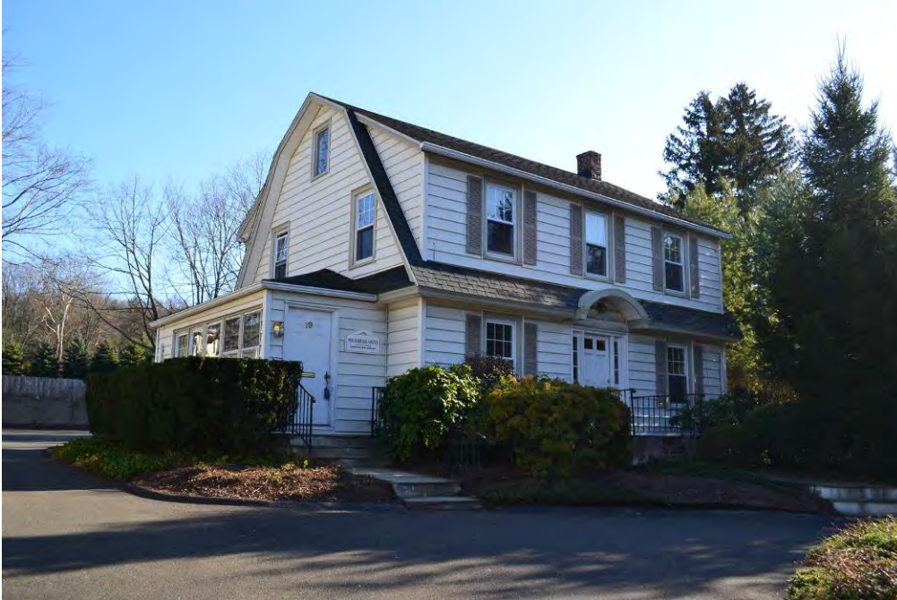
View of the north and west elevations.
