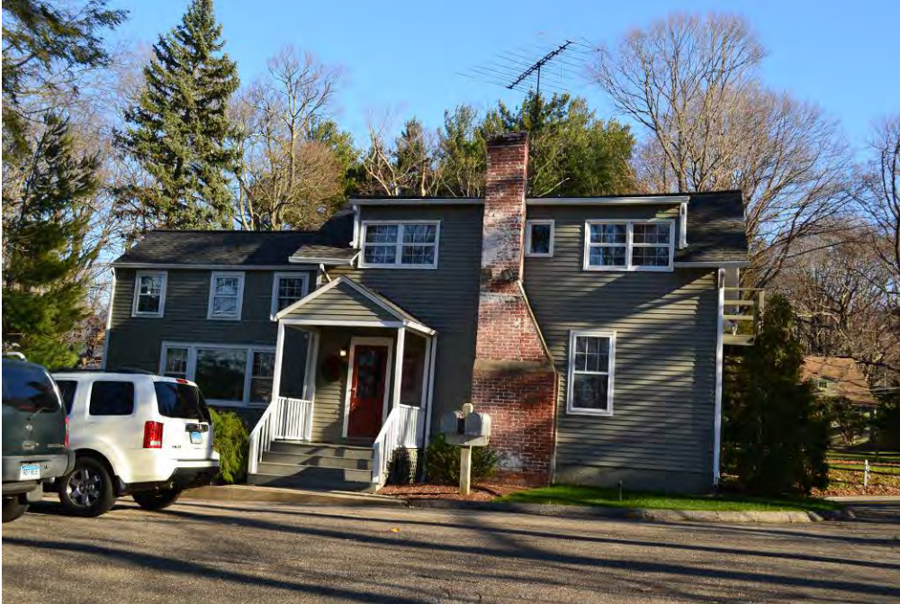
View of the west elevation.
