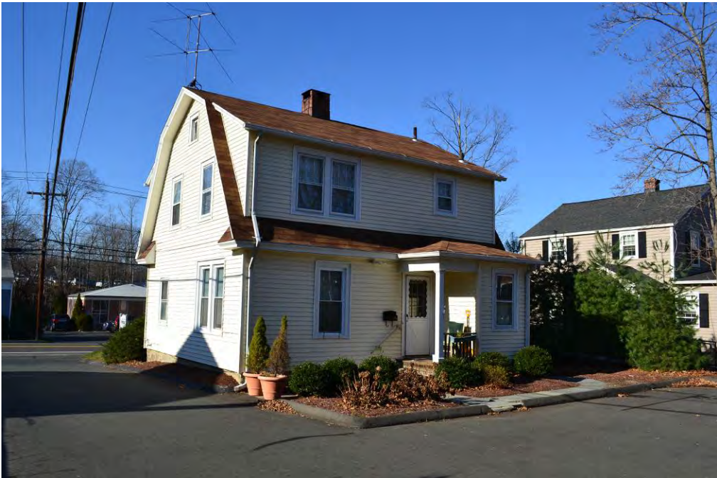
View of the east and south elevations.
