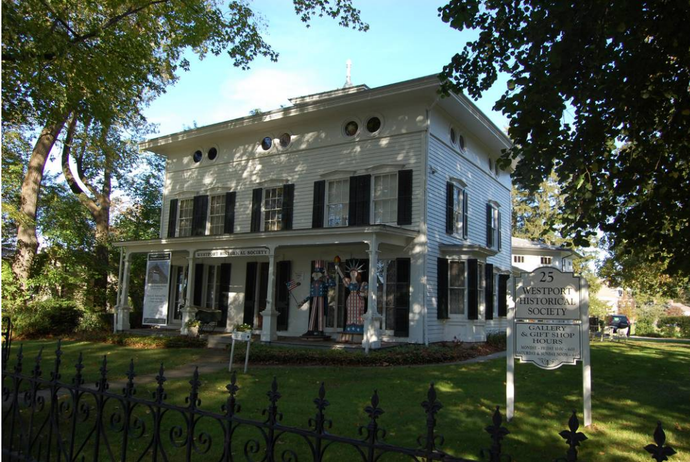
View of the south and east elevations.
