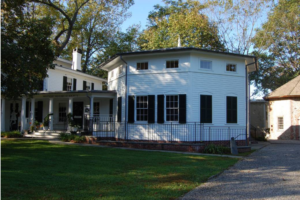
View of the east elevation.
