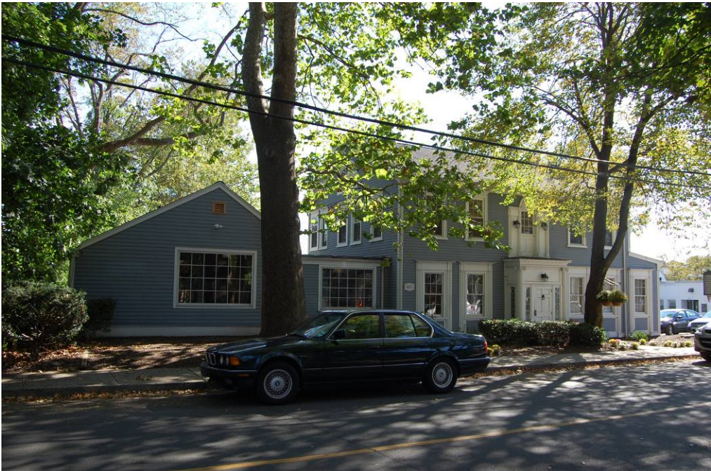
View of the north and east elevations.
