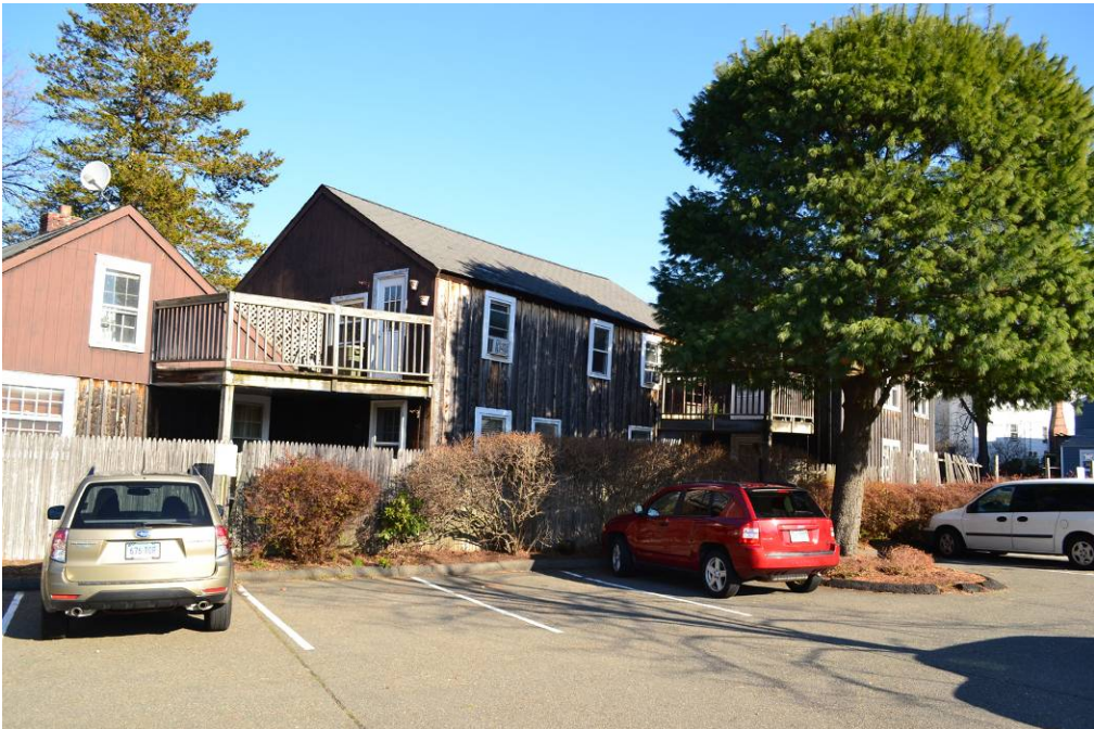
View of the south and west elevations.
