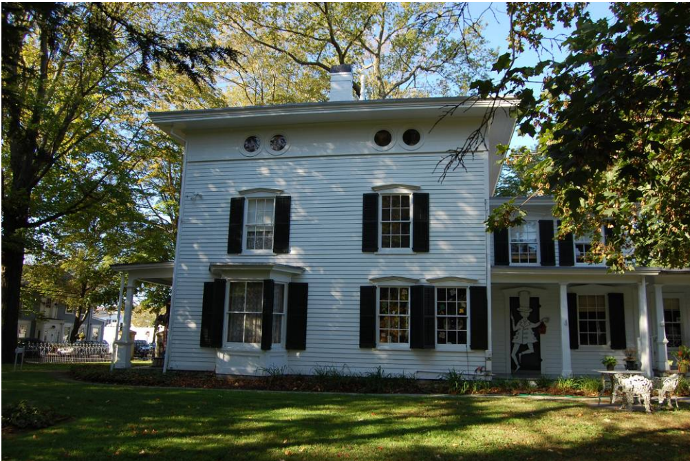
View of the east elevation.
