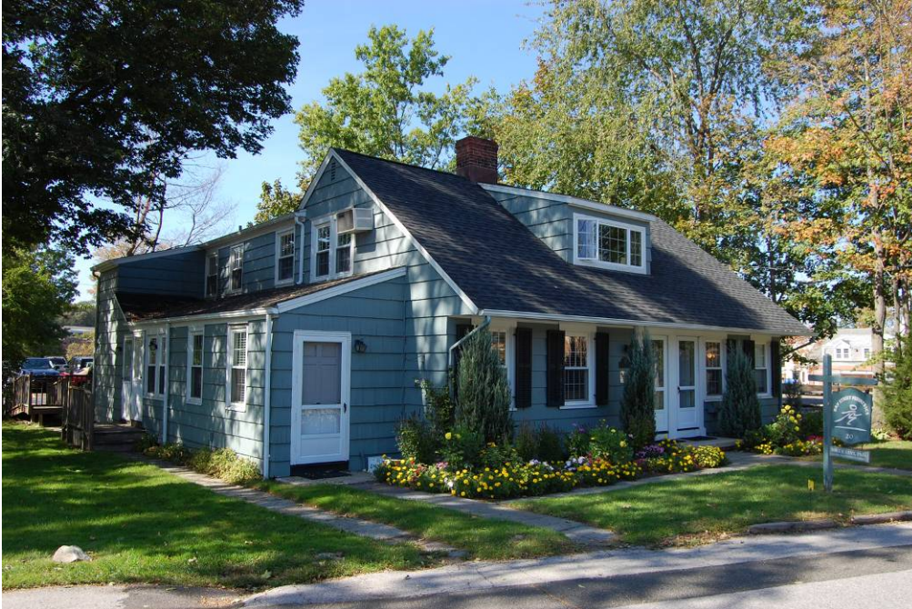
View of the east and south elevations.
