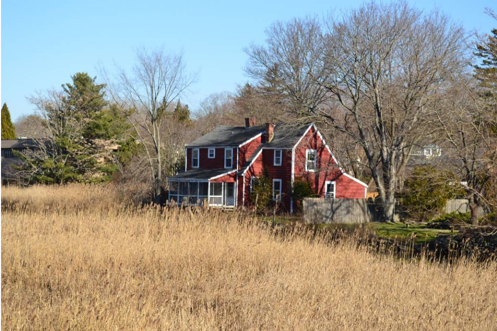
View of the south and west elevations
