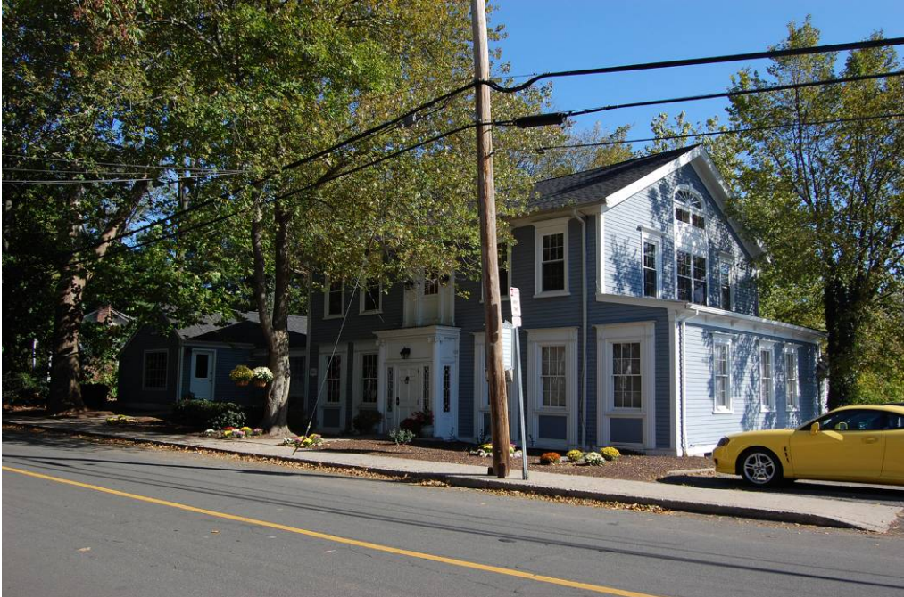
View of the north and west elevations.
