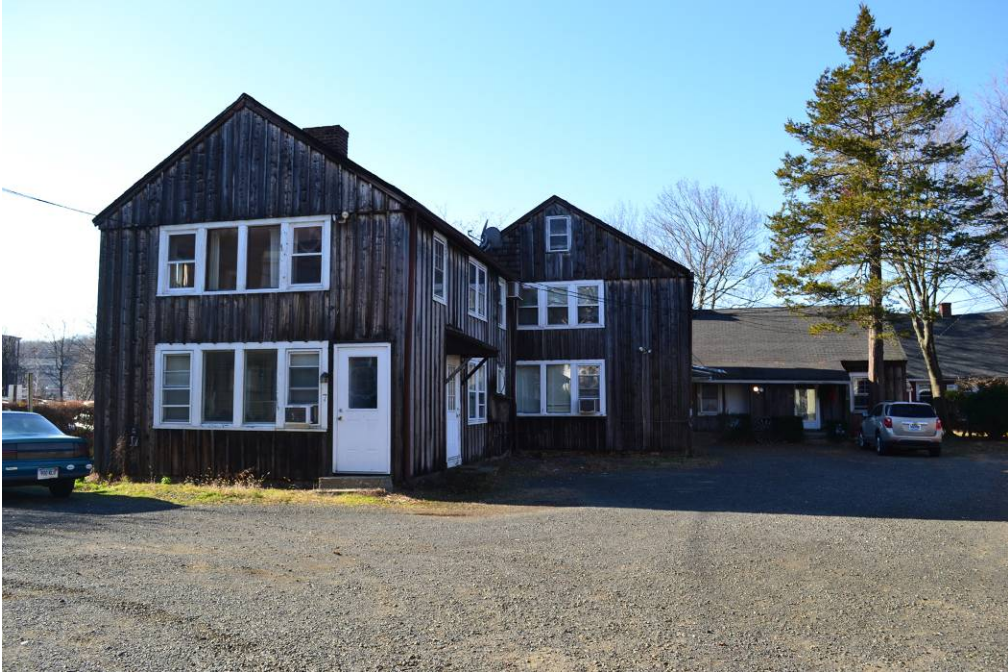
View of the north and east elevations.
