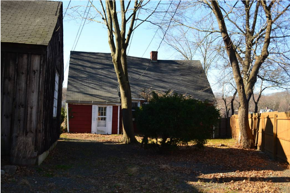
View of the east elevation.
