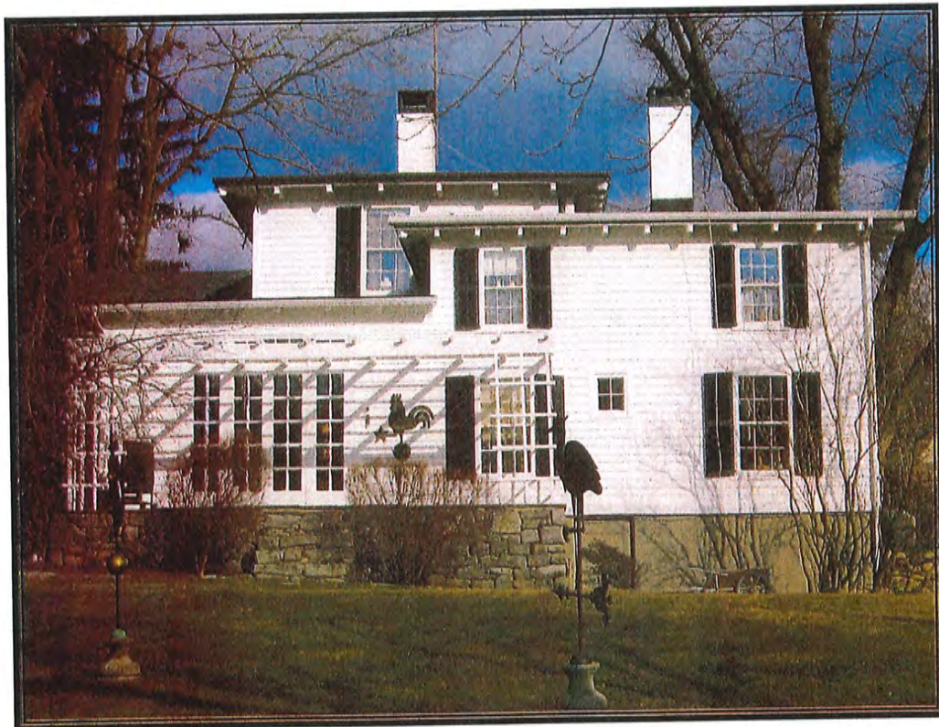
Figure 7. Main House, west elevation—View to East
