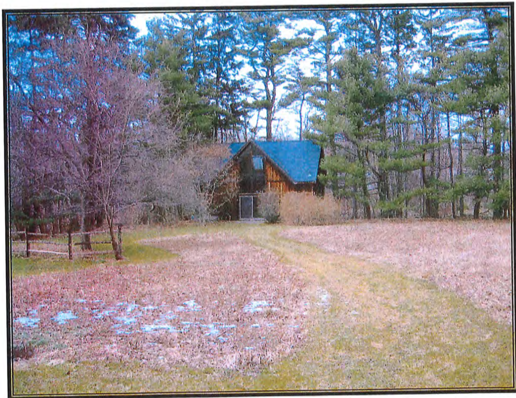
Figure 13. North Lawn & Studio— View to Northwest
