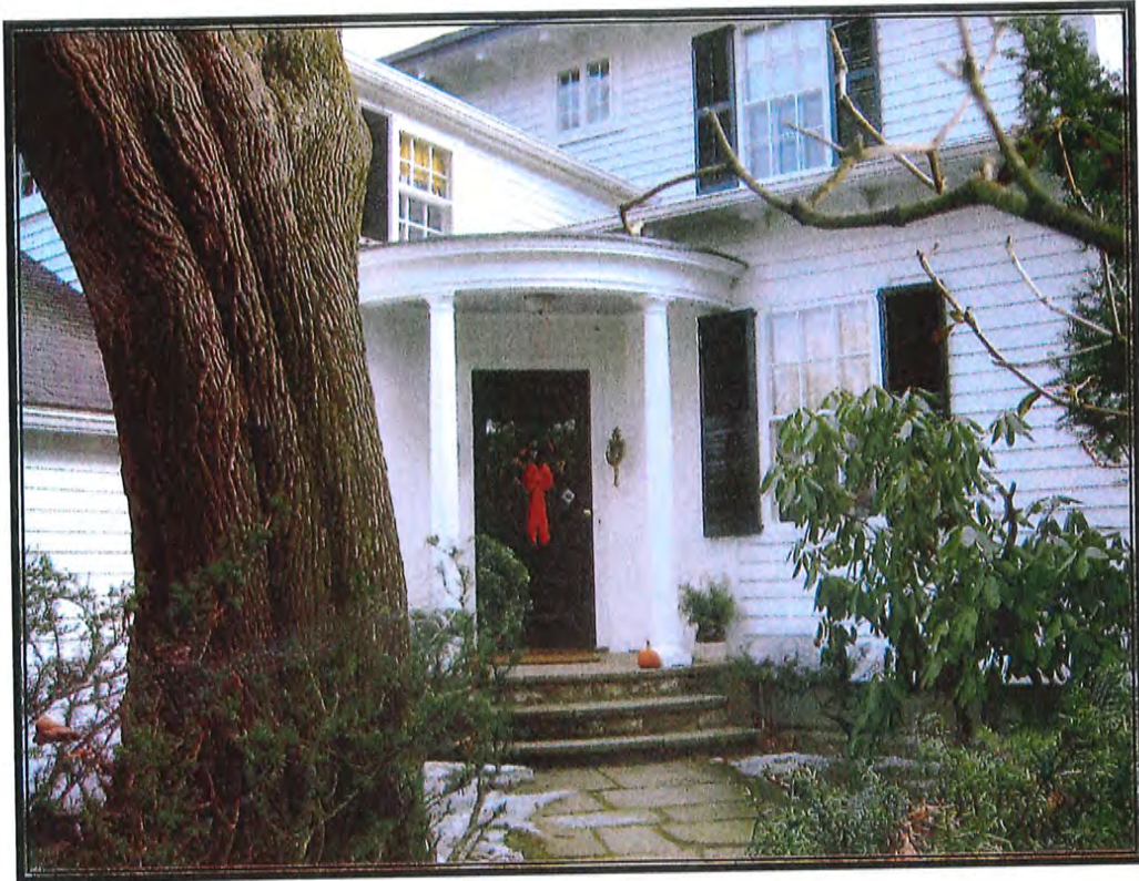
Figure 8. Main Entrance—View to Southeast
