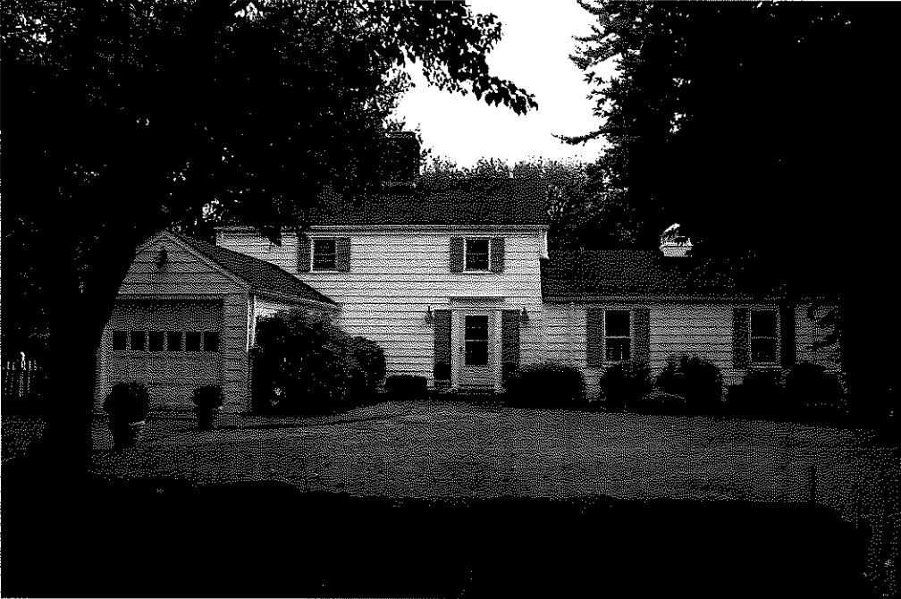
View of the west elevation.
