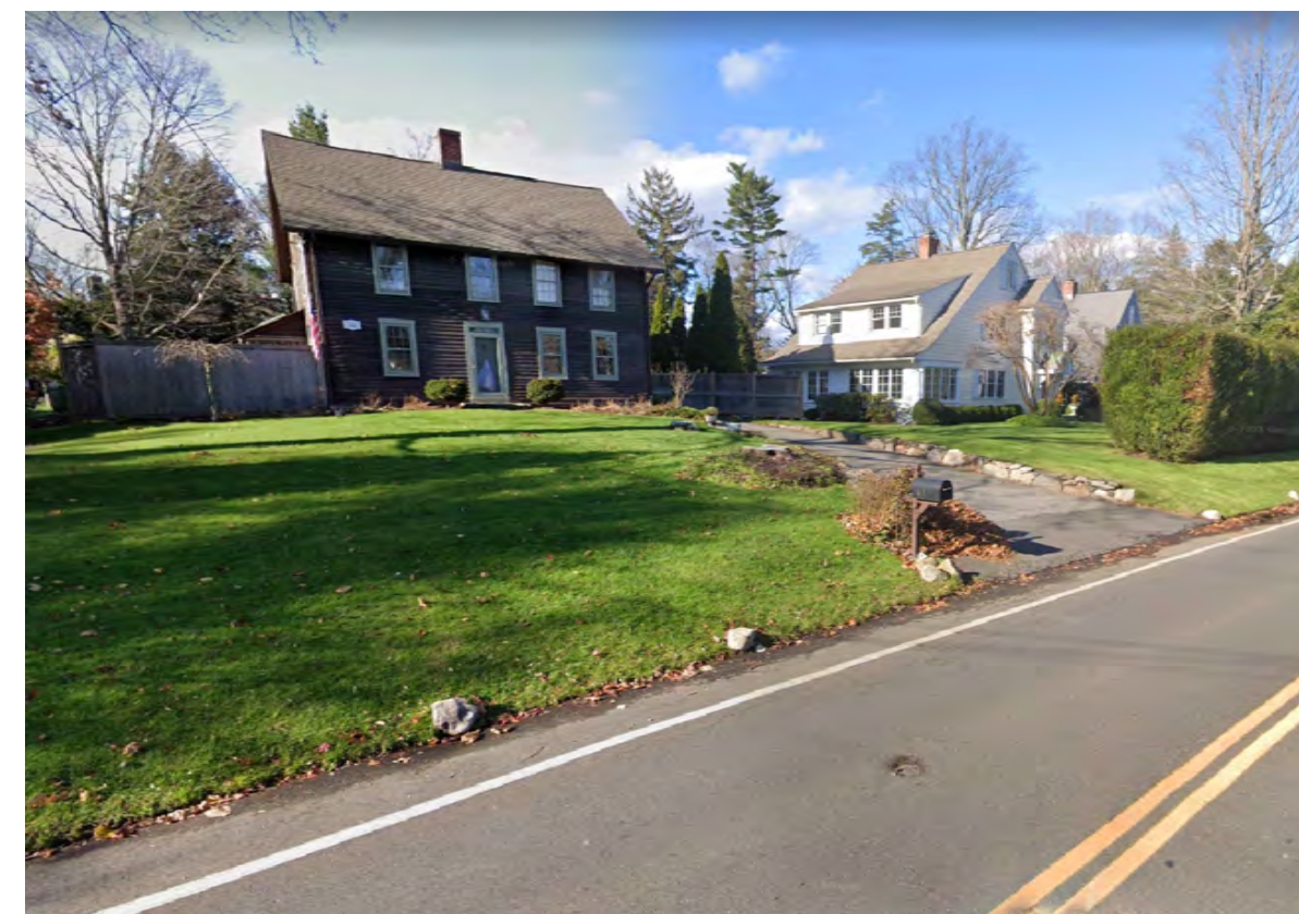
C-67/69 KINGS HIGHWAY
