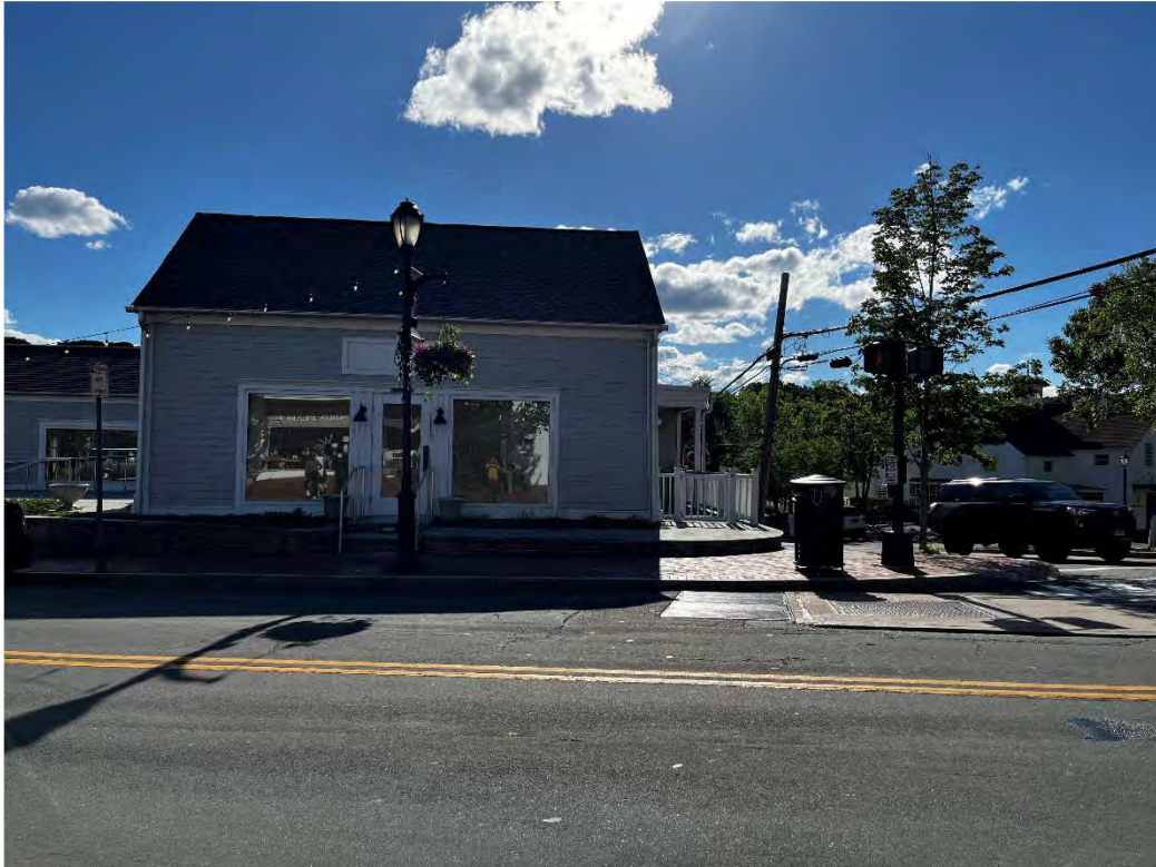
Original Building and Corner – Existing
