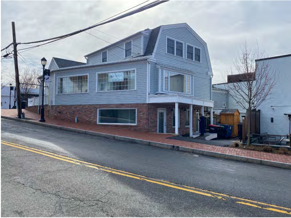
Rear of Building – Existing
