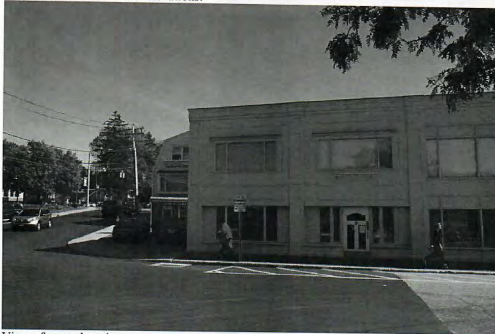
View of west elevation.
