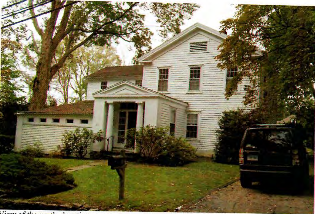
View of the north elevation.
