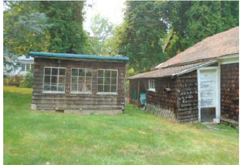
SHED FRONT (EAST)
