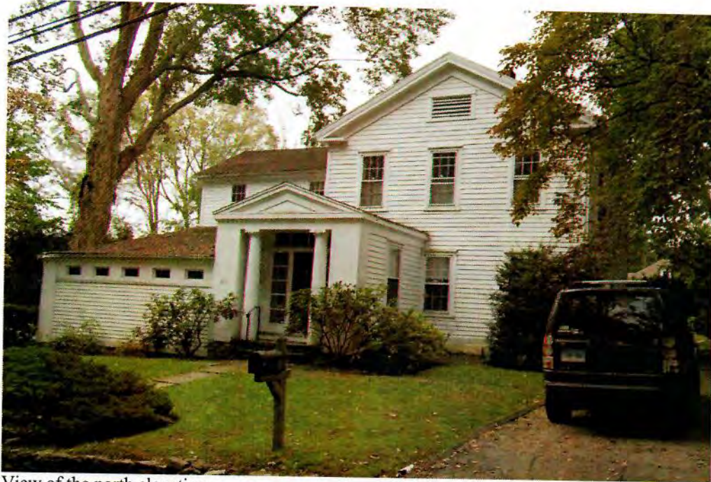
View of the north elevation.
