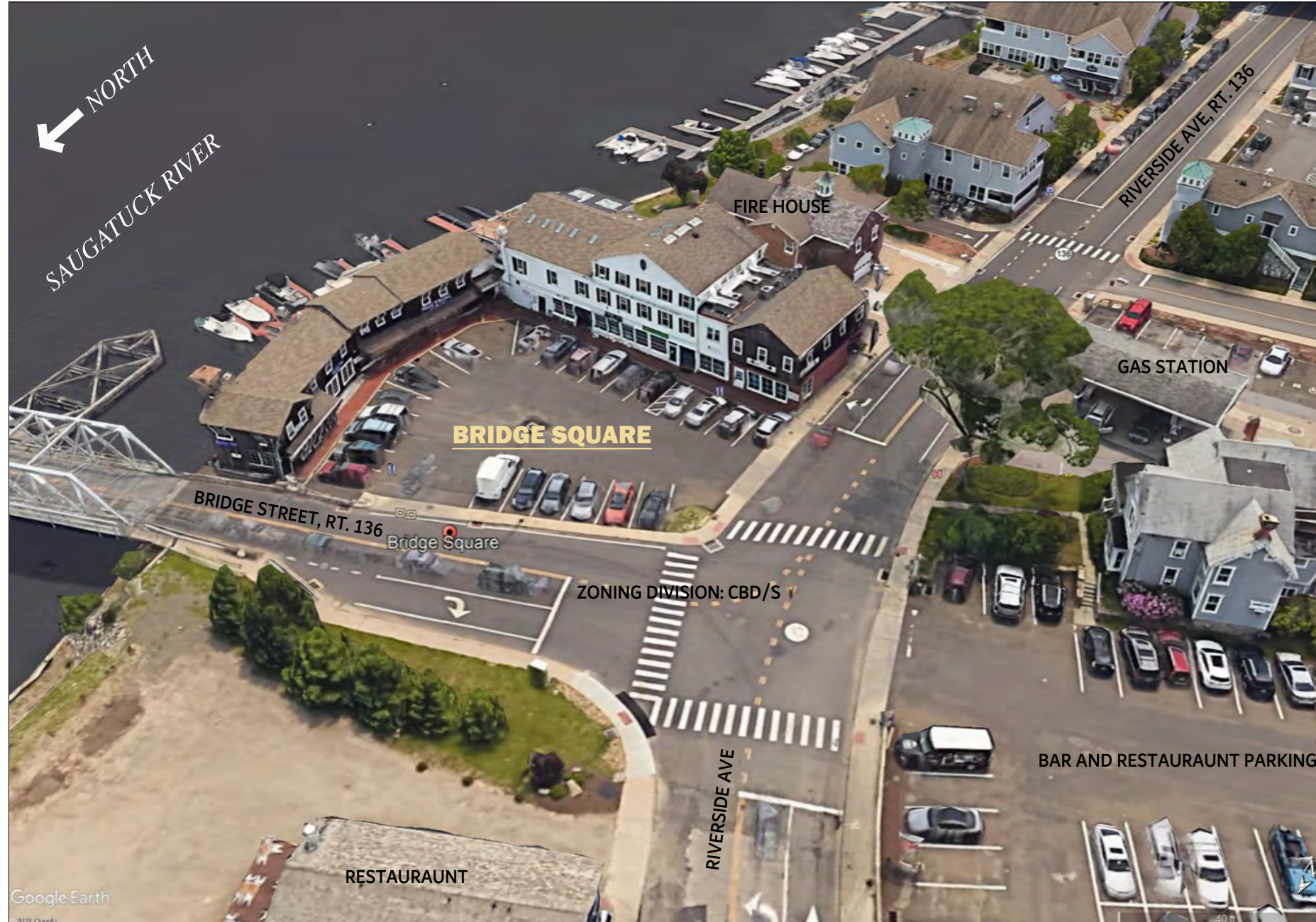
EXISTING CONDITIONS + LOCATION
