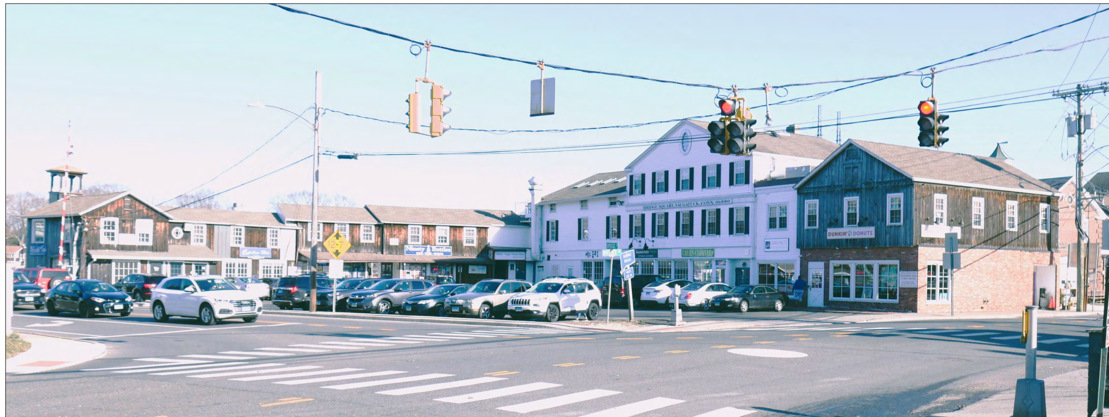
STREET VIEW EXISTING CONDITIONS
