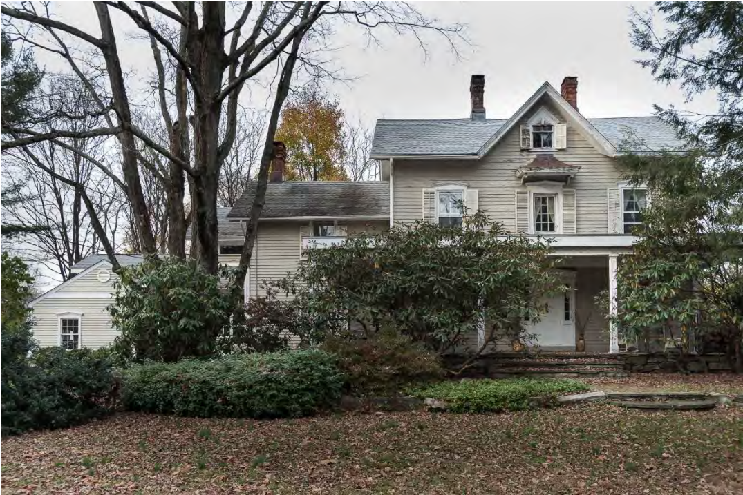
Photo 1. 39 Cross Highway view north showing façade
