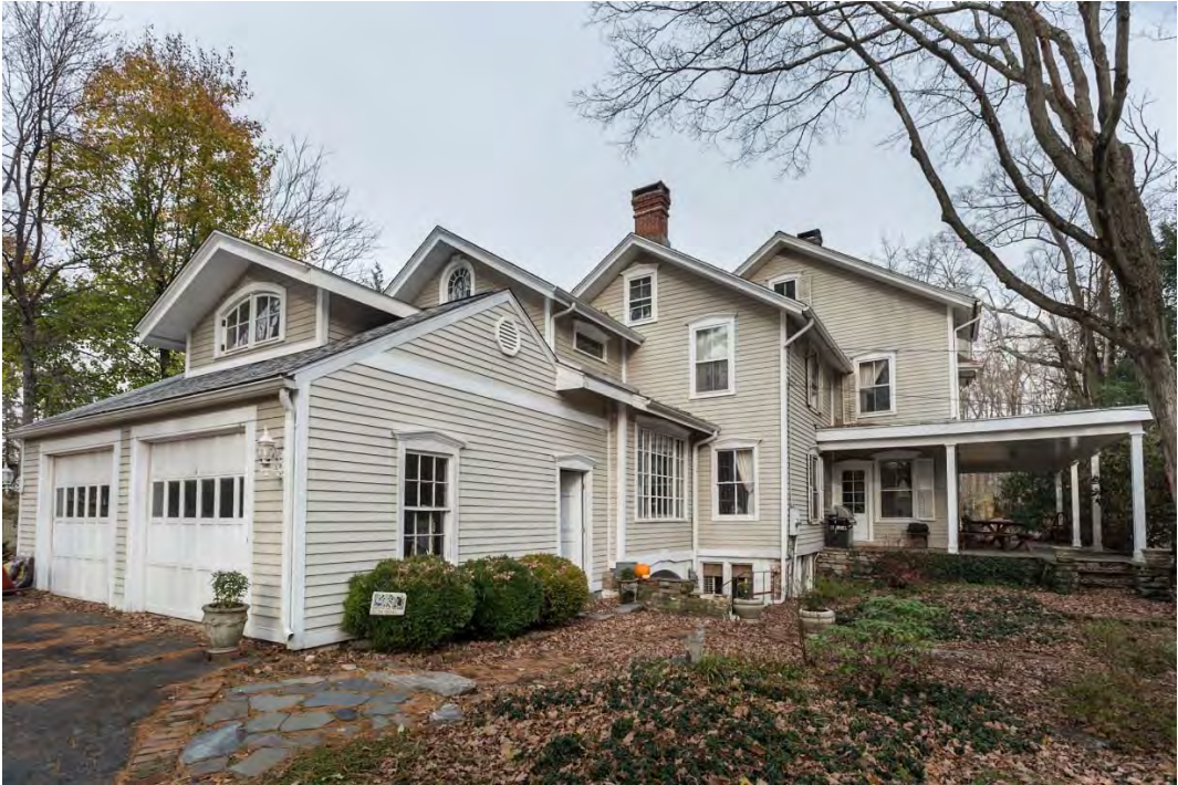
Photo 2. View northeast showing west elevation
