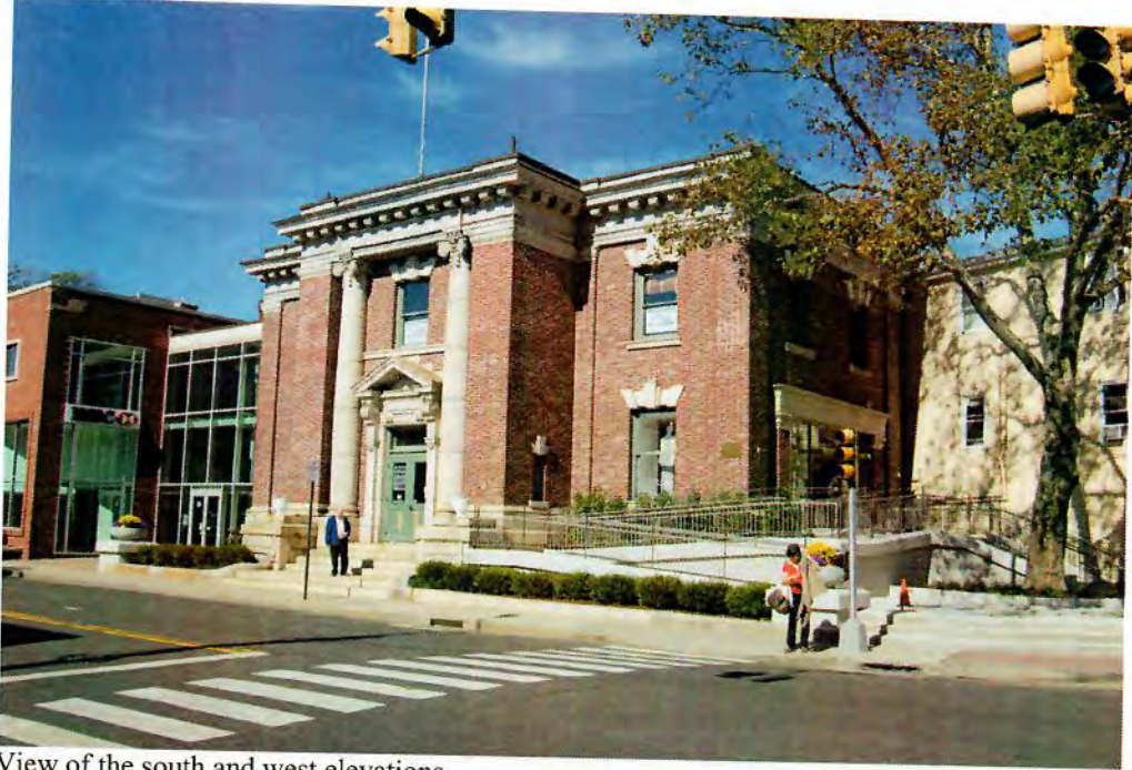
View of the south and west elevations.
