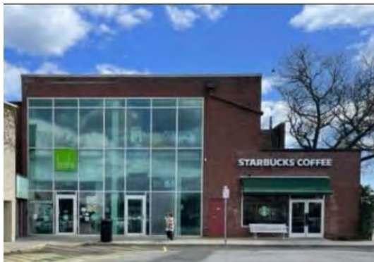
1 – Parker Harding Plaza (North)
