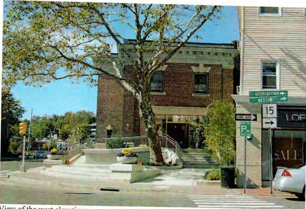
View of the west elevation.
