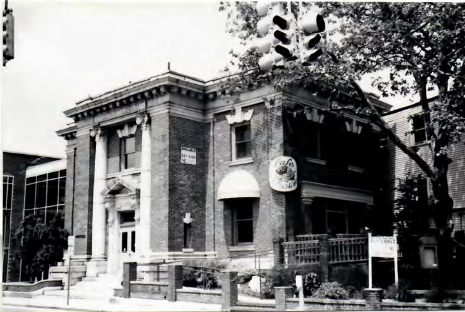
View from the southeast.
